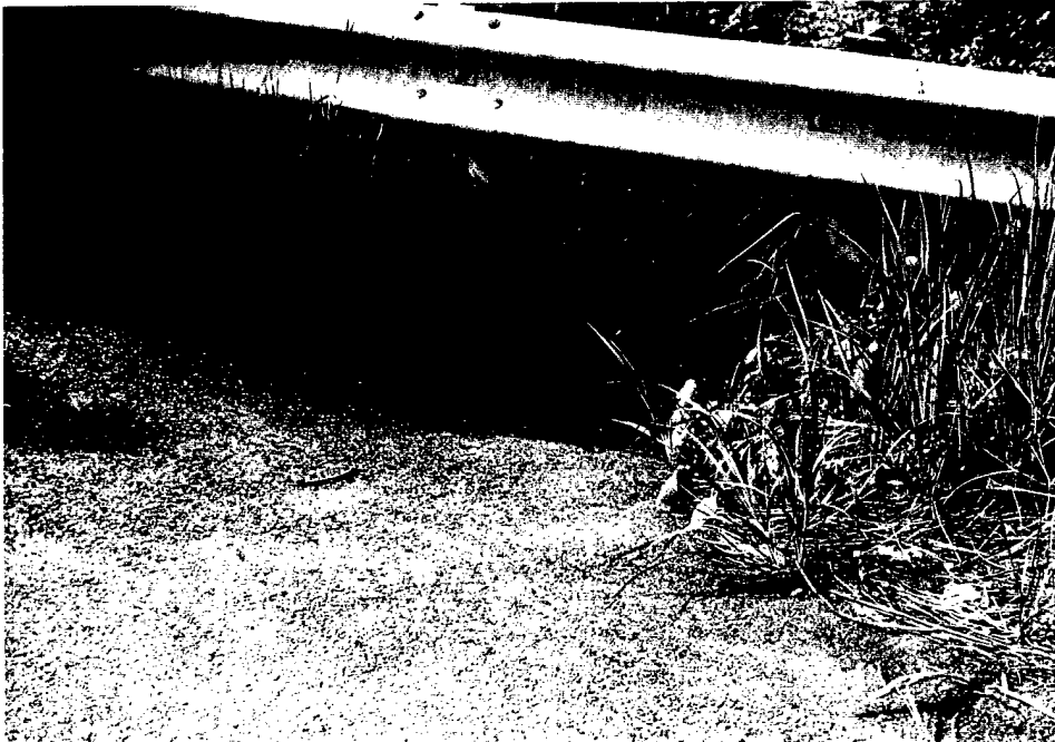
Photo 8: Paved Drainage Swale, School Street (stateline)
