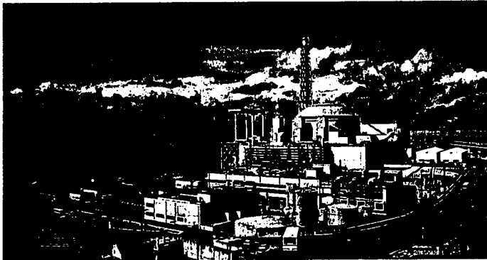
▲FBR "MONJU" under construction
