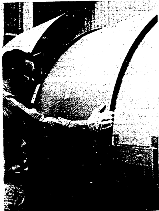
FIGURE 17. S-II TEST PANELS BEING FITTED TO AN EVALUATION TANK
