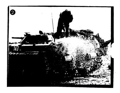
Pretreatment involves spraying down with a powerful jet of water. The dirt is washed off from top to bottom, which rinses away up to two-thirds of the chemical agent that settled on the mud-covered vehicles.
