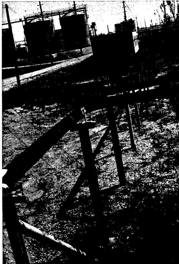
STEAM DISTRIBUTION SYSTEM SUBSTANDARD INSULATION
