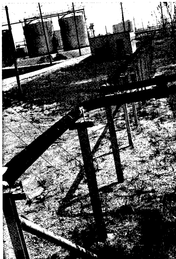
STEAM DISTRIBUTION SYSTEM SUBSTANDARD INSULATION
