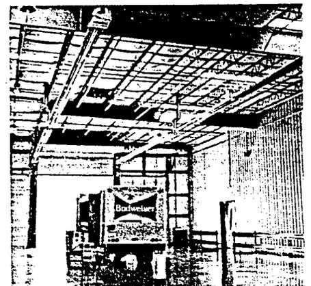
Floors are kept warm by Vantage infrared energy and act as heat reservoirs to provide rapid heat recovery after bay doors are closed in this warehouse/shipping area.
