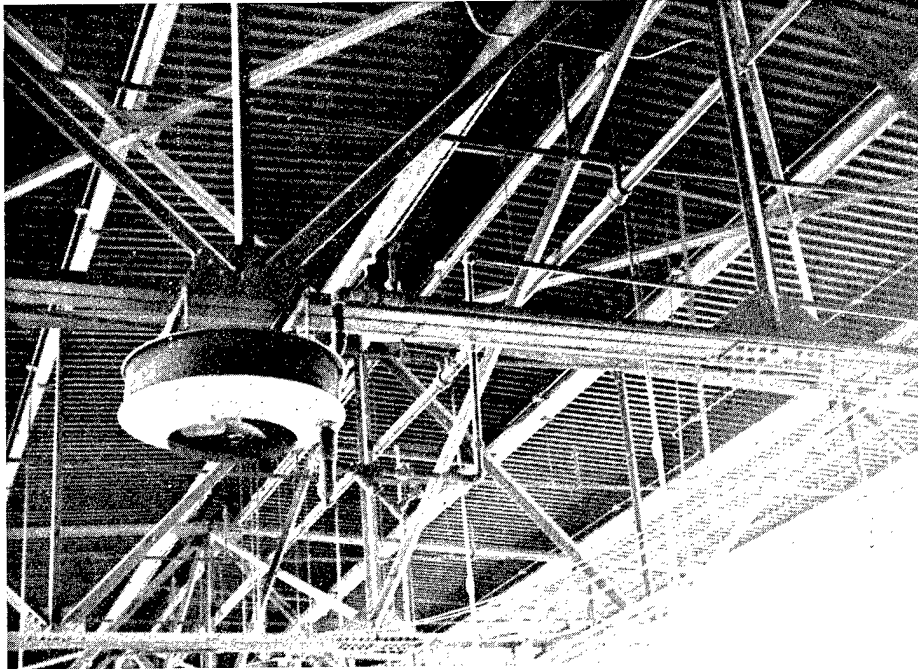
POTENTIAL PROJECT TO INSULATE STEAM LINES AND INSTALL HIGH-BAY AREA DESTRATIFICATION UNITS IN BUILDING 1503
