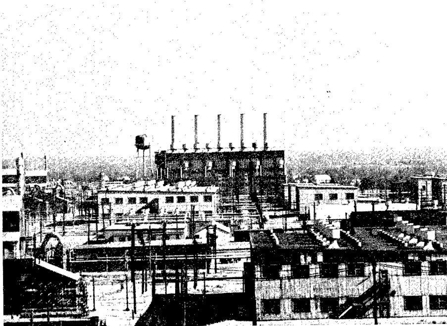
BOILER PLANT — P&E AREA
