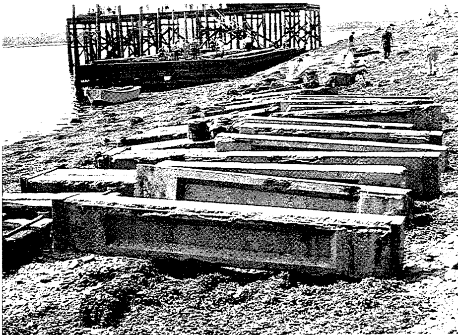
1986 - Nine remaining post-tensioned beams in foreground.
