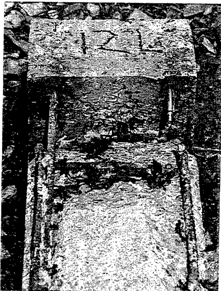
Beam 12 - Landward end - 1994 Concrete and rebar deterioration
