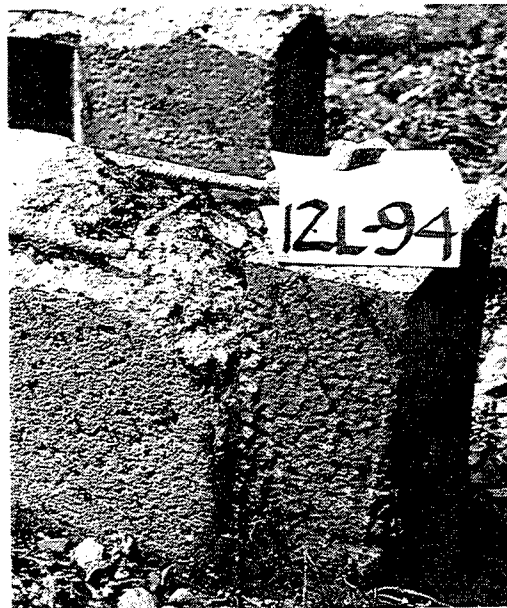
Beam 12 - Landward end - 1994 Concrete and rebar deterioration
