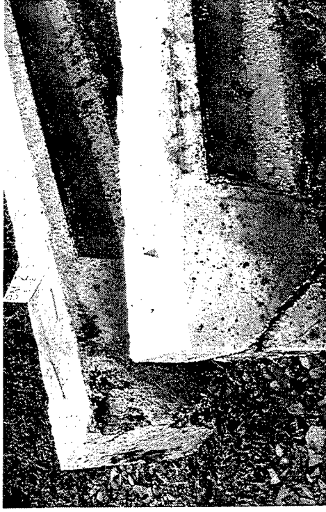
Beam 2 - Landward end - 1982
