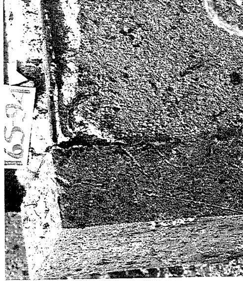
Beam 16 - Seaward end - 1978 Progressive corrosion & spalling Fig. 8-1B
