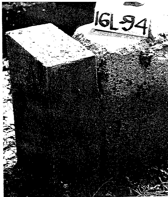
Beam 16 - Landward end - 1994 Fig. 8-2H
