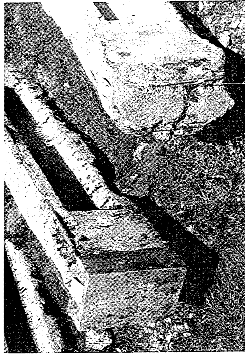
Beam 16 - Seaward end - 1988 Fig. 8-1C
