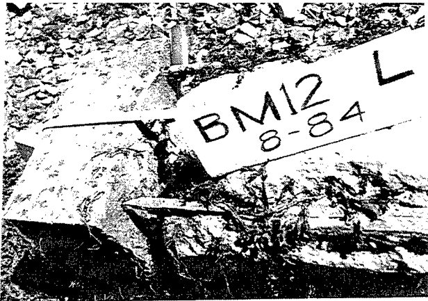
Beam 12 - Landward end - 1984 Corrosion of rebar Fig. 7-3I
