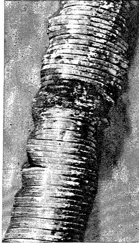
Beam 17 - Outside - 1984 Post-tensioning conduit corrosion Fig. 9-3I
