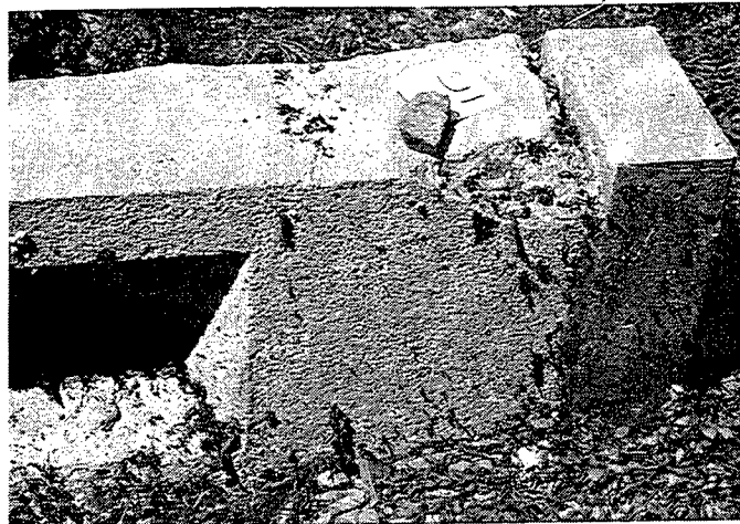
Beam 16 - Landward end - 1988 Fig. 8-2F
