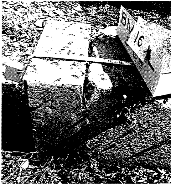
Beam 16 - Landward end - 1984 Concrete interface breakdown Fig. 8-2E
