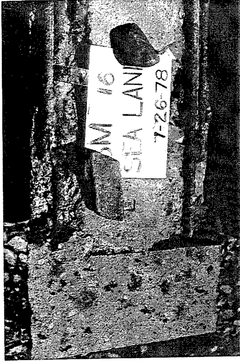
Beam 16 - Seaward end - 1978 Progressive corrosion & spalling Fig. 8-1B
