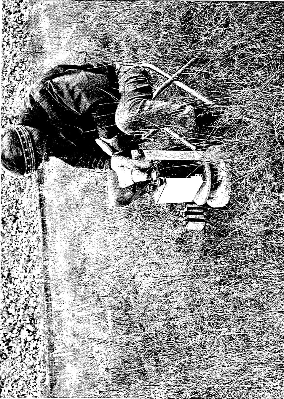
Figure 7. Microgravity measurement at base station
