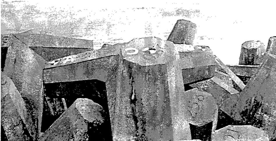
Figure 10. Example of a dolos with three targets established
