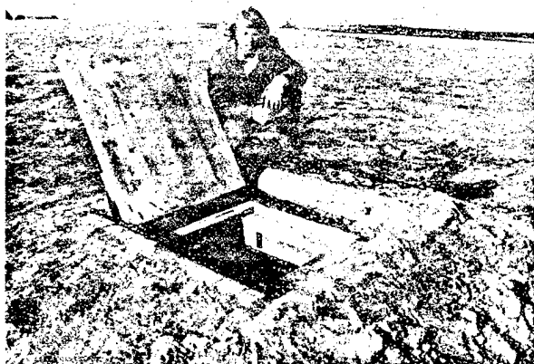
Fig. D.13. Blast door surrounded by 4 blast-protector logs that were notched and nailed together. The wet, mounded soil had been compacted by the blast but not blown away.
