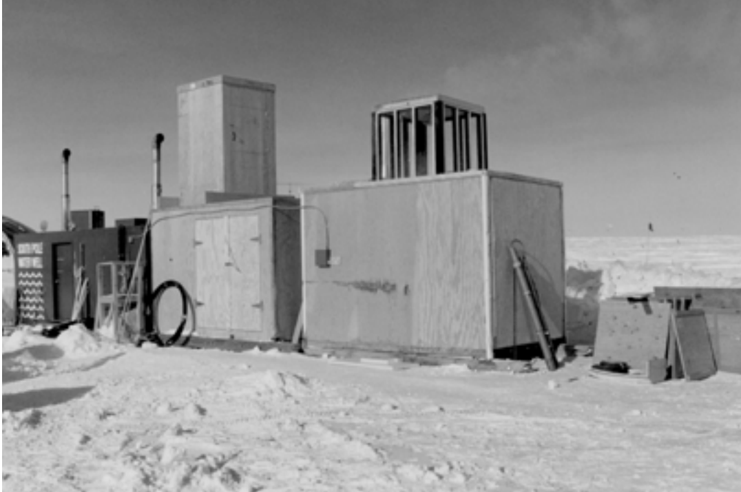
Figure 10. Work space at the SPWW, consisting of a winch room directly over the access hole and an adjoining laboratory.
