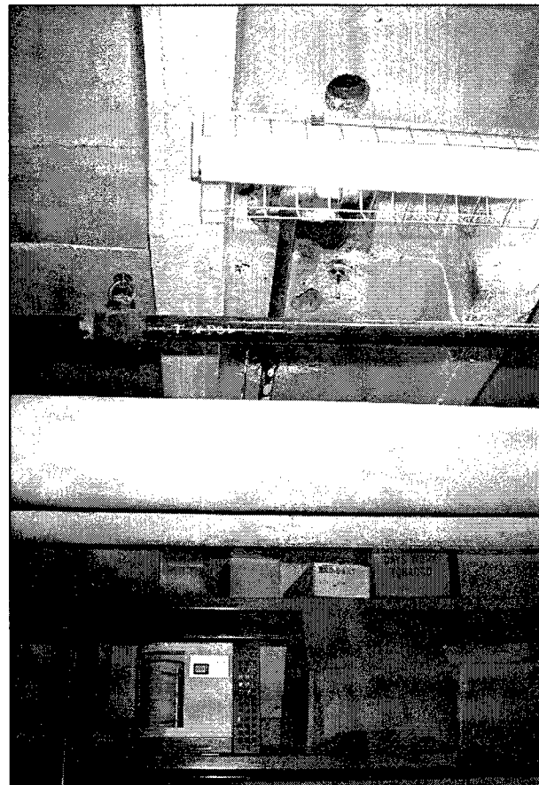
Figure 55. Hygrothermographs are located in each of the collections storage rooms in the LVR building. Also note the sprinkler system, unfiltered fluorescent lights, and holes in the concrete ceiling.
