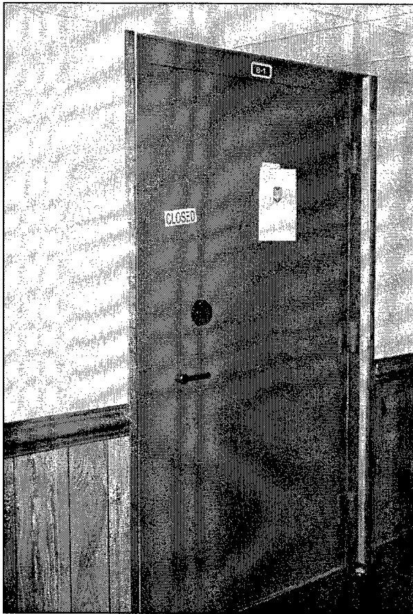
Figure 93. Vault door leading to the collection storage area.
