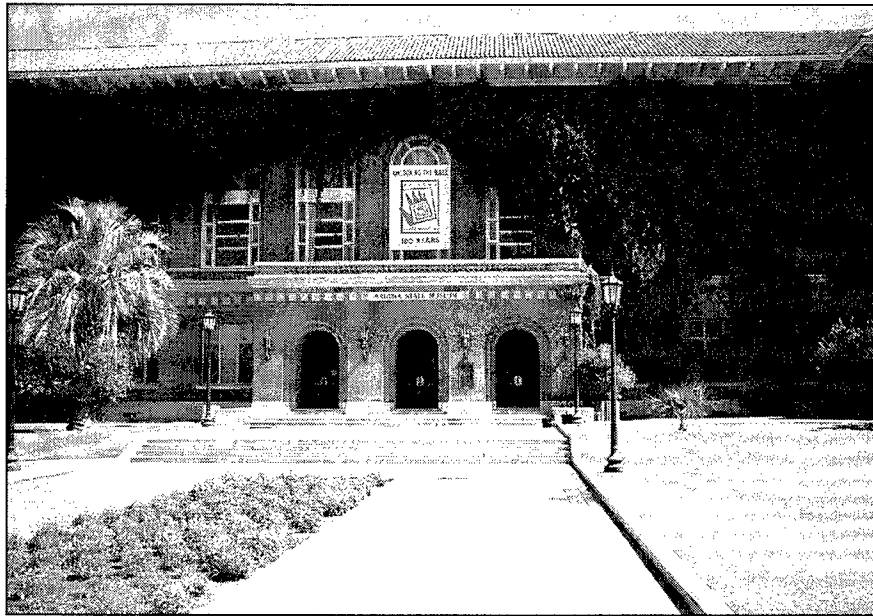
Figure 5. Exterior of ASM's South Building.
