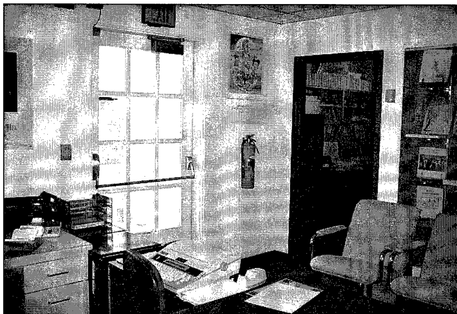
Figure 88. Contact-point intrusion alarms are installed on all doors leading to the exterior. Also note the fire alarm and extinguisher.
