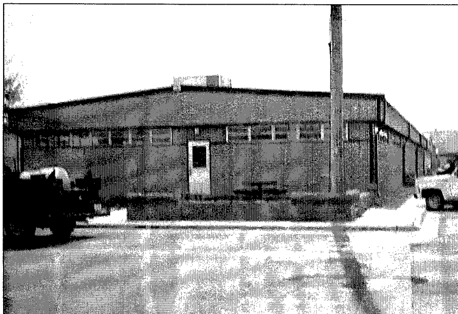
Figure 77. Exterior of the Civil Engineering Building addition housing the Environmental Flight offices.
