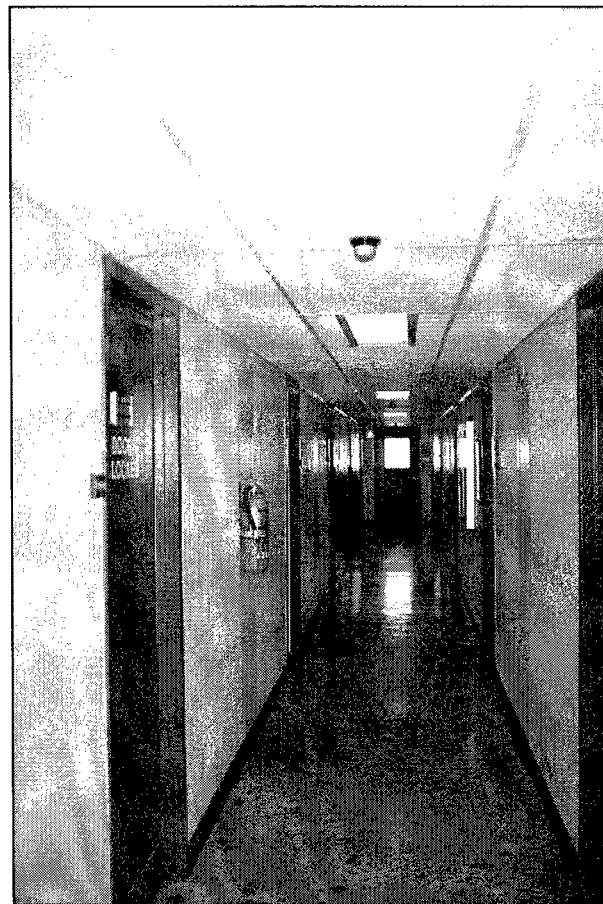
Figure 2. Fire extinguishers, fire doors, and fire walls in the hallway of Building 4300. The motion sensor on the ceiling may be nonfunctional.
