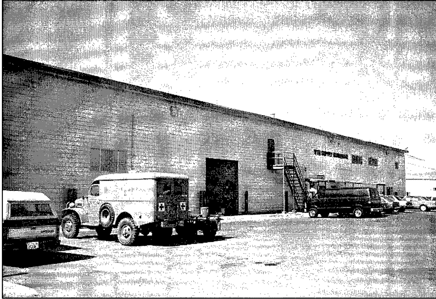
Figure 16. Exterior of Building 2471, location of the Beale AFB Museum.
