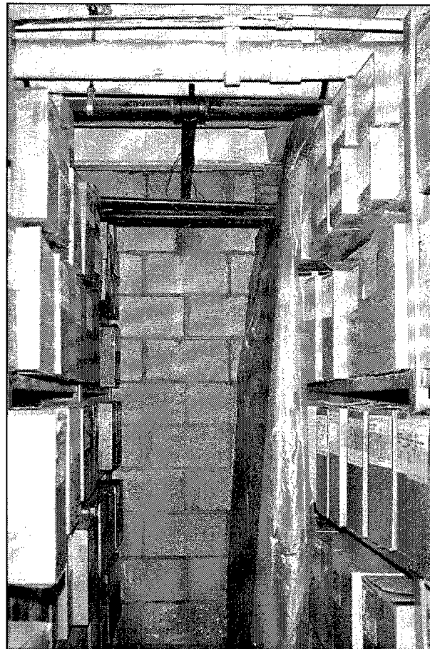
Figure 53. Plastic has been placed over the shelves and primary containers to prevent water damage from leaking overhead pipes.
