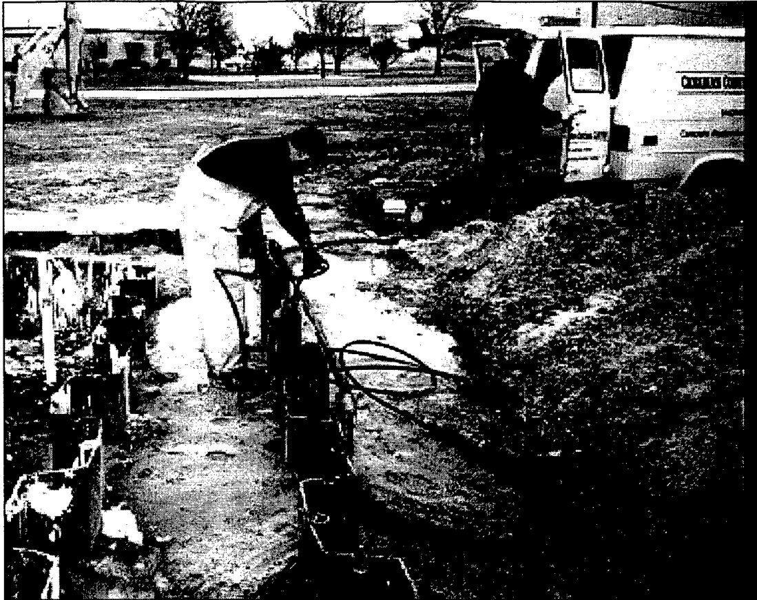
Figure 79. Photograph Showing Sealing of Sheet Pile Joints.
