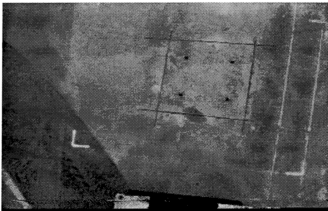
Figure 5-2. Visible Image of Area A: a 7.5 ft (W) by 6 ft (H) grid. Inside, a 2.8 ft by 2.8 ft square was cut from the 6 in. thick asphalt and lifted. A round, 2 ft diameter, 6 in. deep hole was dug under the asphalt and the square was replaced. The 1/8 in. cracks and the 1 in. bolt holes were filled with tar. On the second morning of the test the grid was painted black. This image was taken with the 650 nm filter and the 16 mm lens.
