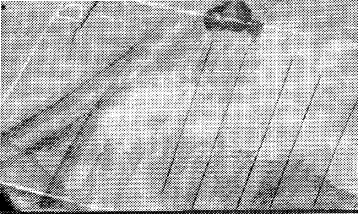
Figure 5-5. Visible Image of Area D: 8.5 ft by 12.5 ft grid. There is a large crack, approximately 2.5 ft long and 0.5 to 1.0 in. wide, just under the "D" at the upper corner of the grid. The other cracks were cut into the asphalt and from the right are: 3/8 , 3/4 , 5/4 , 3, and 5\ 1/8 in. in depth. They were all 1/8 to 1/4 in. wide. Filter: 650 nm; lens: 16 mm. The dark spot at the top of the frame is water. The darker areas in the image are bare pavement and the lighter areas are ground in dirt.
