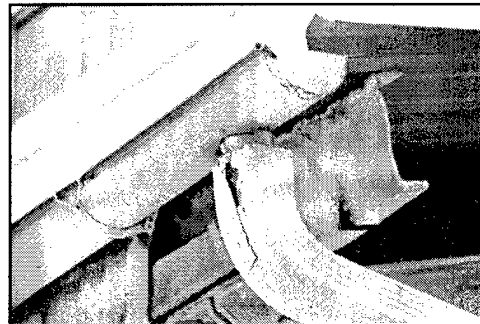
Figure 37. Original half-round gutters shall be maintained; the nonoriginal downspouts should be replaced with original style when they have deteriorated.
