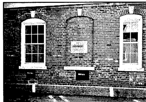
Figure 7. Spray-painted signage is non-compatible and can damage bricks, but this bricked-in window maintains its original character-defining elements and is sensitive to the integrity of the original.
