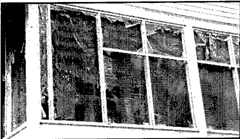
Figure 48. This weatherstripping is not functional, is intrusive to historic appearance, and should be removed.
