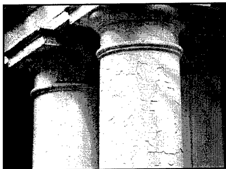
Figure 32. Paint buildup can change the historic character of building elements.
