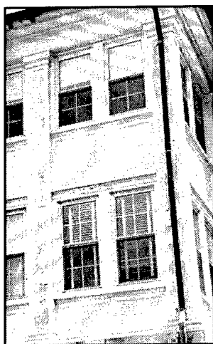
Figure 33. Peeling paint exposes wood to destruction by weathering.
