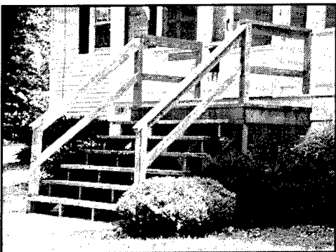
Figure 12. Replacement material and construction of stairs are compatible, but should be painted white to be color-compatible.
