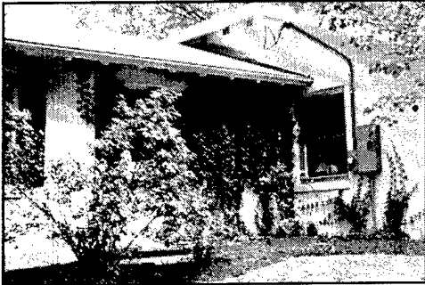
Figure 8. Vines should be cut back to avoid damage to stucco and wood.
