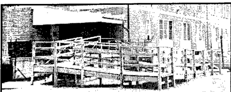
Figure 58. Ramp placed in good location at rear of the building closest to parking lot, but more compatible materials should have been chosen.
