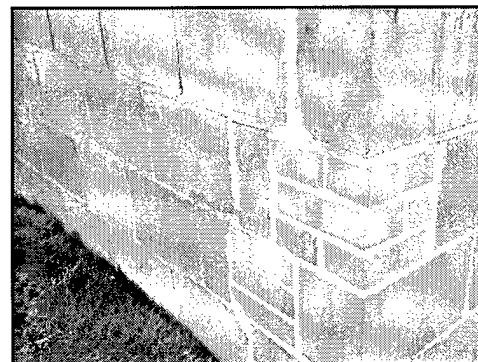
Figure 23. Incompatible masonry units and mortar adversely affect character.
