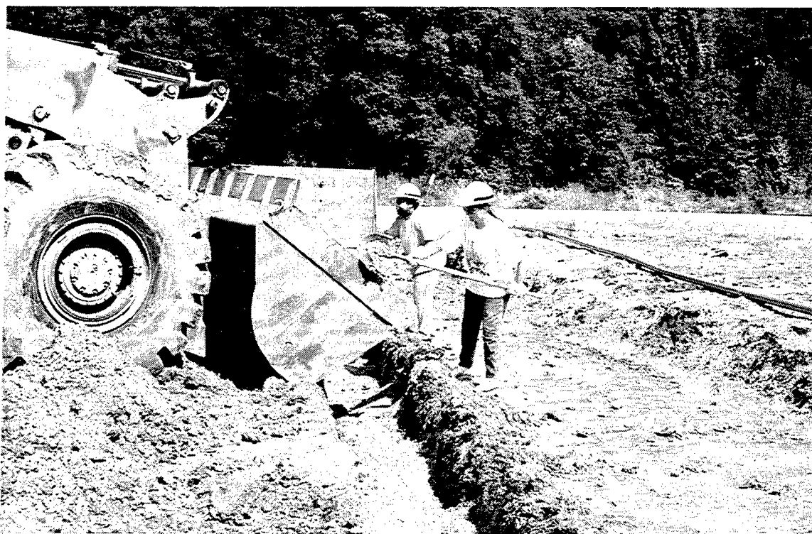
Figure 4. Photograph of test bed instrumentation installation for retrievable microtunneling tests
