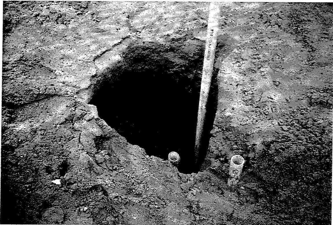
Figure 19. Photograph of surface void at sta 0+06 m (0+20 ft) during reaming drive of retrievable machine test
