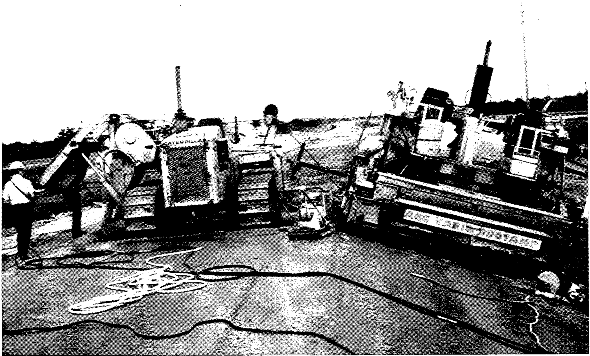
Figure 15. RCC paver connected to a bulldozer for paving slopes at Barker Dam
