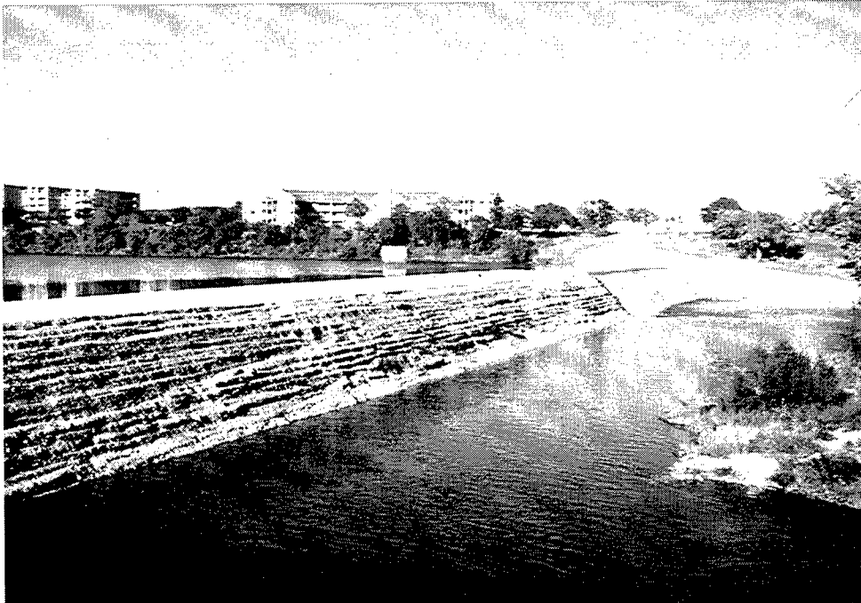
Figure 11. Condition of the RCC following overtopping, Kerrville Pounding Dam
