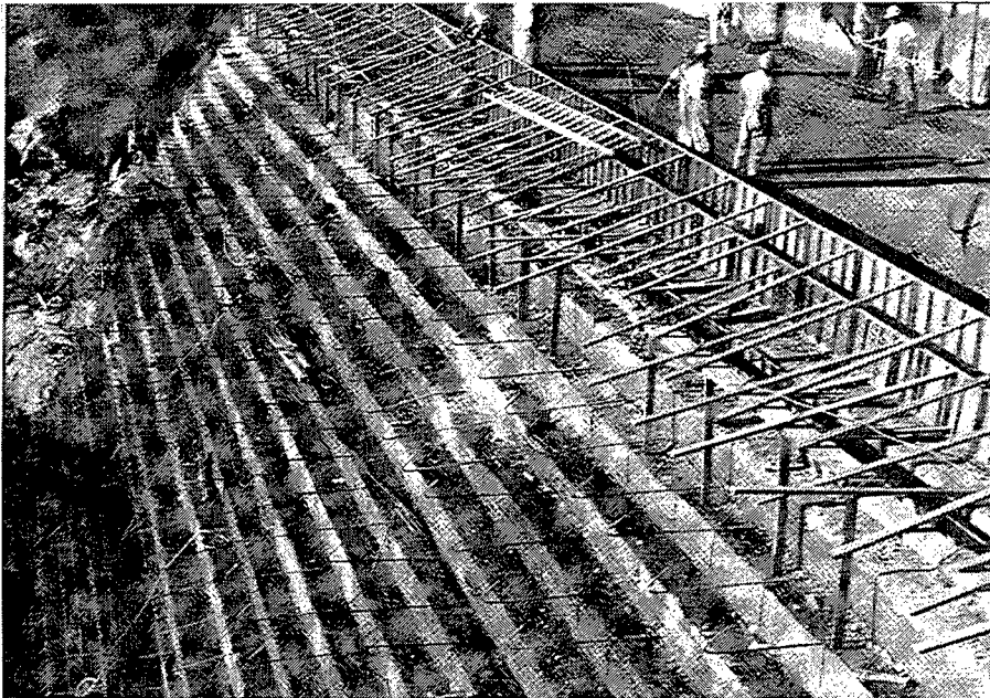
Figure 95. RCC on downstream face of Marmont Dam prior to placing conventional concrete facing (courtesy of Bloomberg 1989)
