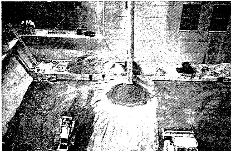
Figure 112. RCC delivered to the lock floor via a drop pipe at New Cumberland Lock (courtesy of Anderson 1984)
