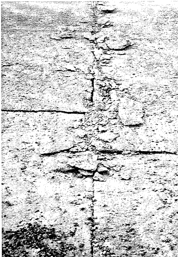
Figure 16. RCC spalling along a joint, Addicks Dam
