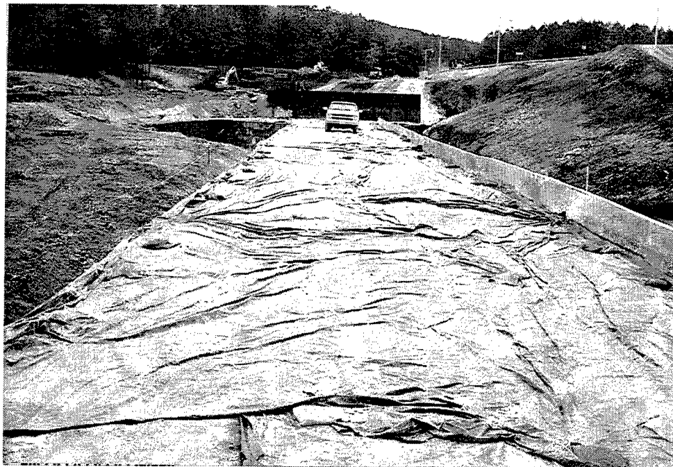
Figure 48. Tarp used for curing RCC at Nickajack Dam
