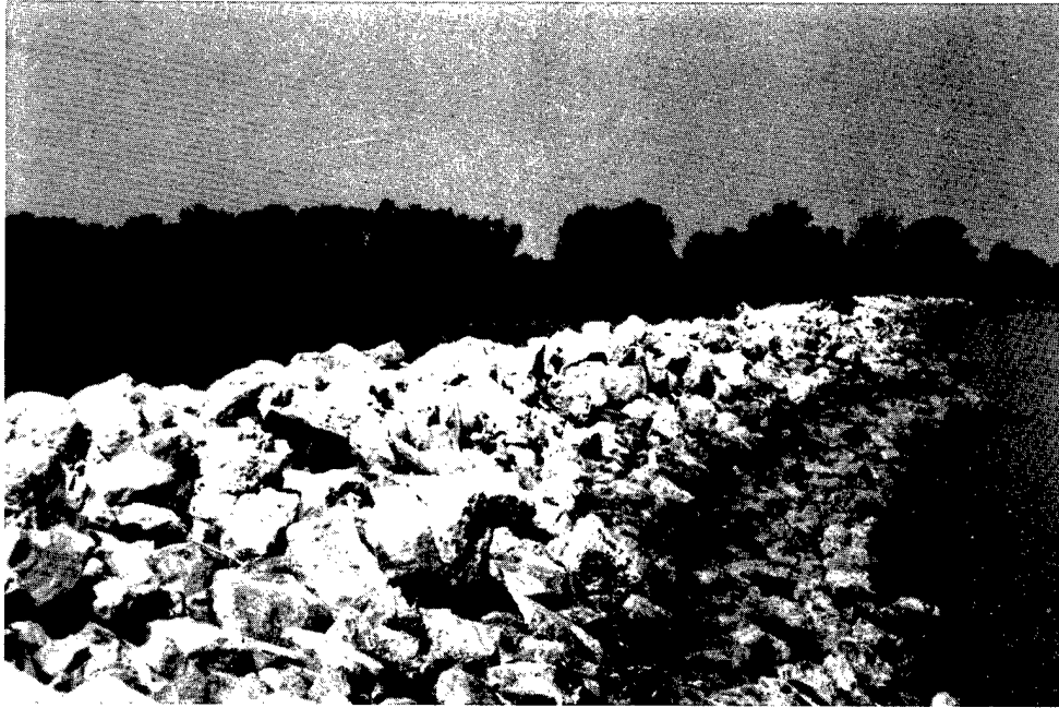
Figure 9. Rip-rap dike separating Lake Erie (right) from Darby Marsh (left); this wetland is part of the Ottawa National Wildlife Refuge (August 1982).
