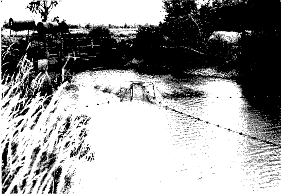
Figure 62. Water level control structure between upper Sandusky Bay and Winous Point Marsh. Trapnet in foreground used to determine fish utilization of marsh (July 1984).
