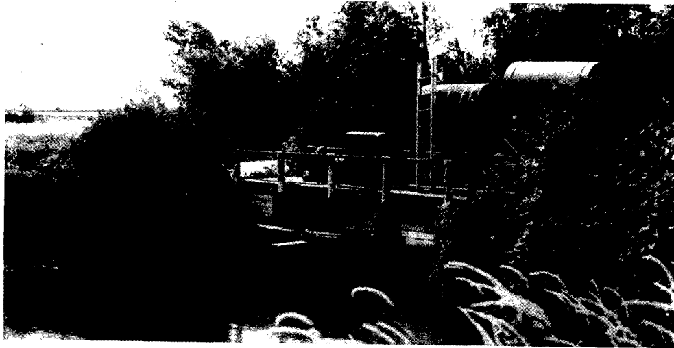
Figure 92. Water level control structure between Sandusky Bay and Winous Point Marsh; note bar screen at left side to exclude carp (July 1984).
