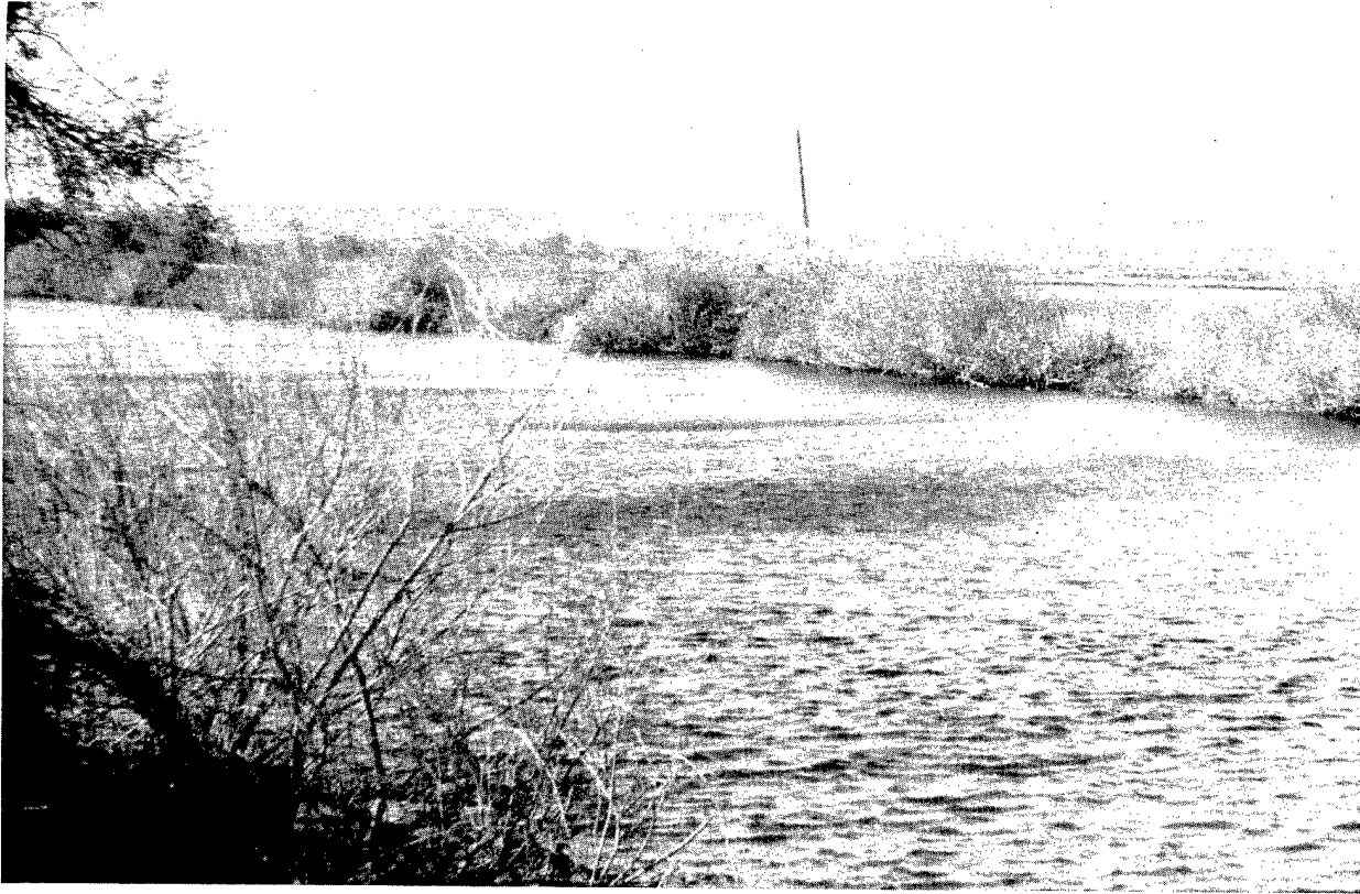
Figure 5. Privately owned and maintained levees on Sevenmile Slough. Note steepness of edge, erosion, and narrow riparian band extending into water.
