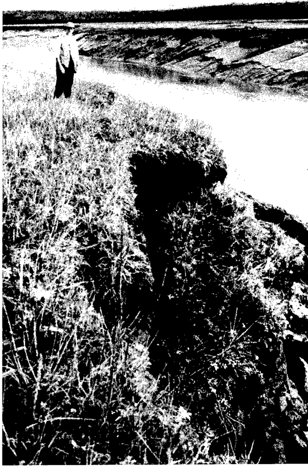
Figure 54. Rotational slump block failure at River Section-North.
