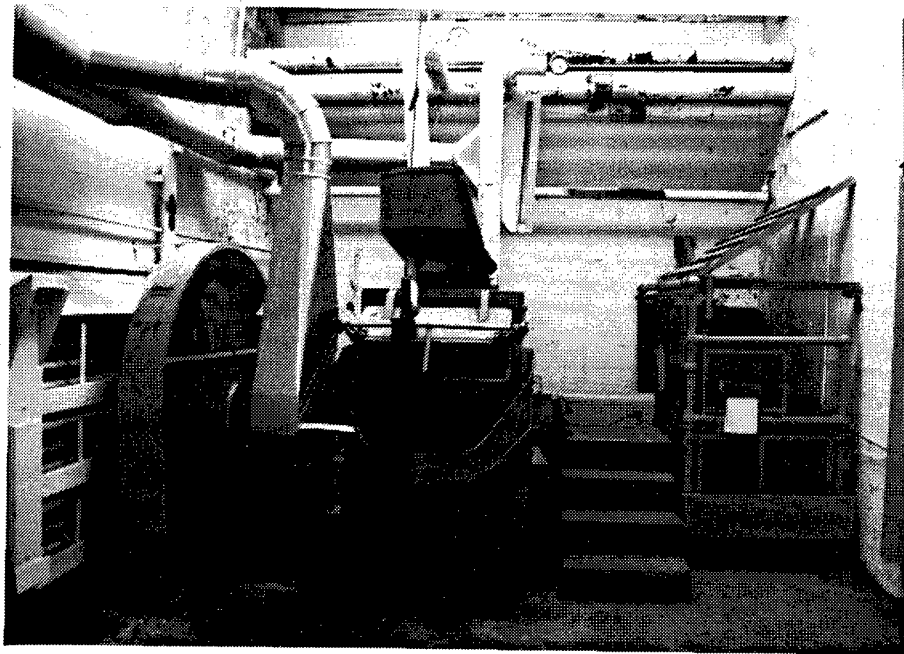
Figure 58. Building 1508: Macerator that improved the colloid consistency and reduced solvent evaporation.
