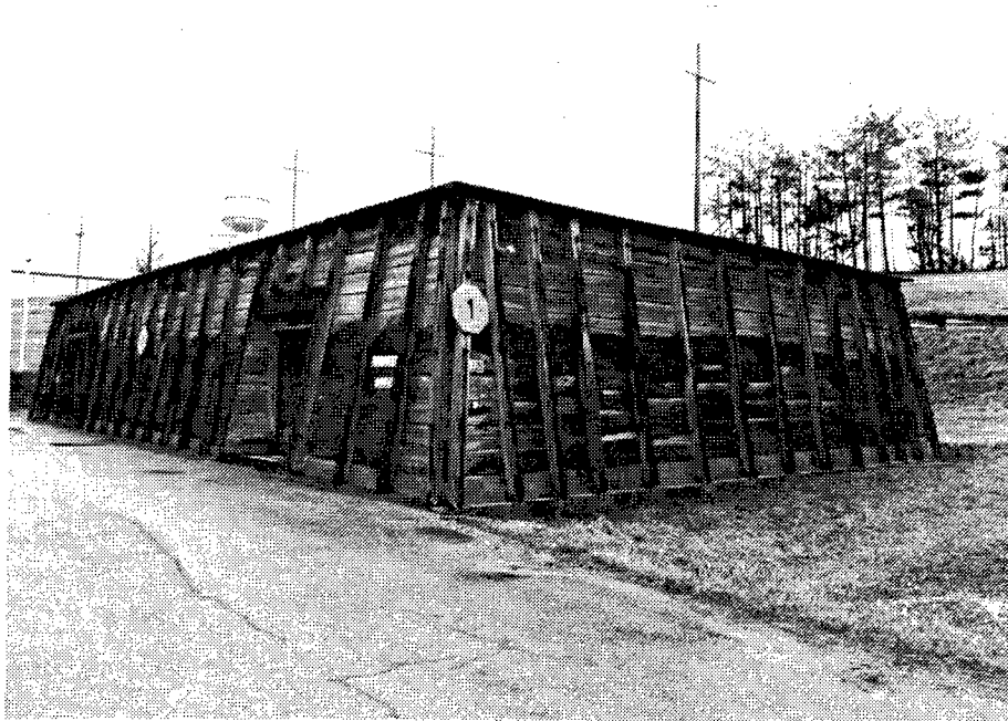
Figure 185. Building 225: Smokeless Powder Magazine.
