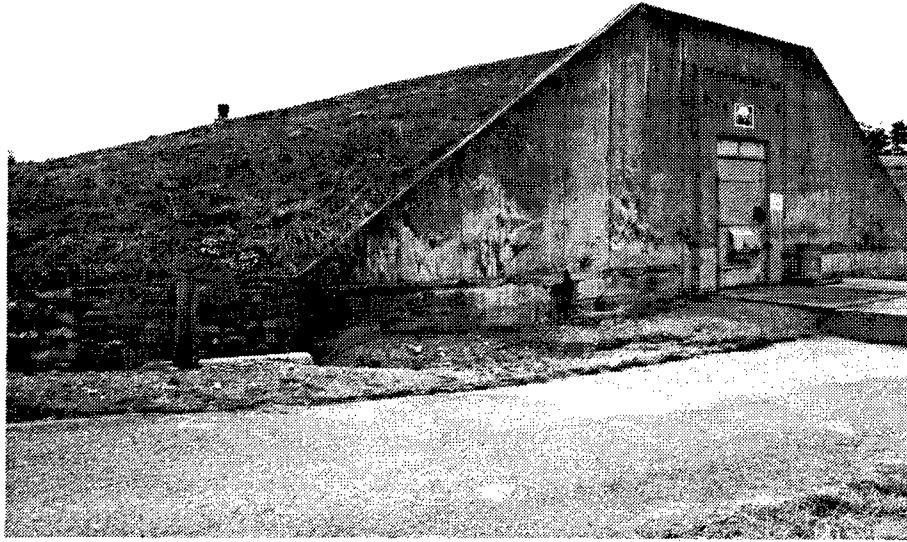
Figure 182. Building 1107: Igloo Storage Magazine with a ventilator extending up from the back of this earthen-covered structure.
