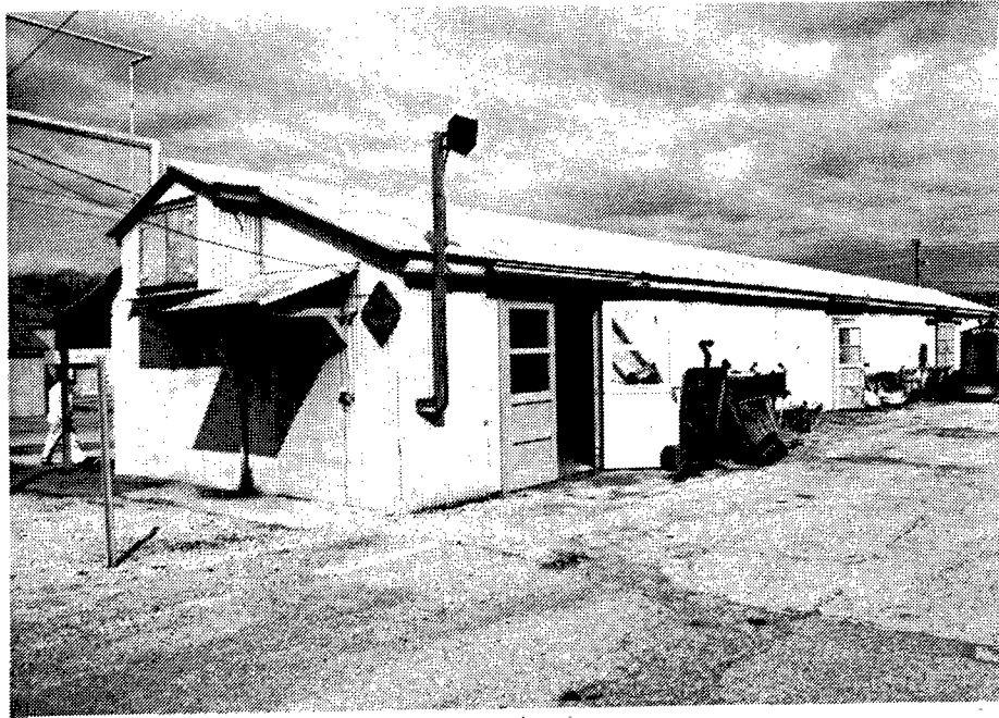
Figure 127. Building 3713: Mobilization Storage.
