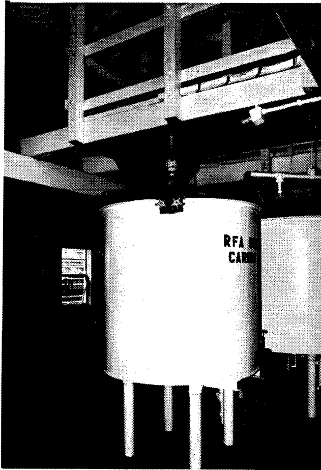
Figure 231. Building 419: Carbon Tank.
