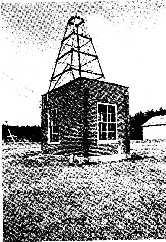
Figure 234. Building 926: Magazine Area's 12-inch well with pump house.
