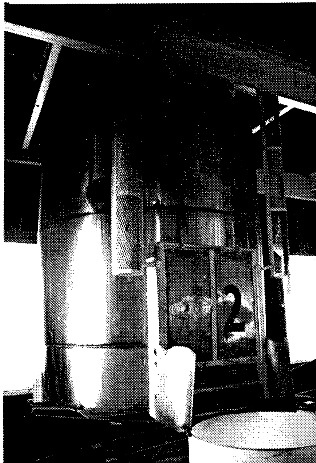
Figure 20. Building 1012: Cyclone cotton hopper on the third floor where cotton from the Dry Cotton Conveyor was received.
