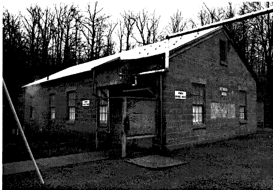
Figure 202. Building 7809: Change House for females.
