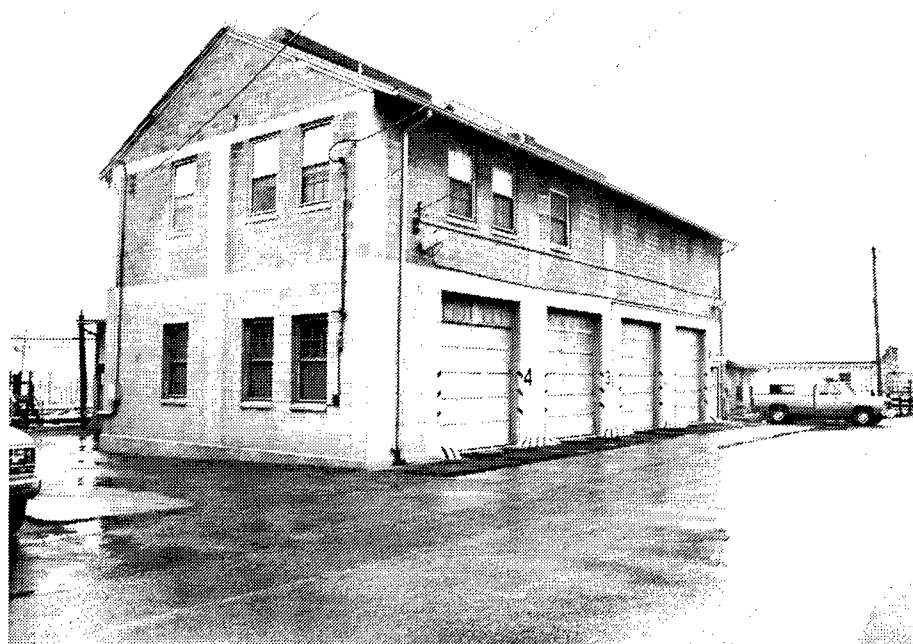
Figure 217. Building 222: Two-story Fire Station containing bays 1 through 4.
