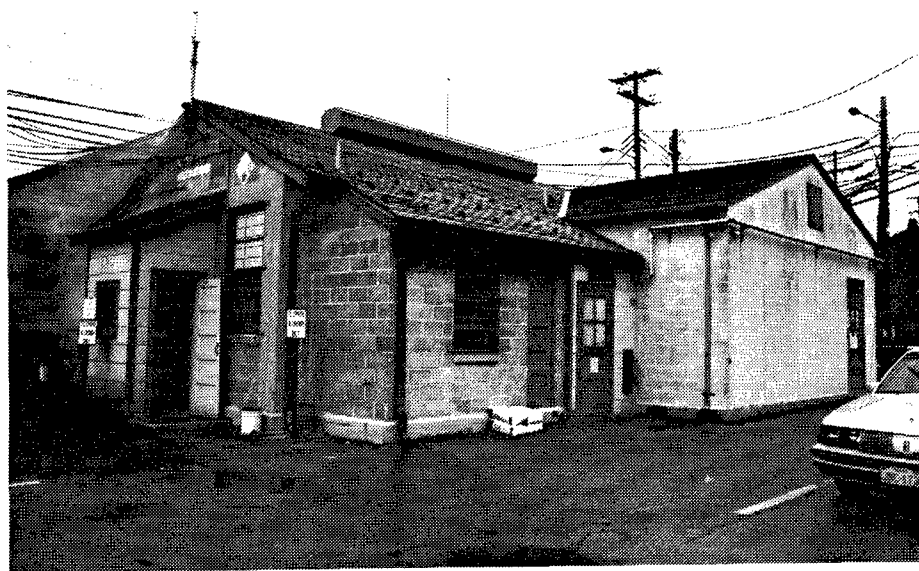
Figure 211. Building 263: Telephone Building.
