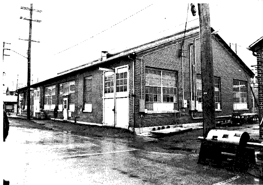
Figure 157. Building 520: Weld Shop.
