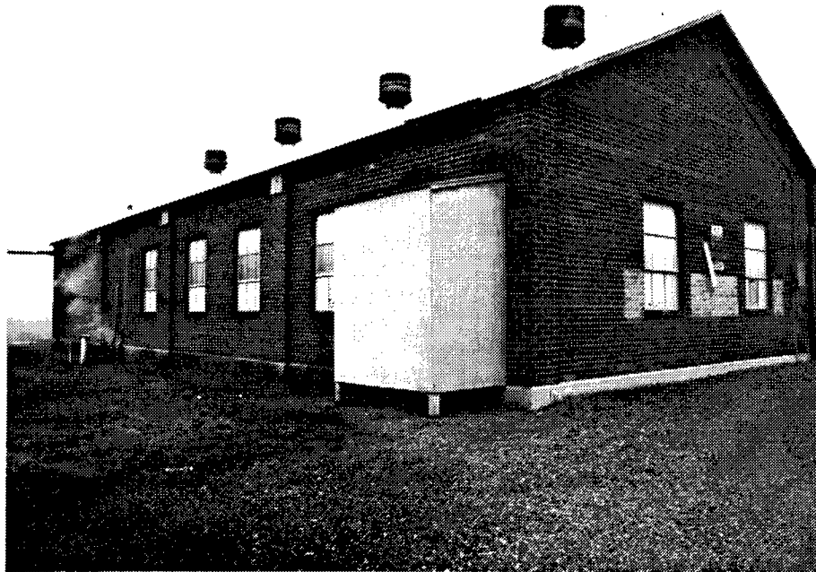
Figure 198. Building 3718: Change House.
