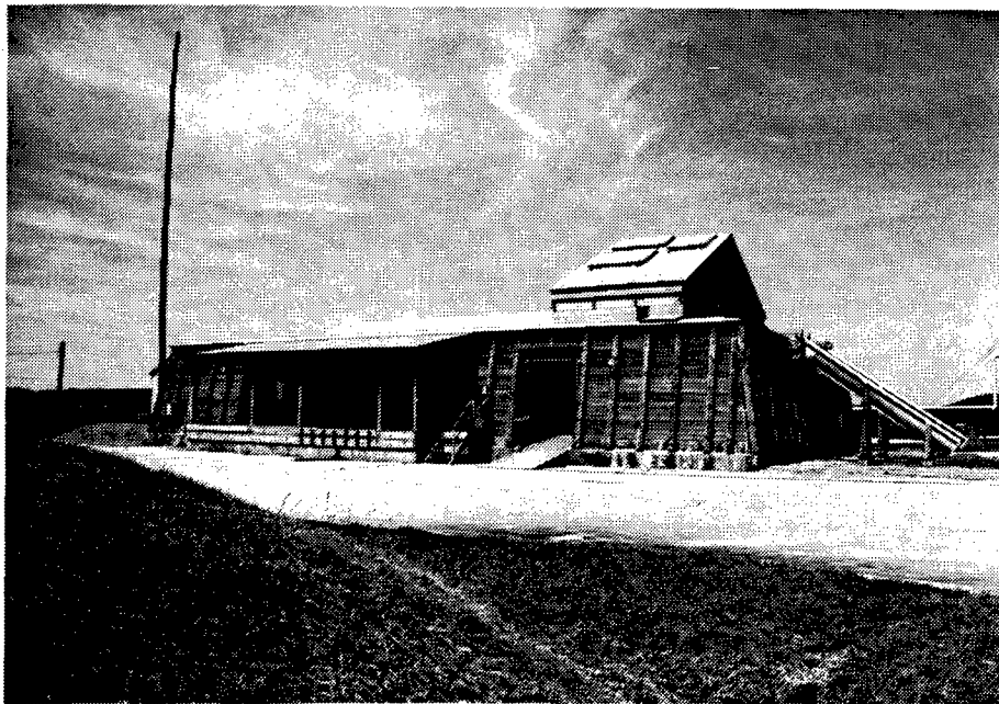
Figure 130. Building 4912-02: Small Grain Loading House.
