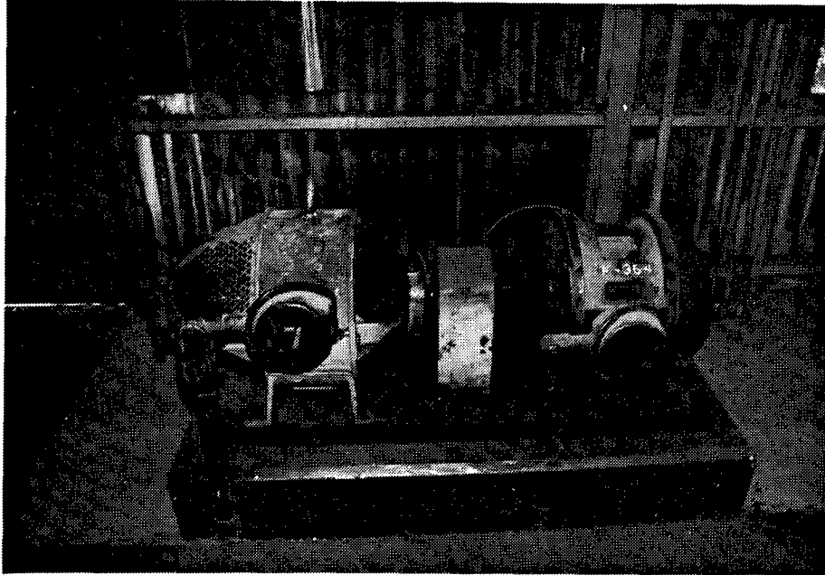
Figure 253. Building 700: Exciter motor that converts DC to AC for the air compressor's control panel.
