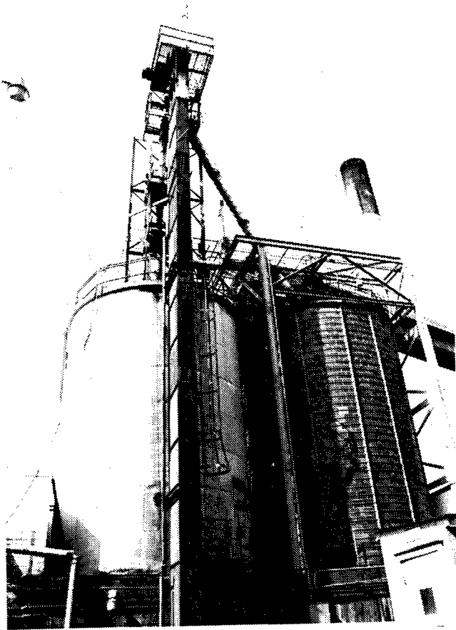
Figure 251. Building 4329: A ceramic coal silo (on the right), a steel coal silo (on the left), and a coal elevator.
