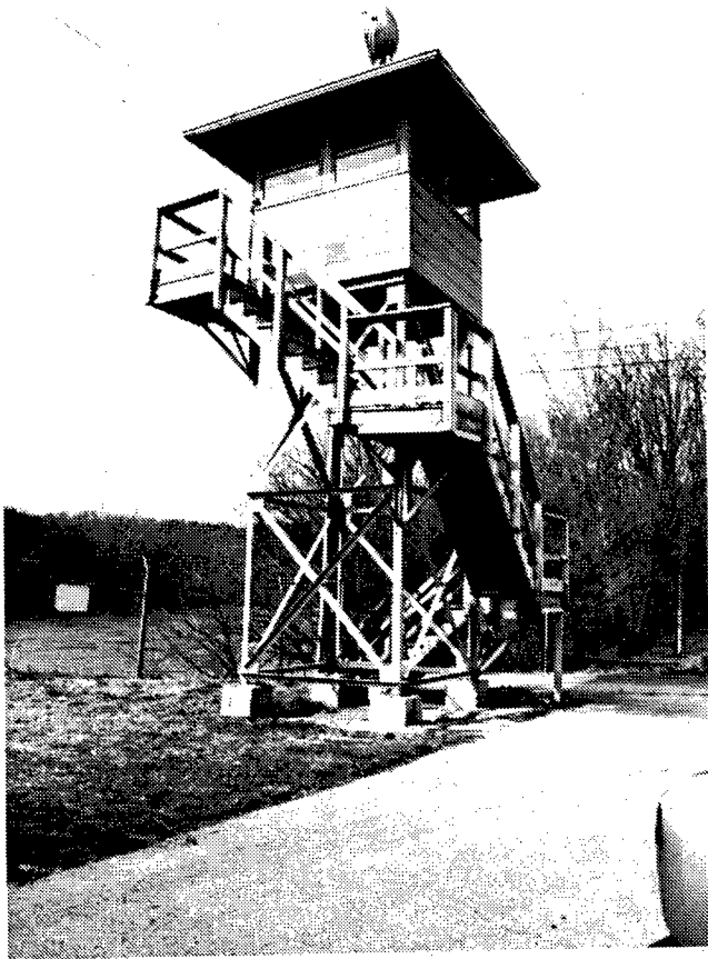
Figure 215. Building 221-5: Sentry House.
