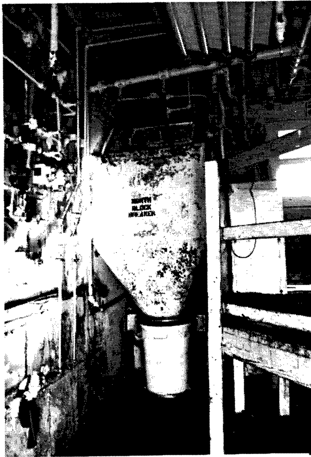
Figure 71. Building 1561: Interior of the Block Breaker House.
