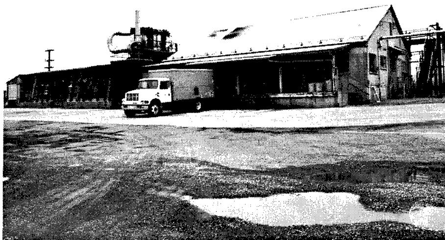
Figure 41. Building 3524: Chemical Grind House.
