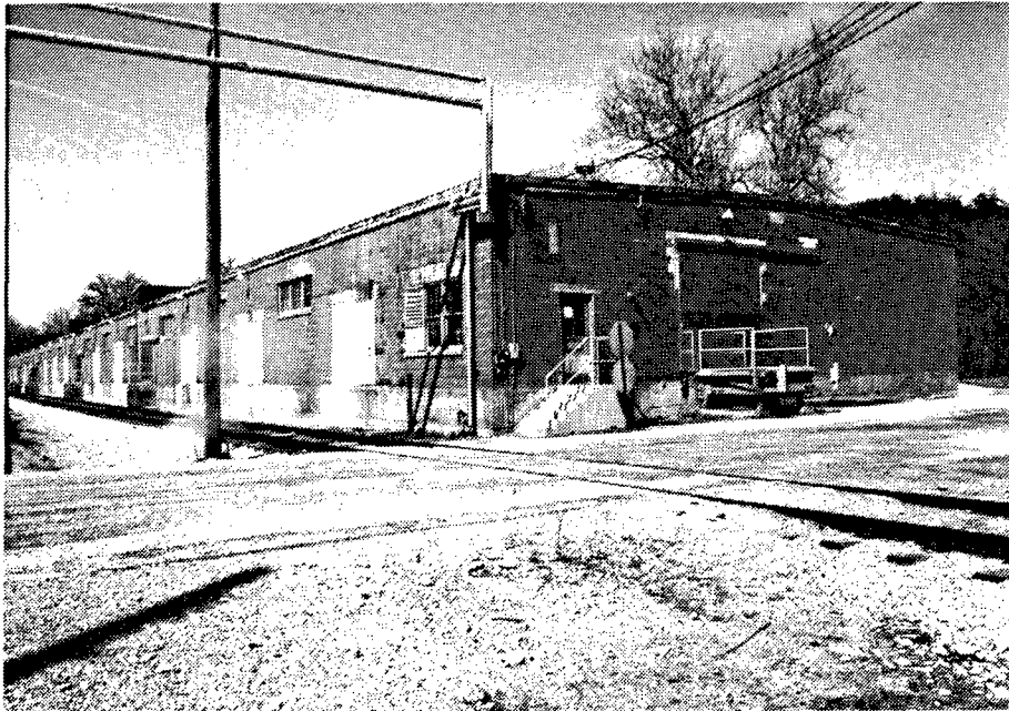
Figure 181. Building 9387-1: Cinder Block Warehouse.
