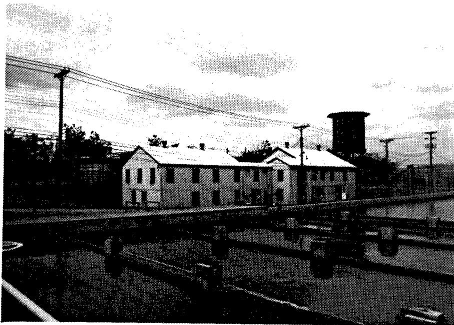
Figure 227. Building 419: Drinking Water Plant with original wooden water tanks.
