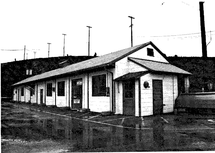
Figure 139. Building 203: Garage which has served as a data center in recent years.
