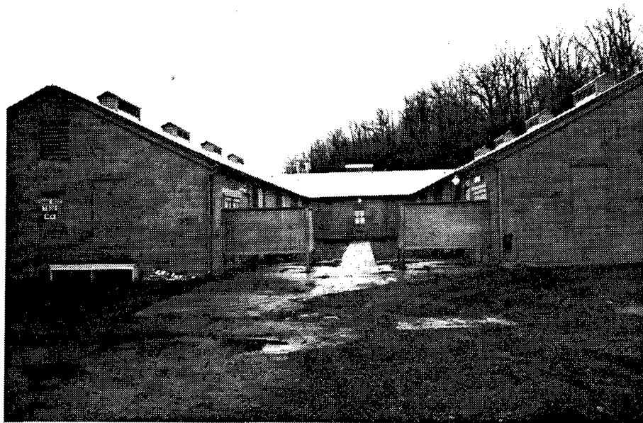
Figure 201. Building 7808: Change House for males.
