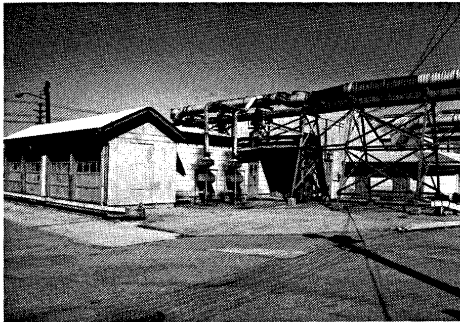
Figure 77. Building 1513: Finishing Press and Cutting House where the loading station is equipped with four garage-like doors with Cyclone Ventilators on the back side of the building.
