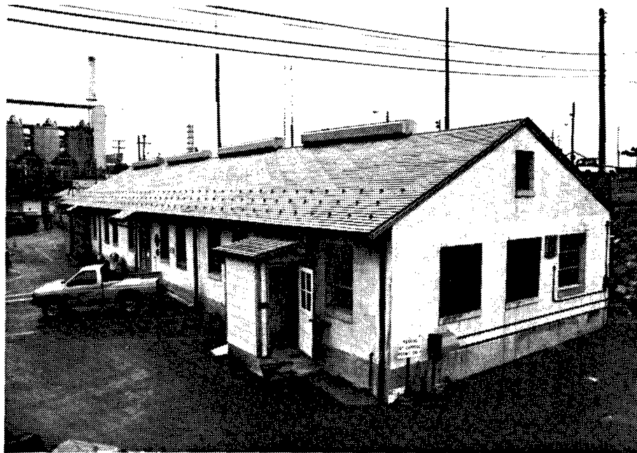
Figure 216. Building 235: Police Station.
