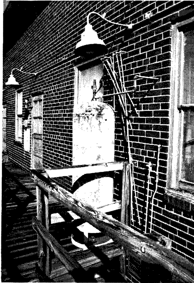
Figure 16. Building 1012: Pressure tank on the fourth floor of this building.
