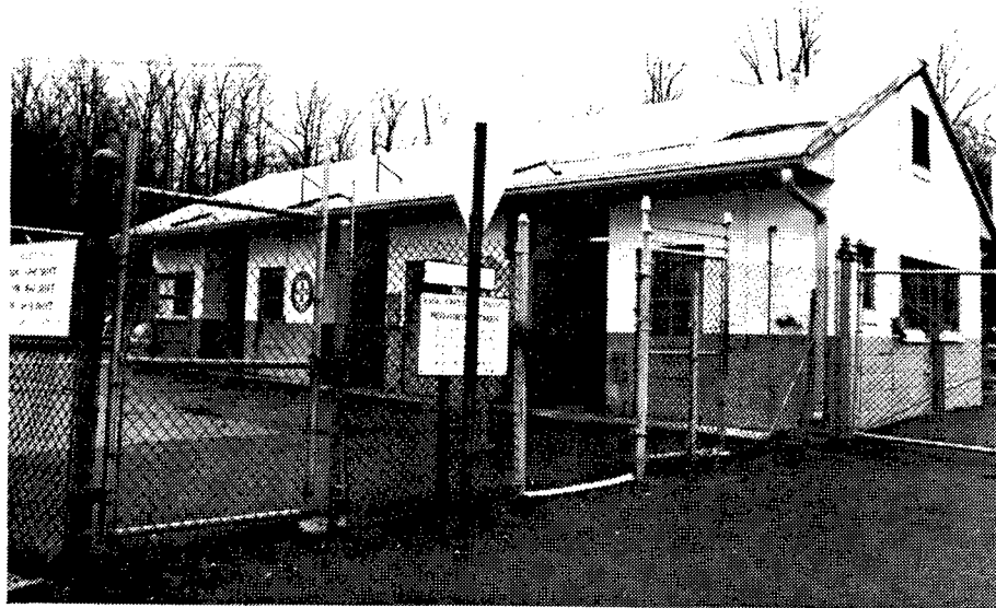
Figure 213. Building 223: Sentry Station/Plant Gate House #3.
