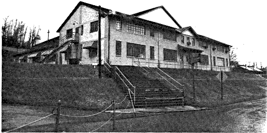
Figure 206. Building 216: Fitness Center or Gym.
