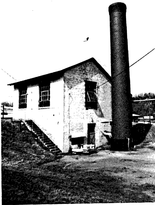
Figure 8. Building 7100: Office with incinerator.
