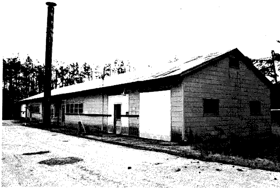
Figure 5. Building 521: Magazine Office and Change House with a "chimney" that serves as a heater smokestack.
