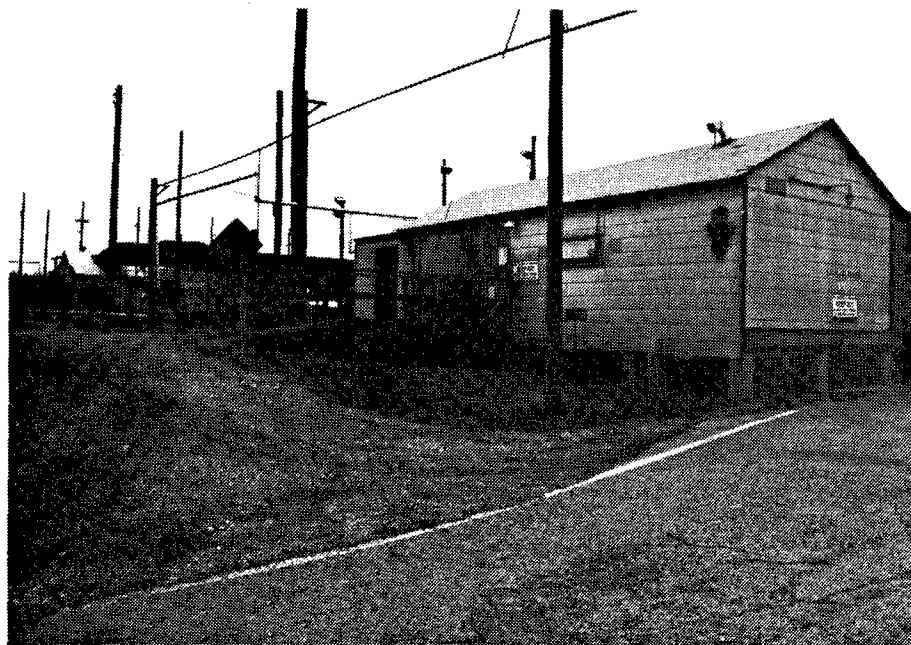
Figure 44. Building 3650: Cotton Store Mix House.
