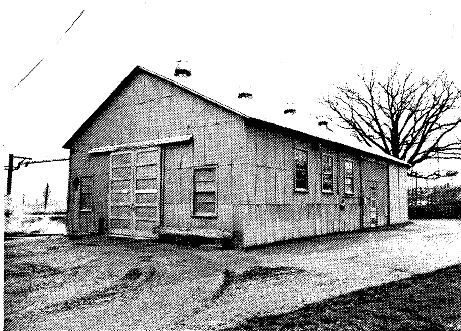
Figure 190. Building 226: Tire Storage Shed with aluminum siding.
