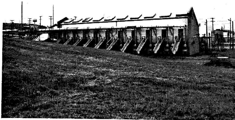
Figure 72. Building 1513: Finishing Press and Cutting House equipped with "blow" panels for explosions that also provided easy access to the machinery for repairs.
