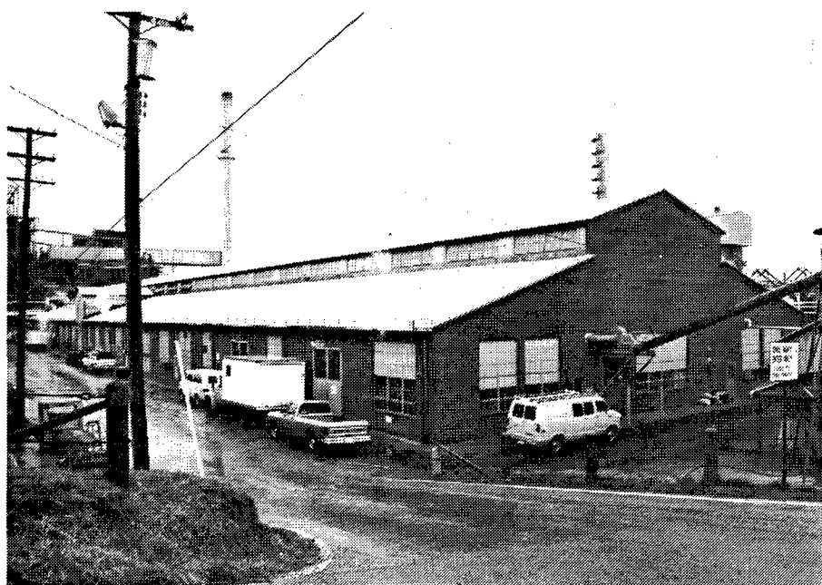
Figure 140. Building 500: The Combined Shop where metal and woodworking took place. Devices were designed and manufactured here to meet OSHA safety laws that required safety cages, bars, and panels on much of the plant equipment.
