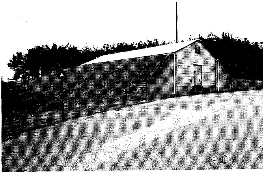
Figure 184. Building 4603-32: Richmond Magazine.
