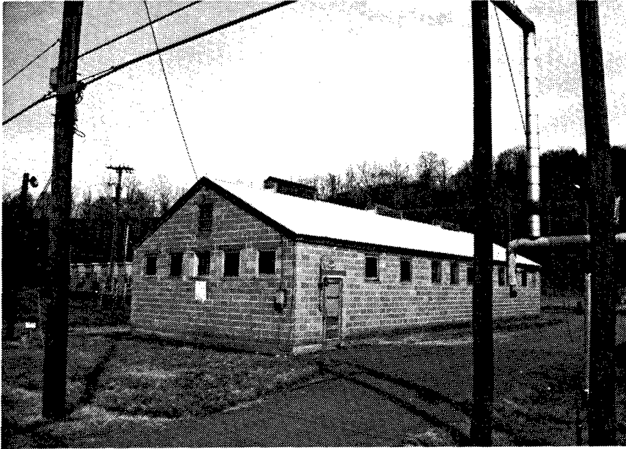
Figure 203. Building 9361-03: Cinder block Change House.
