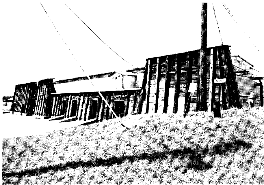
Figure 134. Building 2924-1: Large Motor Load House.
