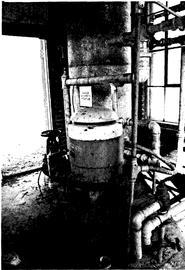
Figure 235. Building 926: Peerless pump.
