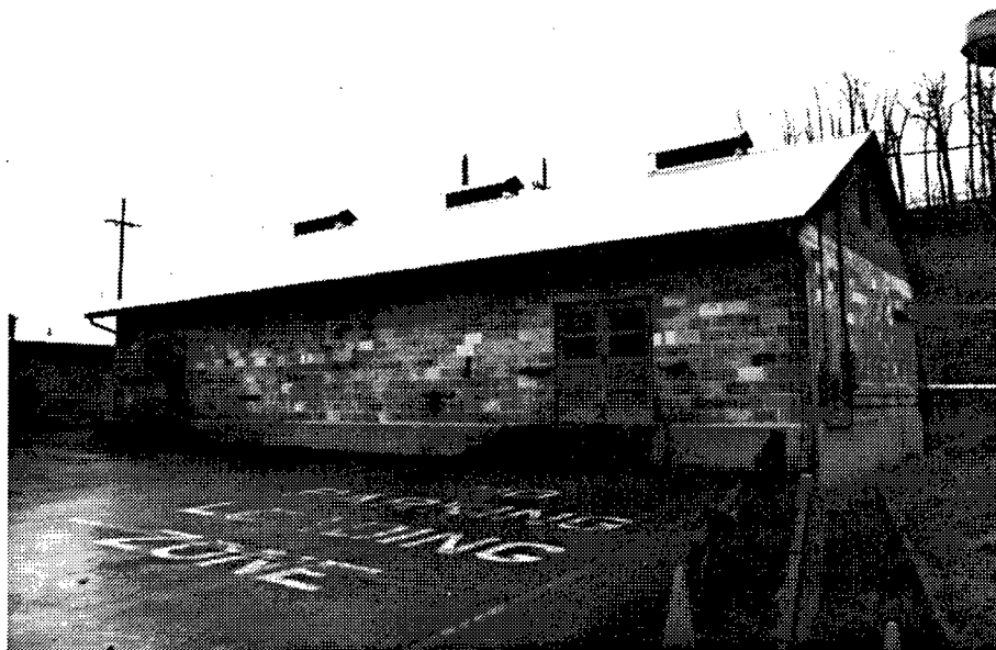
Figure 179. Building 4723: This General Purpose Warehouse contains two walk-in wooden refrigerators.
