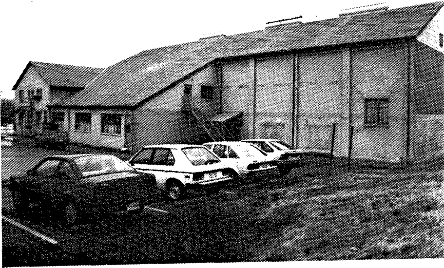
Figure 207. Building 216: West side of the gym.
