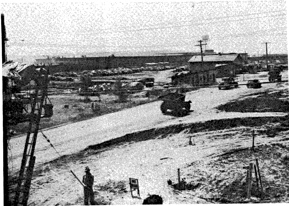
Figure 33. Overview of LCOP during construction, ca. 1941 (original photograph on file, LCAAP).
