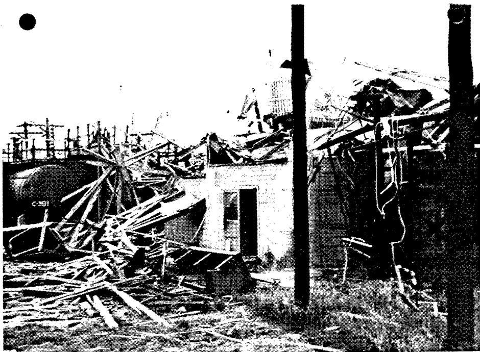
Figure 48. Close-up view of above building damaged during propellant explosion at BOW, World War II Operation (original photograph on file, BAAP Library).
