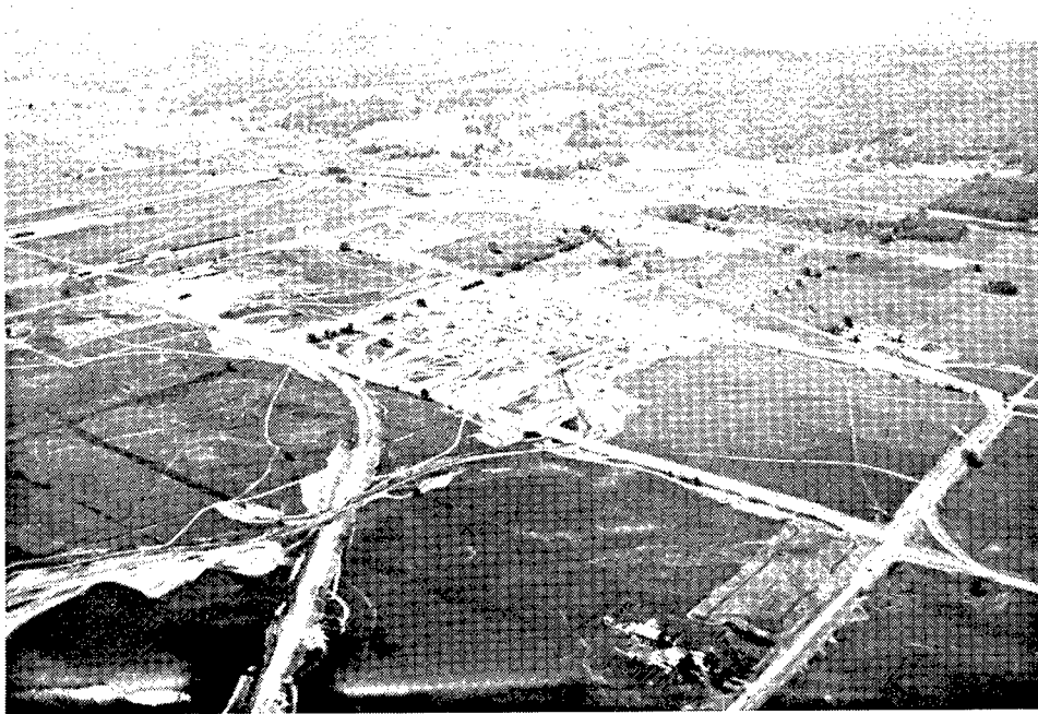
Figure 25. Overview of BOW during construction, World War II Operation (original photograph on file, BAAP Library).
