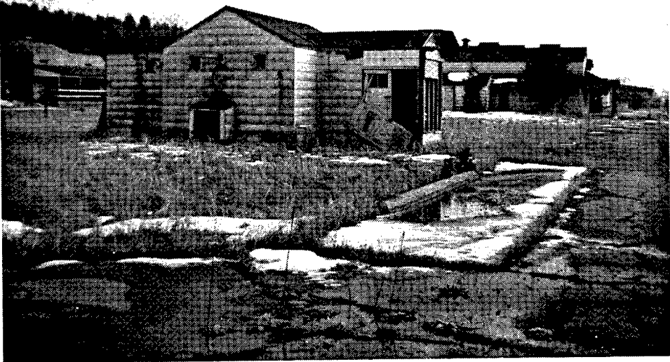
Figure 52. Modern view of dilapidated building at BOW (Bear Creek Archeology, Inc., photograph).
