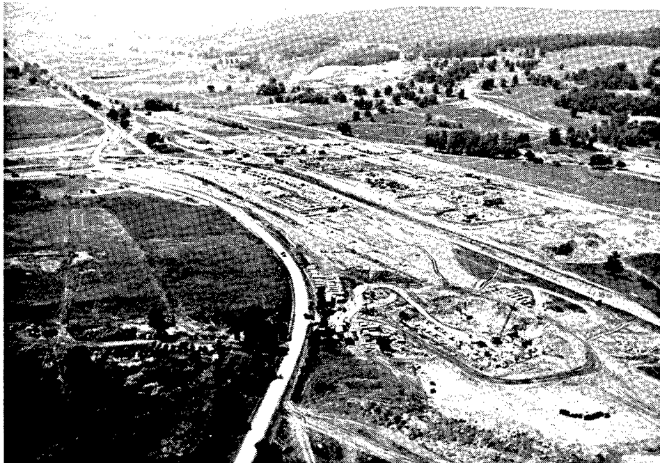
Figure 20. Overview of BOW during construction, World War II Operation (original photograph on file, BAAP Library).
