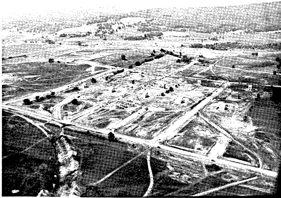
Figure 19. Overview of BOW during construction, World War II Operation (original photograph on file, BAAP Library).
