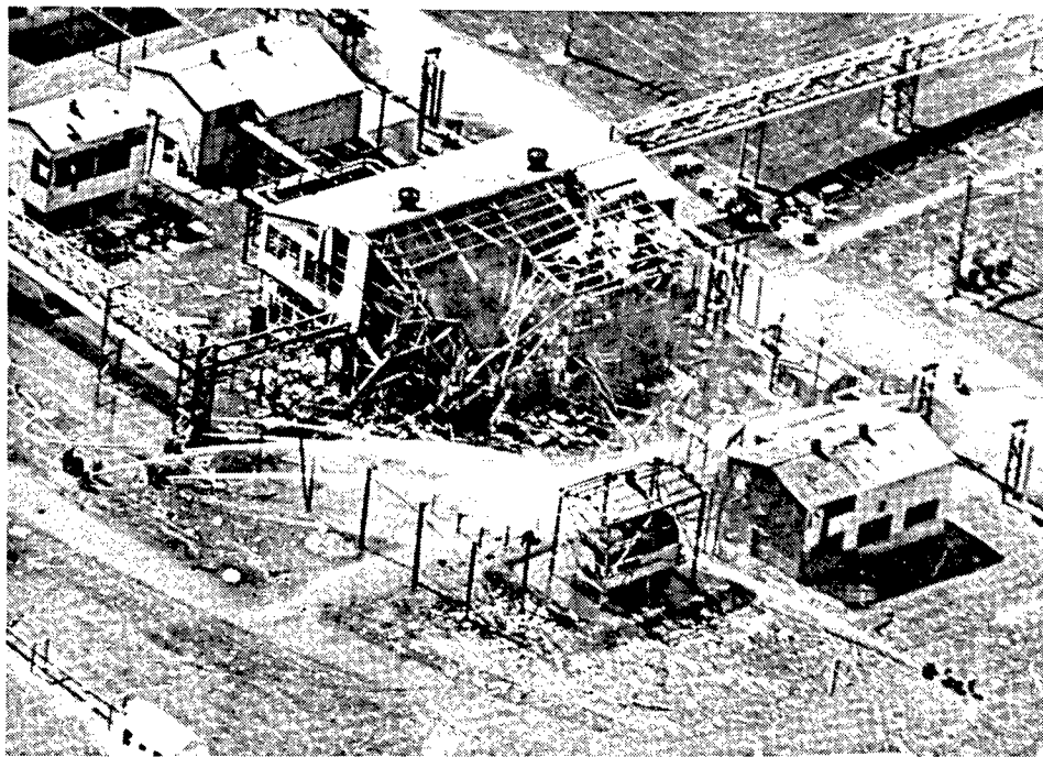
Figure 51. Building damaged during propellant explosion at BOW, Korean Operation (original photograph on file, BAAP Library).
