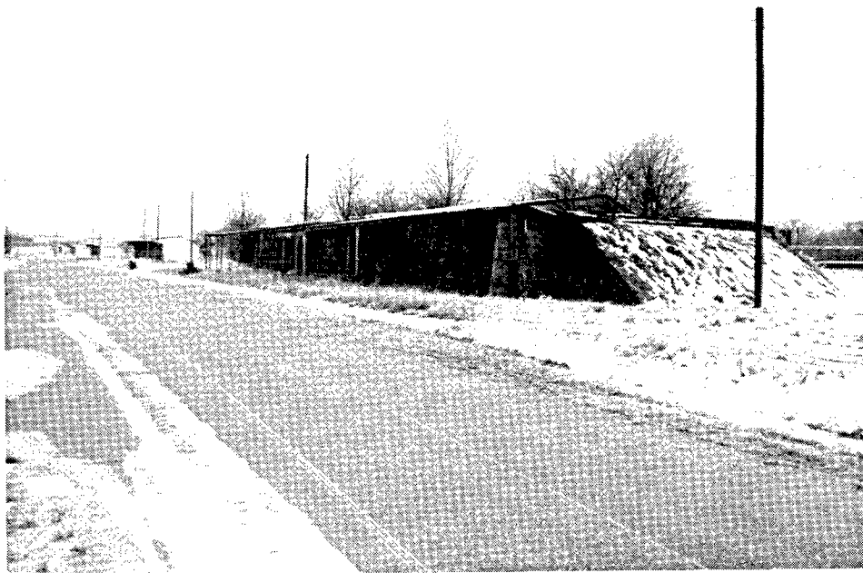
Figure 13. Barricade at Pre-Dry House at BAAP (Bear Creek Archeology, Inc., photograph).
