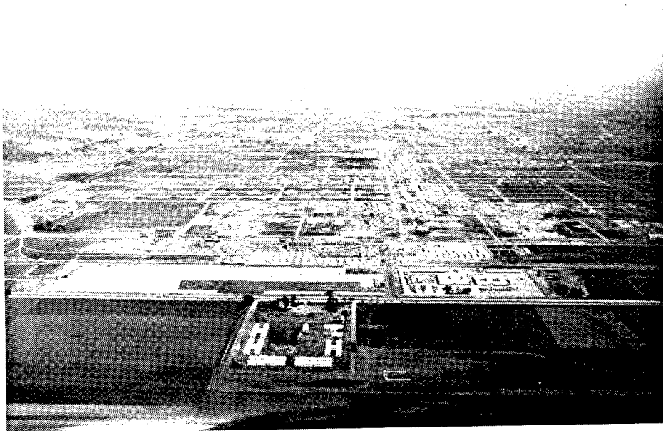
Figure 42. North Badger Village with BOW in background, World War II Operation (original photograph on file, BAAP Library).
