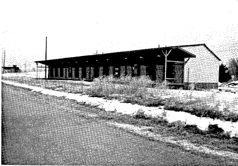
Figure 7. Typical Pre-Dry House at BAAP (Bear Creek Archeology, Inc., photograph).
