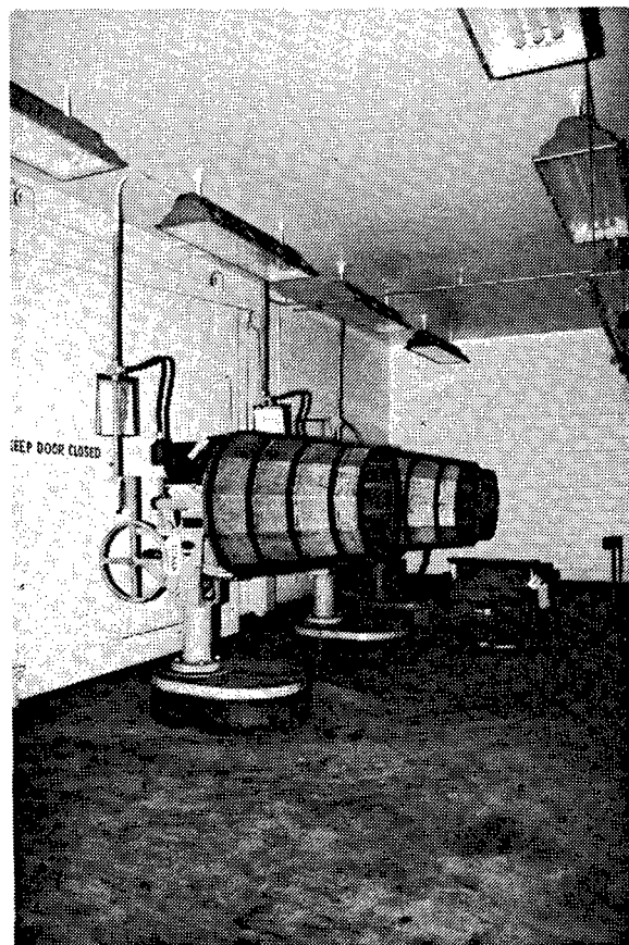
Figure 62. Building 102: Tumbling Barrel (bullet polisher in Tracer Area) manufactured in 1952 by the Hupp Corporation.
