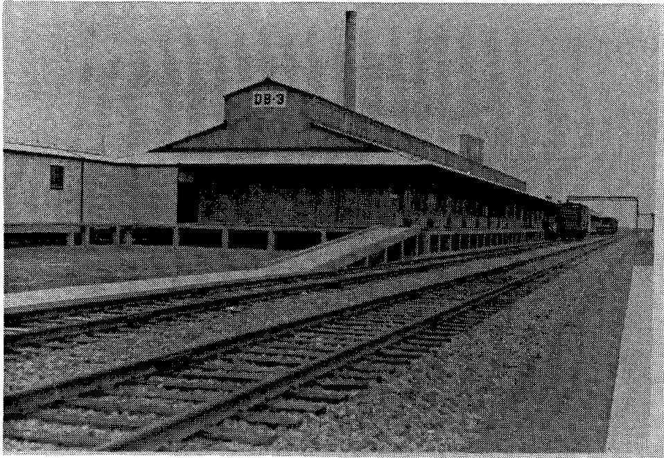
Plate 13. Ca. 1942 photograph of Receiving and Painting Building BD-WP-3A in Load Line II, completed November 3, 1941. Photograph shows the ramps and adjacent railroad line used for transporting and shipping (U.S. Government n.d.).
