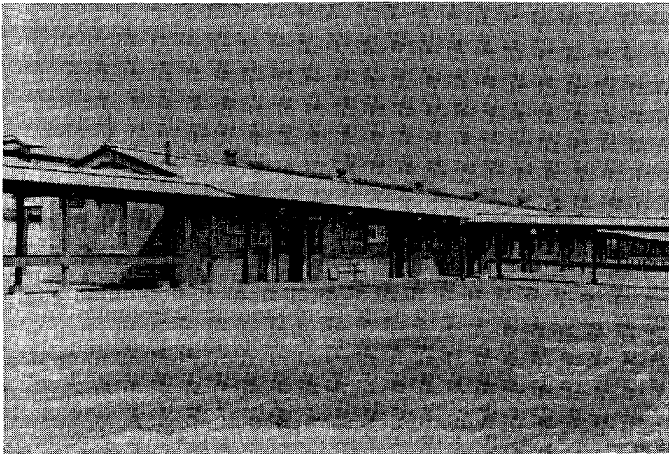
Plate 14. Ca. 1942 photograph of Teteryl Pelleting Building 1B-WP44, Booster Line #1, Fuze and Booster Area, completed March 15, 1942. The plate illustrates the extensive covered walkway system in the Fuze and Booster area (U.S. Government n.d.).
