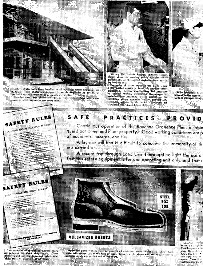
Plate 29. ROP Magazine from November 1941 which shows some of the safety measures instigated throughout the Ravenna Ordnance Plant (ROP, article k, Volume I, No. 5).
