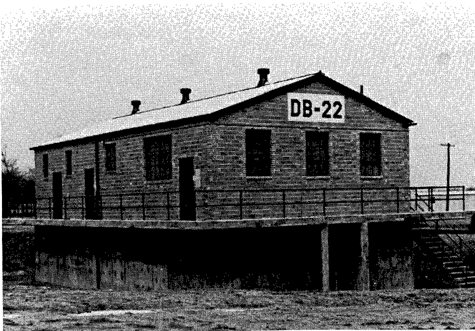
Plate 6. Ca. 1942 photograph of Change House DB-WP-22 in Load Line II, completed November 3, 1941 (U.S. Government n.d.).
