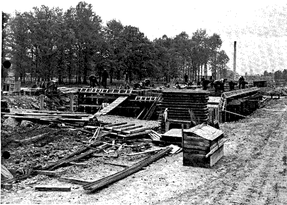
Plate 18. Hunkin-Conkey Construction Company photograph from June 1, 1942, shows the construction of Building 904 in the Ammonium Nitrate Line. The plate illustrates the large number of construction personnel who worked on one building at the same time (Hunkin-Conkey Construction Company n.d.).
