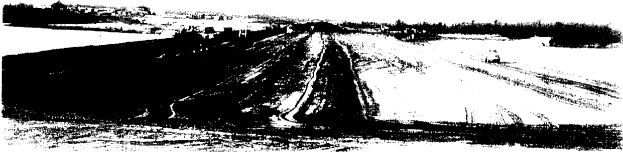
29. Construction of the closure dam.
