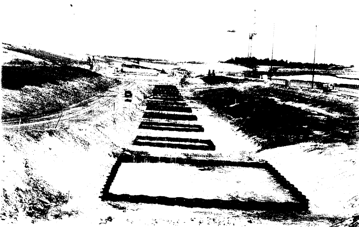
28. Sheet pile encapsulated footing for the downstream guidewall.
