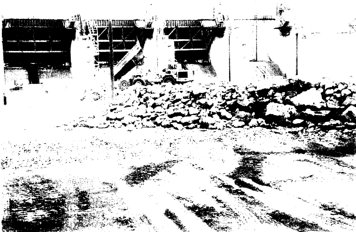
15. Placing riprap in the downstream channel.
