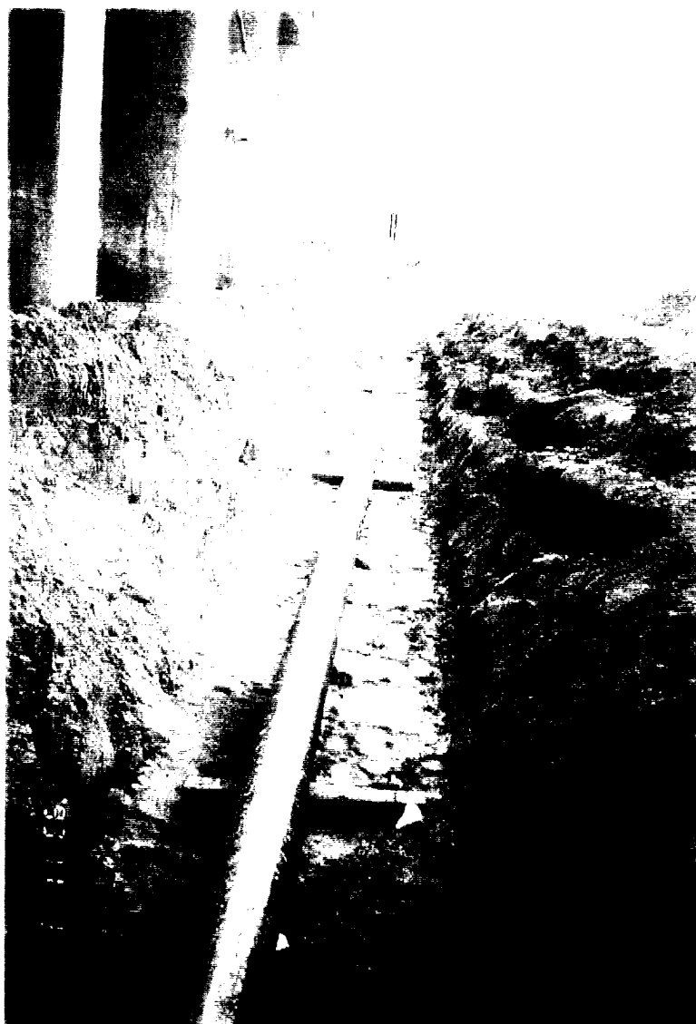
8. Installation of stainless steel collector pipe well screen in backfill landside of lock.
