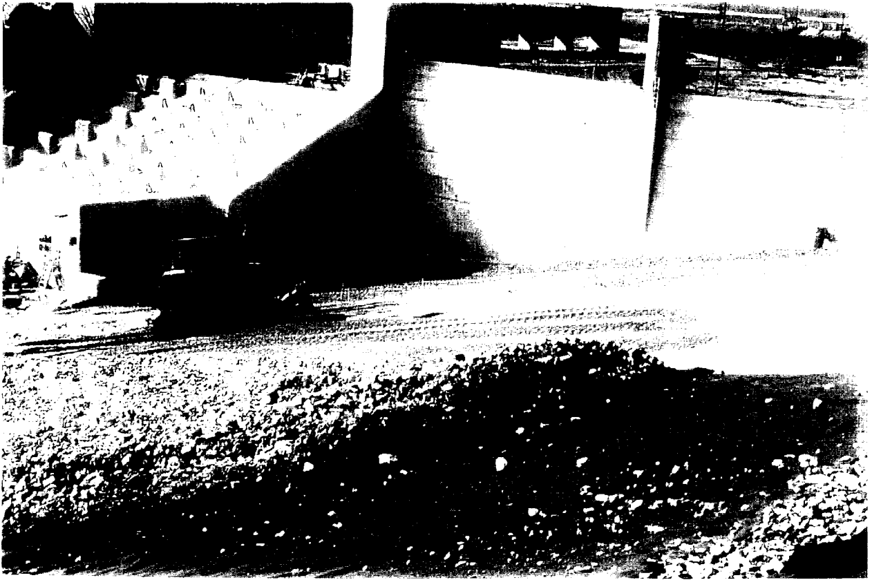
23. Placing pervious backfill downstream of the overflow wall.
