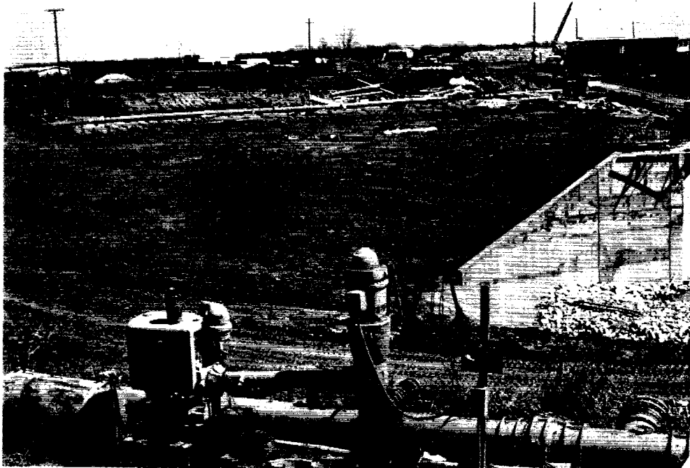
11. DEWATERING WELL #6, NOTE PRIMARY (ELECTRIC) AND BACKUP (DIESEL)
