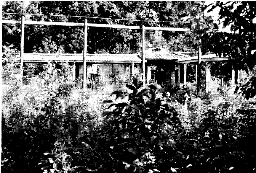
Figure 187. Building PE-14: Metal Parts Loading Building.
