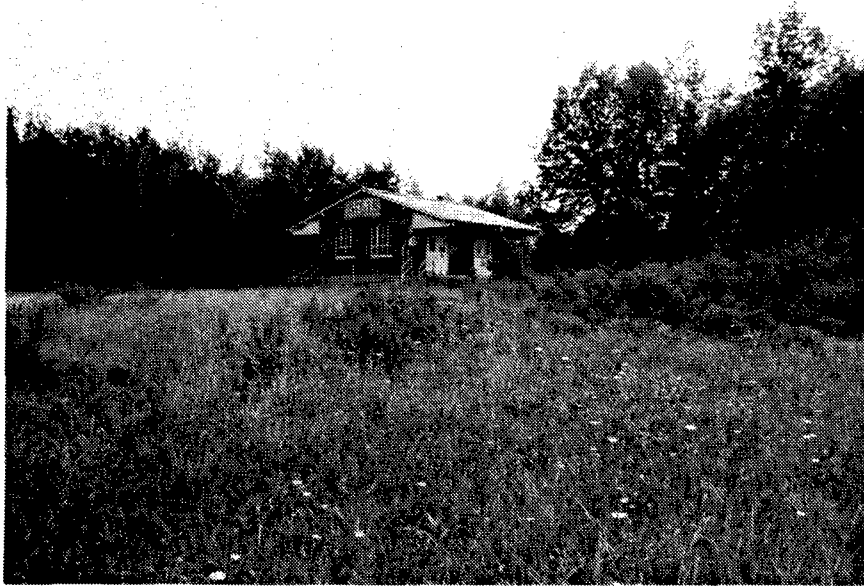
Figure 256. Building AP-16: Ready Magazine.
