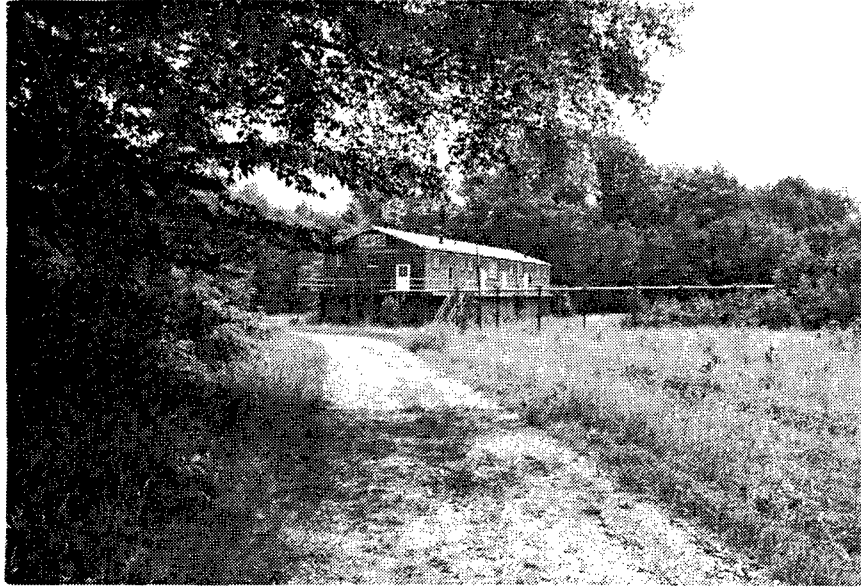
Figure 288. Building CA-15: Change House.
