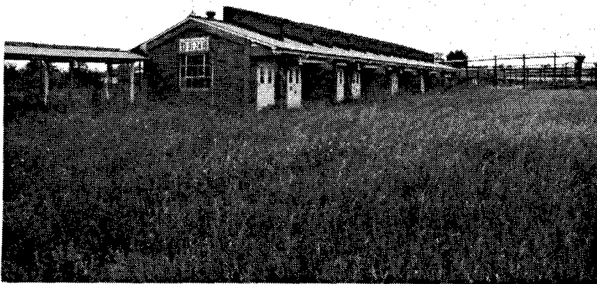
Figure 154. Building DT-24: Another view of this Metal Parts Loading Building.
