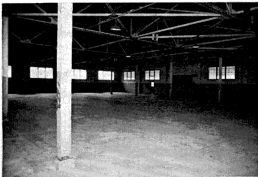
Figure 223. Building CB-801: Interior view of this Inert Storage Warehouse.
