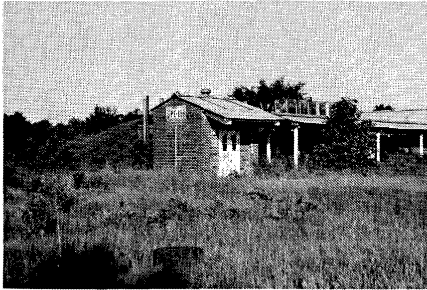
Figure 272. Building PE-11: Ready Magazine.
