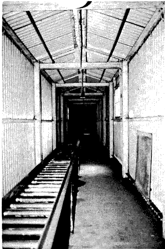
Figure 35. Corridor between H.E. Preparation Building (Building CA-6A) and Ammonium Nitrate Building (Building CA-5).
