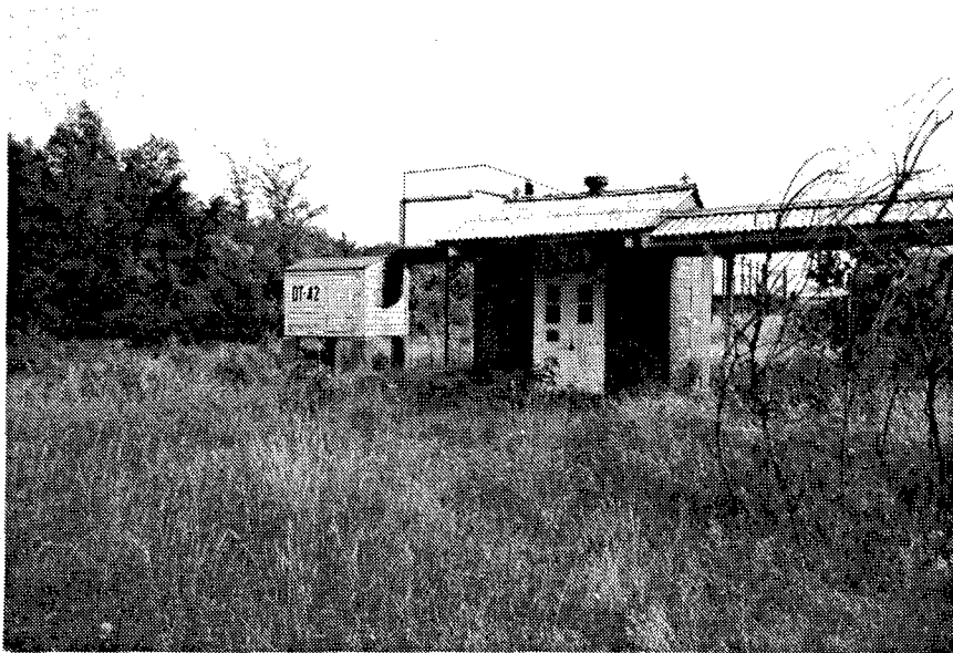
Figure 160. Building DT-42: Metal Parts Loading Building with a view of a Ready Magazine (Building DT-25).
