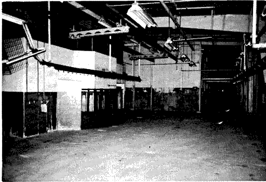
Figure 71. Building G-13A: Interior view of this Top Pour Building.
