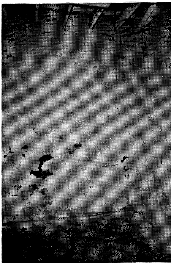
Figure 267. Building DT-27: Interior of this Ready Magazine.
