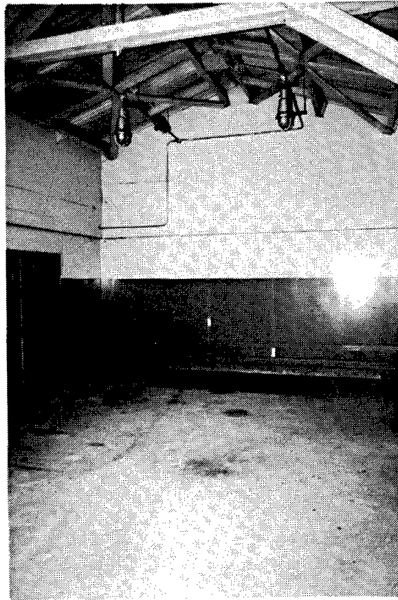
Figure 59. Building G-16: Interior view of this TNT Service Building.
