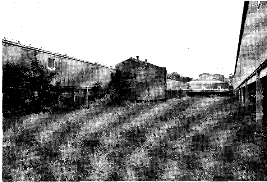
Figure 261. Building CA-16: Ready Magazine.
