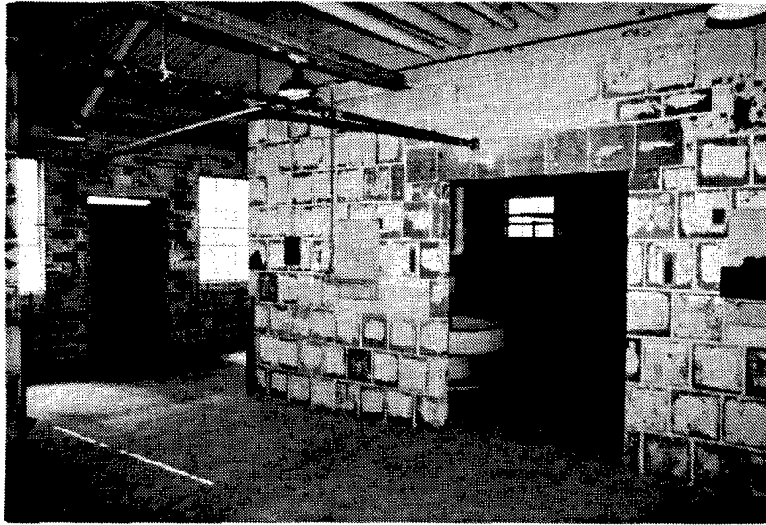
Figure 302. Building 2F-36: Interior view of this Change House.
