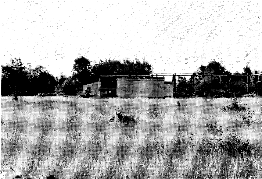
Figure 134. Building DT-8: Metal Parts Loading Building.
