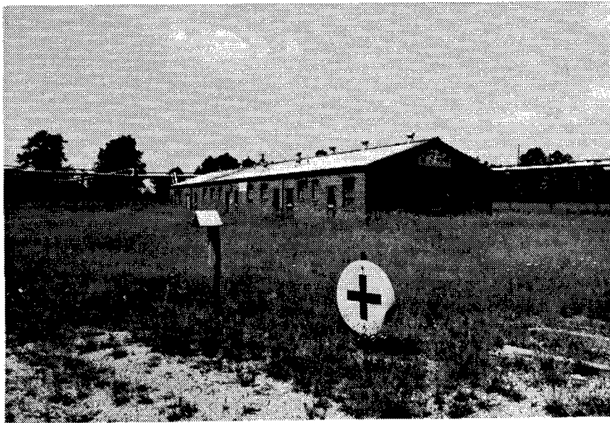
Figure 300. Building 2F-14: Change House.
