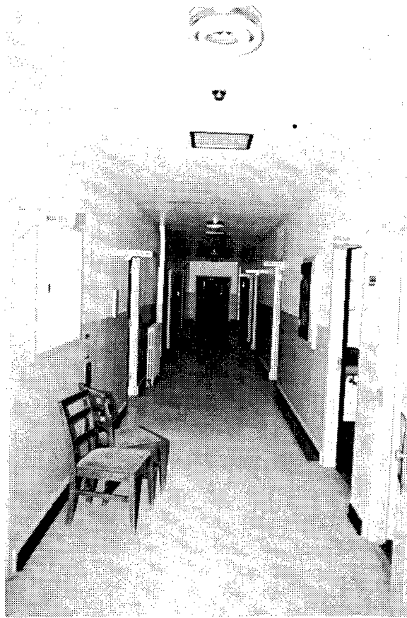
Figure 317. Building 1031: Interior view of the Hospital.
