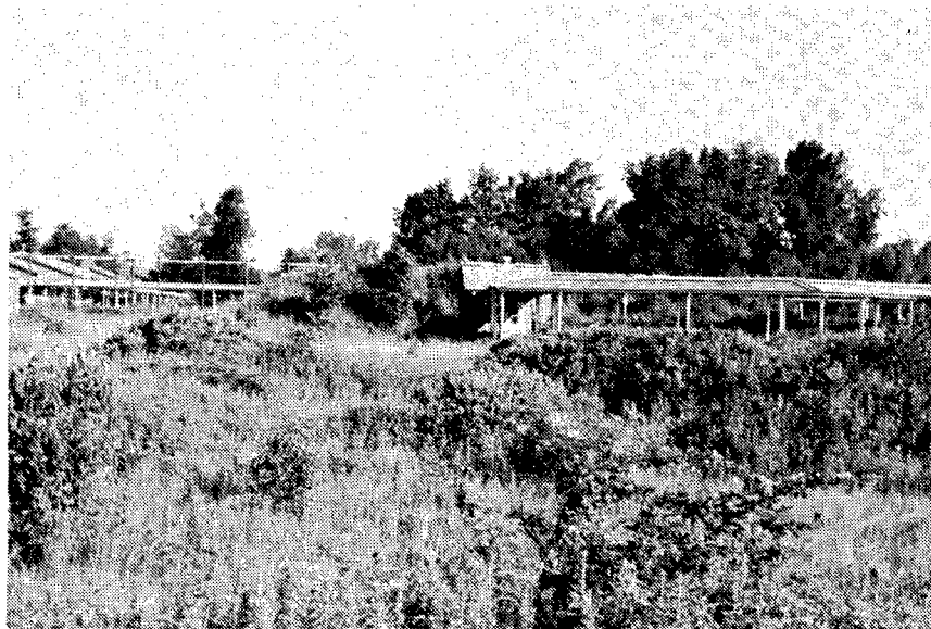
Figure 277. Building PE-19: Ready Magazine.
