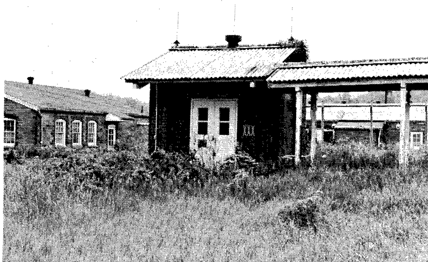
Figure 257. Building AP-17: Ready Magazine.
