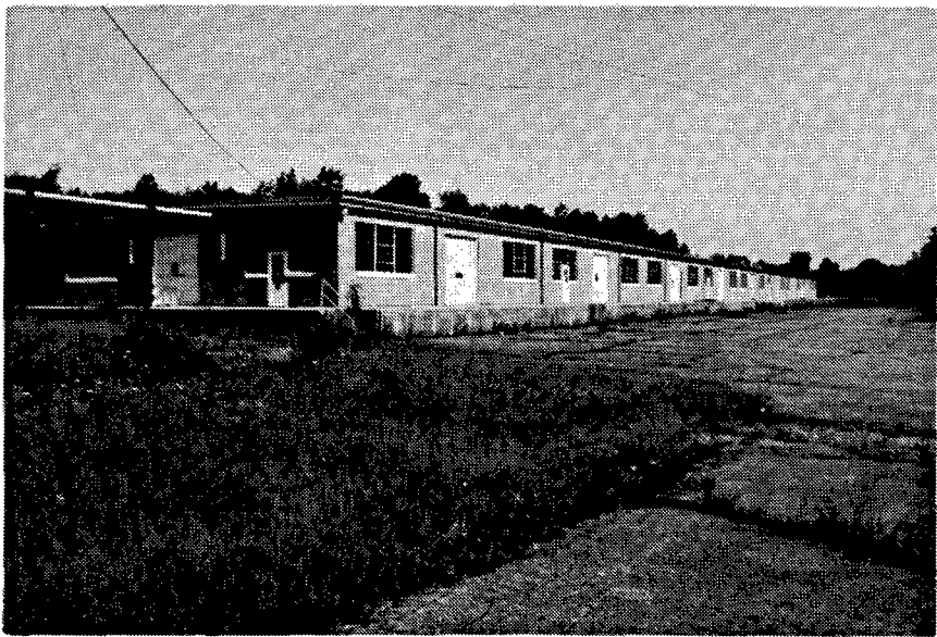
Figure 284. Building U-14: Dunnage Building.
