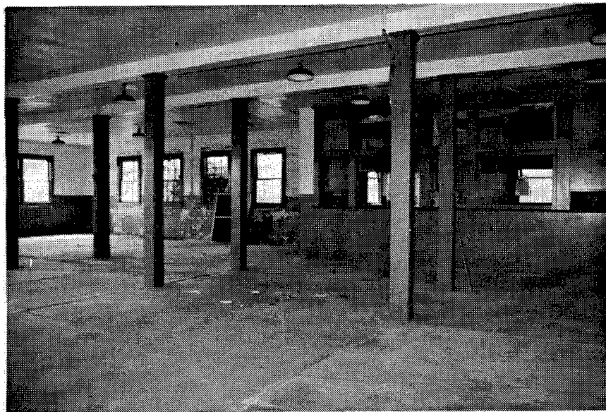
Figure 169. Building DT-52: Interior view of this building.
