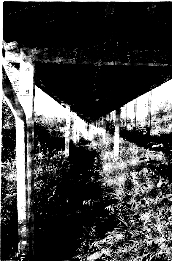
Figure 170. Building DT-54: Metal Parts Loading Building.
