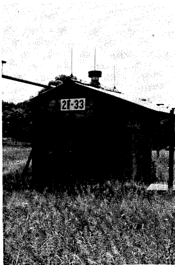
Figure 246. Building 2F-33: Pellet Storage Building.
