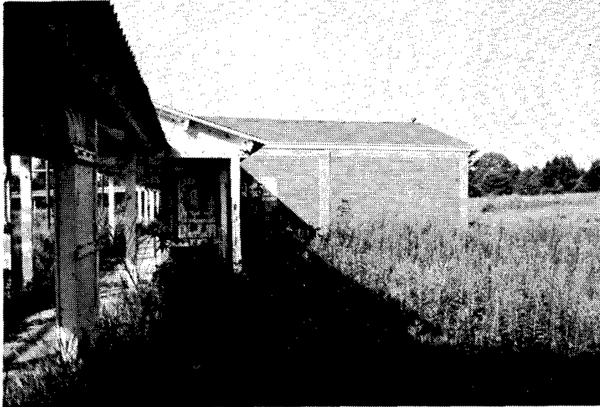
Figure 175. Building PE-5: Metal Parts Loading Building.
