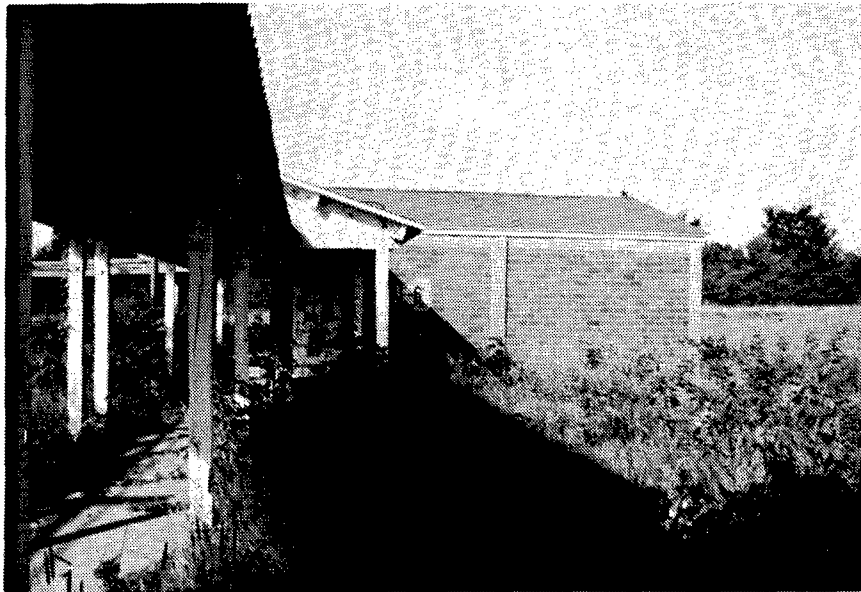
Figure 177. Building PE-6: Metal Parts Loading Building.
