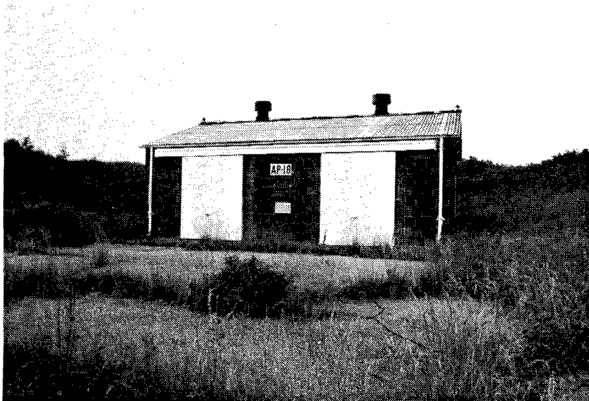
Figure 259. Building AP-18: Ready Magazine.
