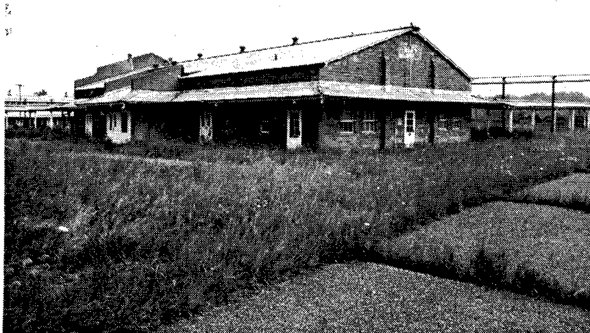
Figure 114. Building AP-8: Metal Parts Loading Building.
