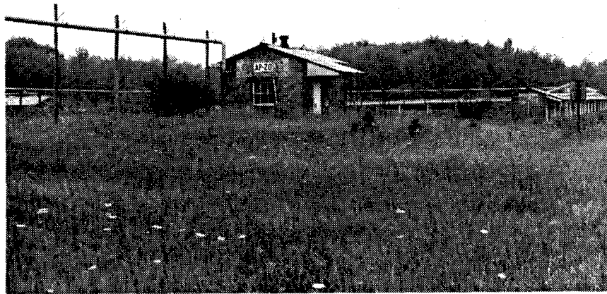
Figure 120. Building AP-20: Metal Parts Loading Building.
