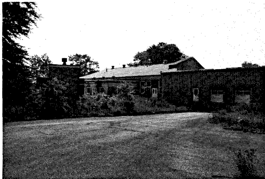
Figure 72. Building G-13A: Top Pour Building.
