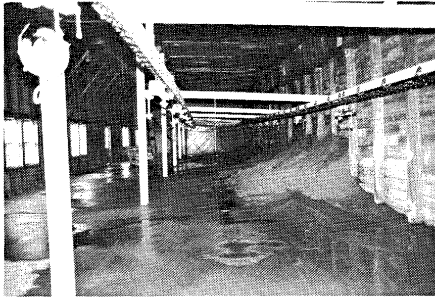
Figure 206. Building G-1A: Interior view of the Truck Repair Shop.
