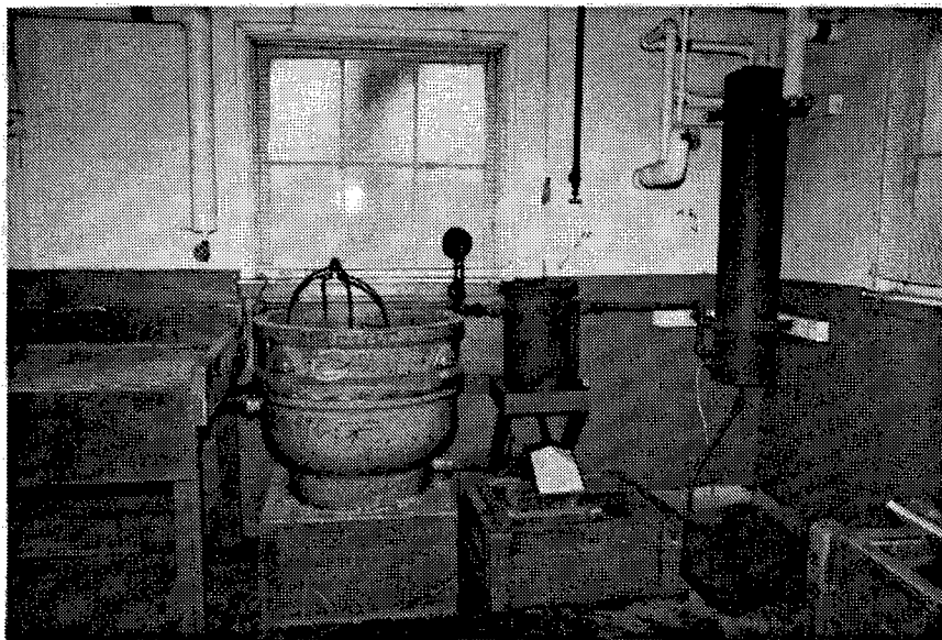
Figure 197. Building PE-30: Interior view of this building.
