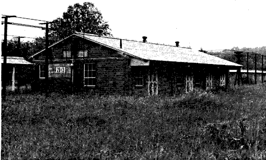
Figure 101. Building 2B-13: Tetryl Cupping Building.
