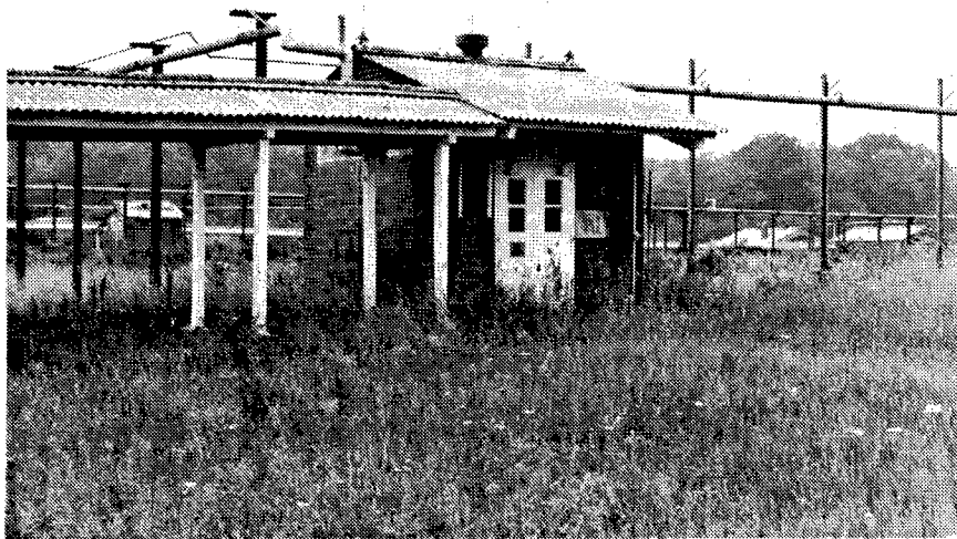
Figure 254. Building AP-10: Ready Magazine.
