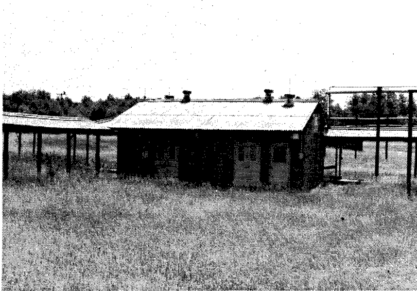
Figure 87. Building 2F-9: Primer Dry House.
