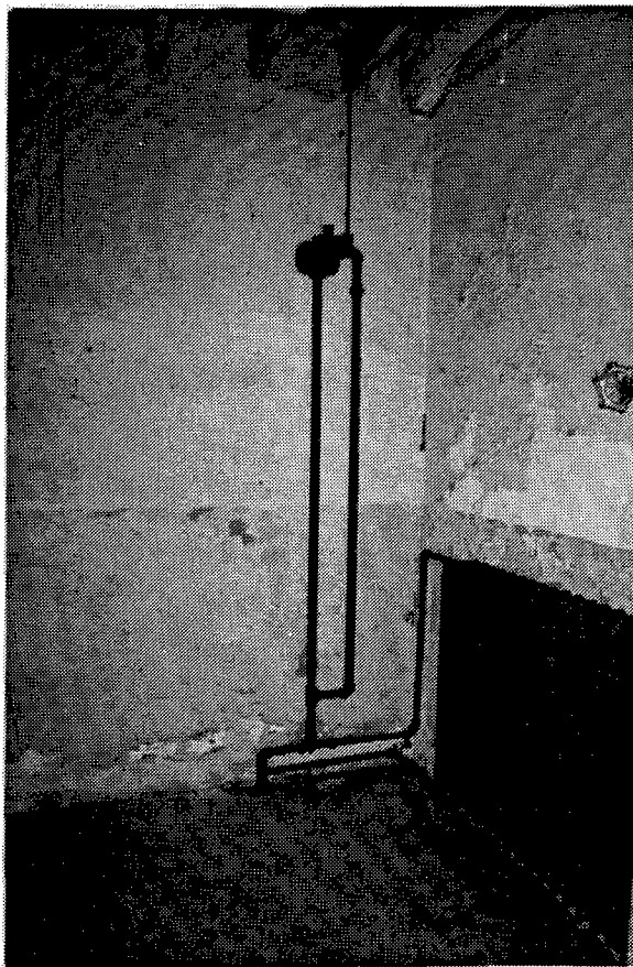
Figure 145. Building DT-15: Interior view of this building.
