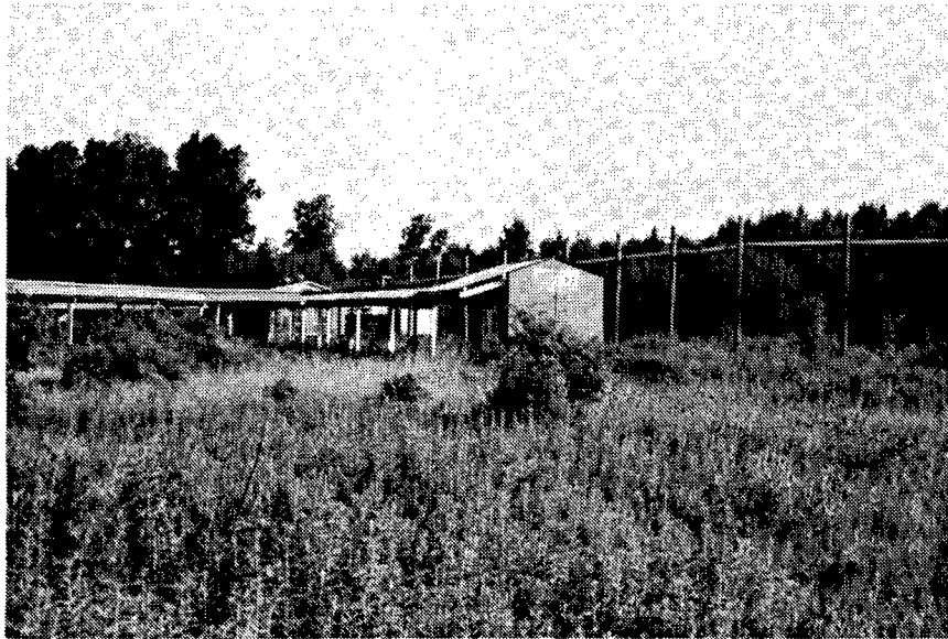
Figure 274. Building PE-17: Ready Magazine.
