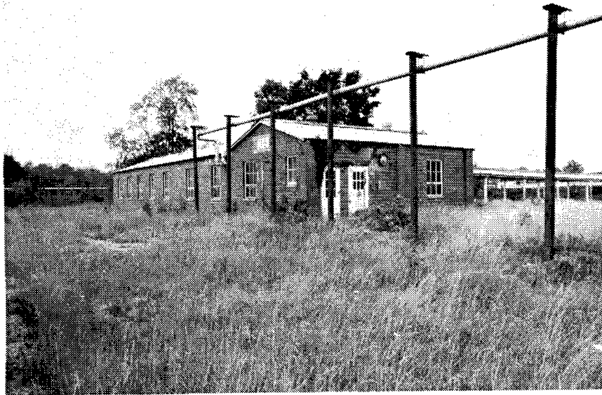
Figure 148. Building DT-18: Metal Parts Loading Building.
