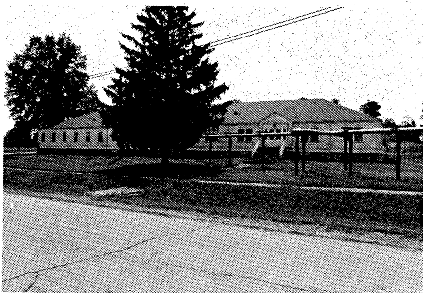
Figure 4. Building 1038: Office and Guard House recently used as a Civilian Persons Building.
