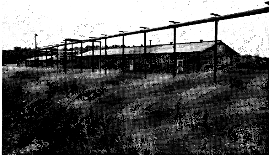
Figure 292. Building DT-29: Change House.
