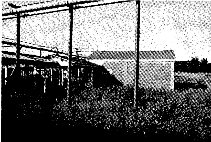
Figure 173. Building PE-4: Metal Parts Loading Building.
