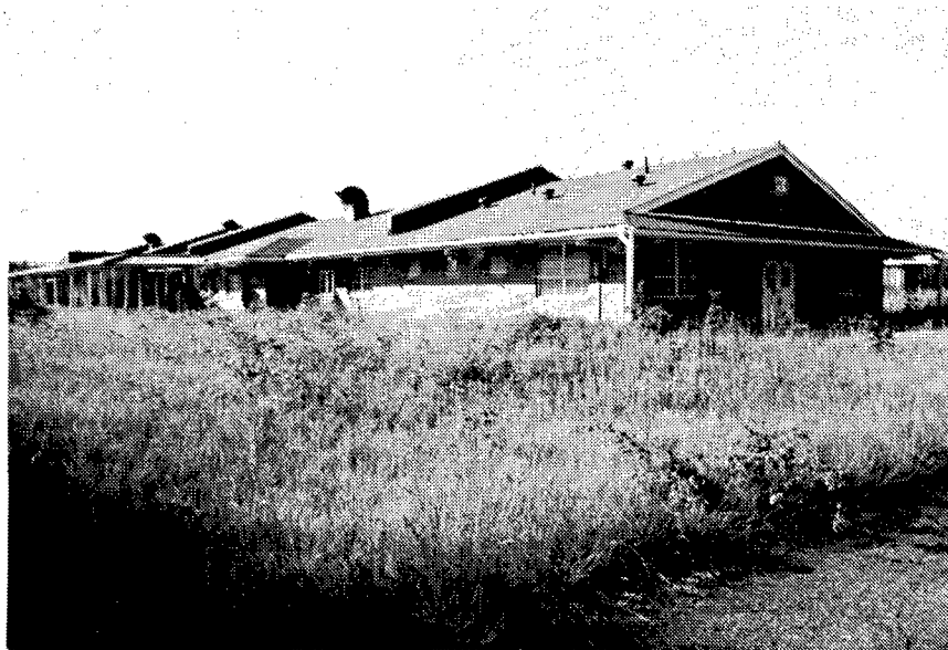
Figure 171. Building PE-1: Metal Parts Loading Building.
