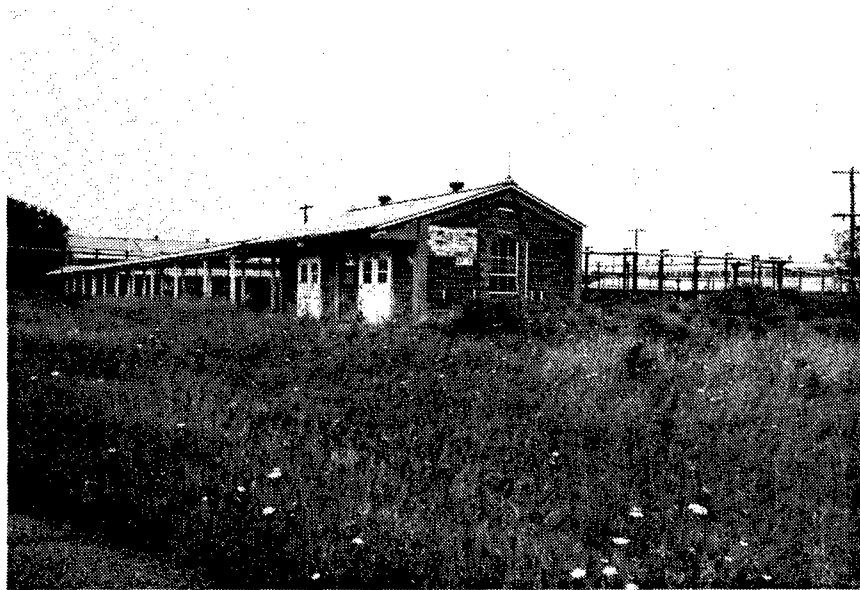
Figure 116. Building AP-9: Metal Parts Loading Building.
