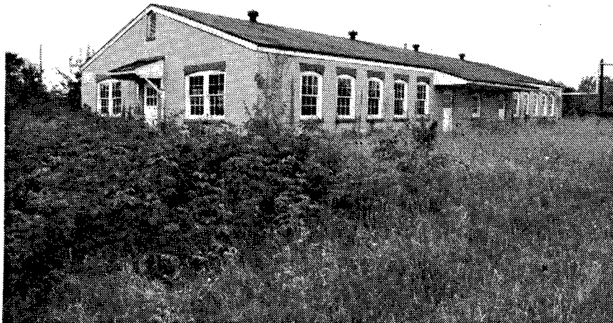
Figure 168. Building DT-52: Metal Parts Loading Building.
