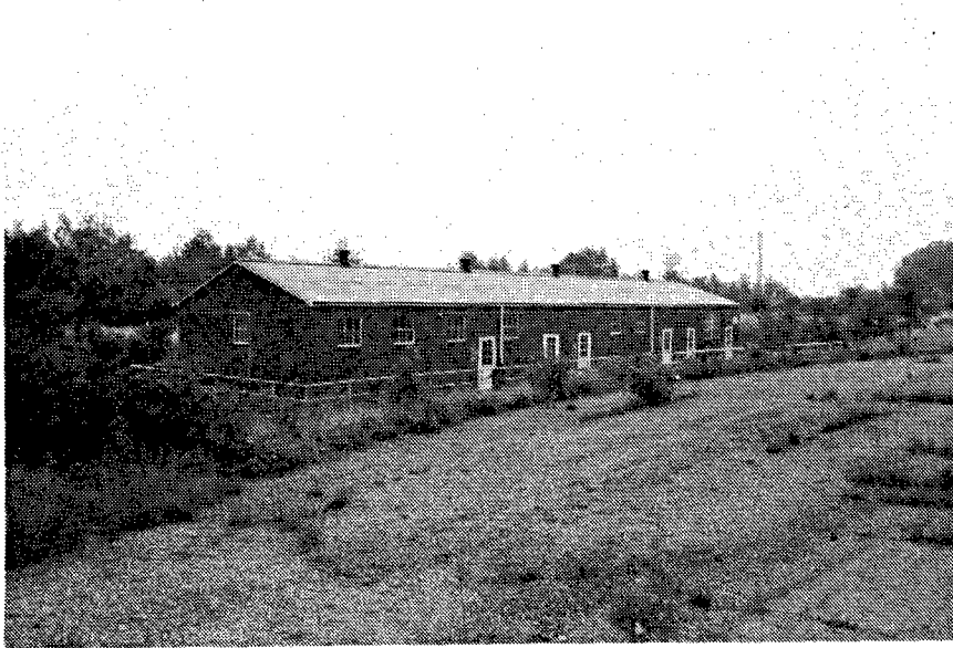
Figure 290. Building CB-8: Change House.
