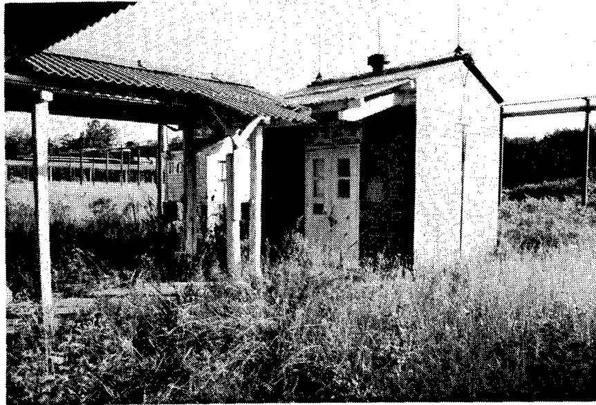
Figure 161. Building DT-43 and Building DT-4: Metal Parts Loading Buildings.
