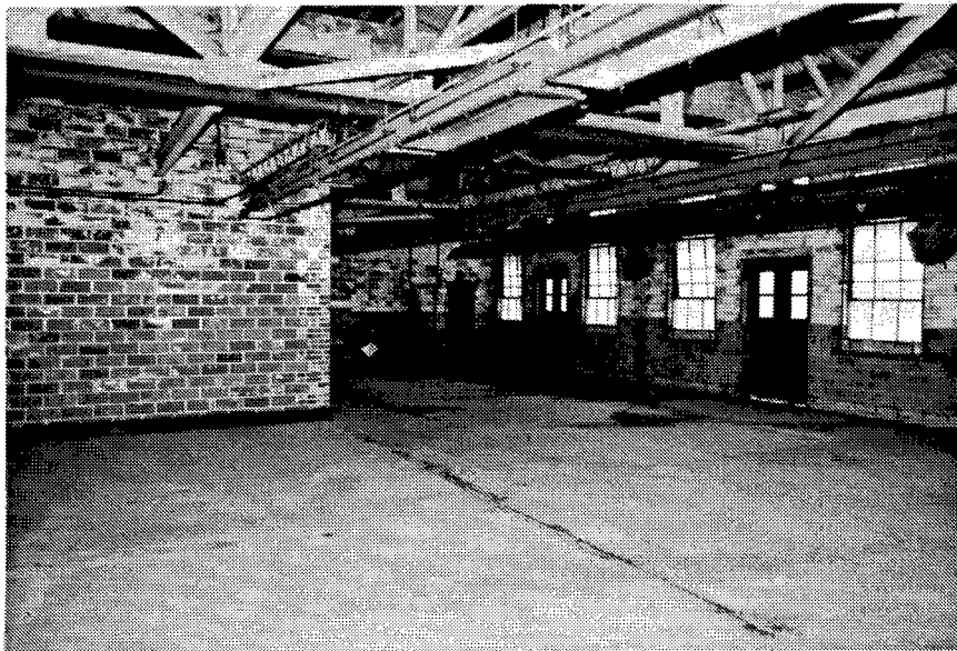
Figure 82. Building 2F-4: Interior view of this Primer Loading Building.
