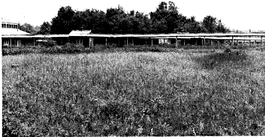
Figure 103. Building 2B-17: Cupped Pellet Rest House. Photograph also includes a Detonator Magazine (Building 2B-5) and a Small Heater House (Building 2B-24).
