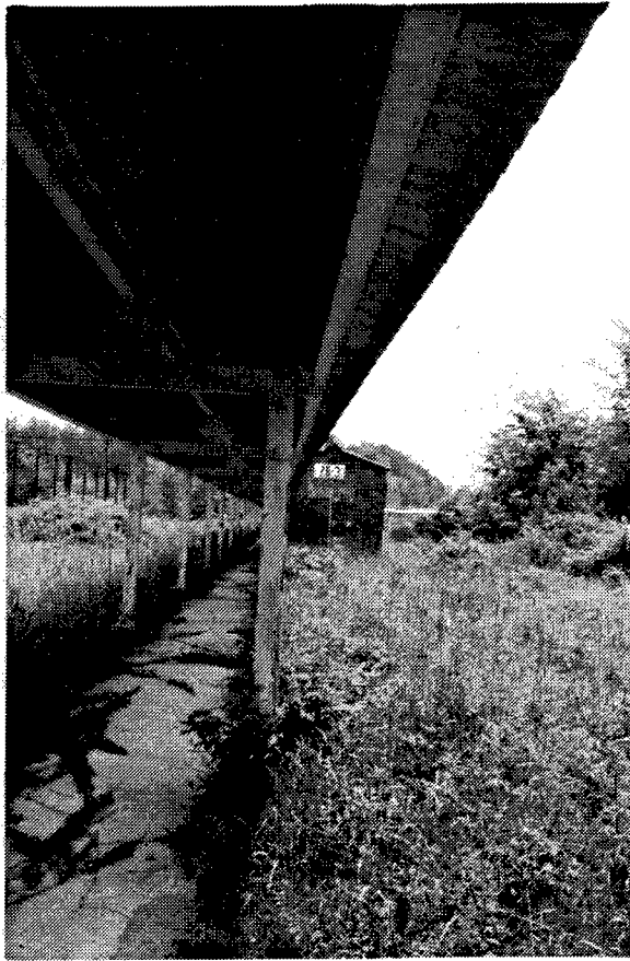
Figure 97. Building 2B-3: Blended Tetryl Rest House.
