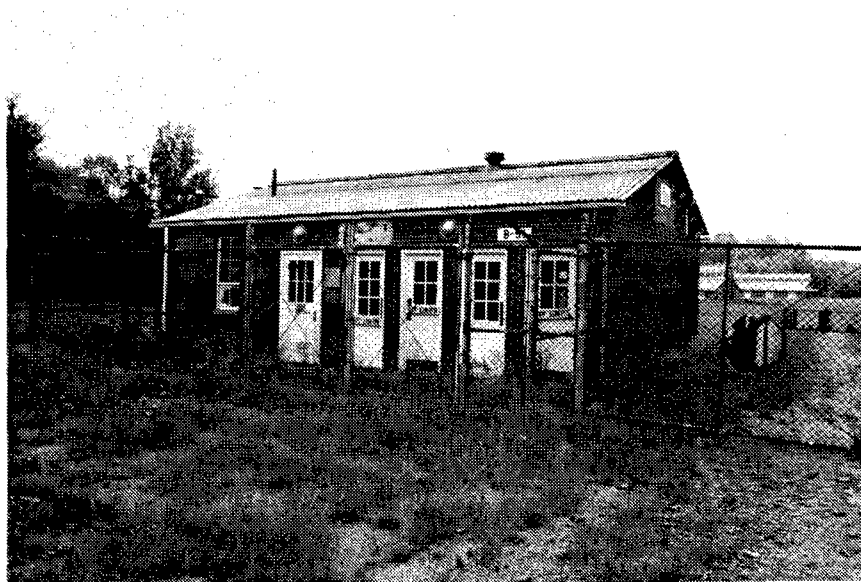
Figure 305. Building 8-51: Time Clock Alley with covered walks.
