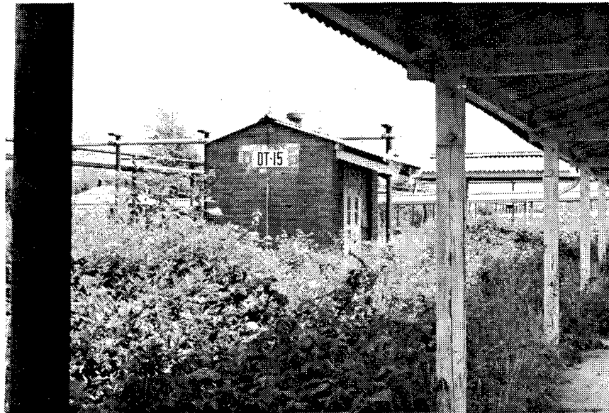
Figure 144. Building DT-15: Metal Parts Loading Building.
