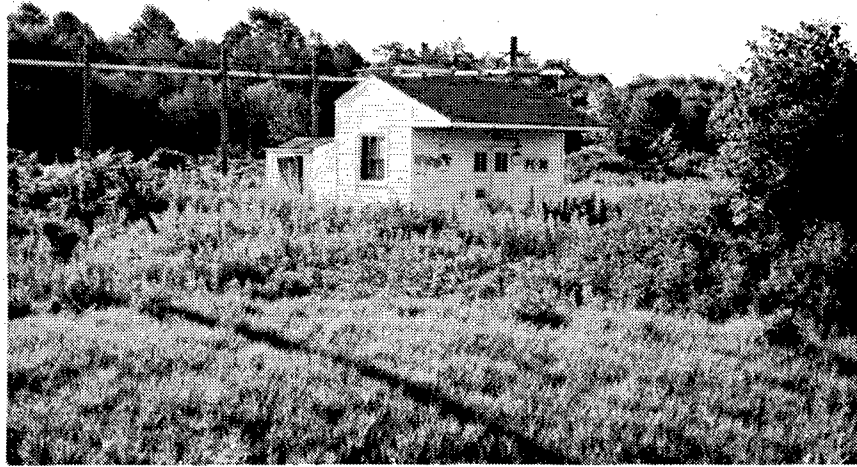
Figure 196. Building PE-30: Metal Parts Loading Building.
