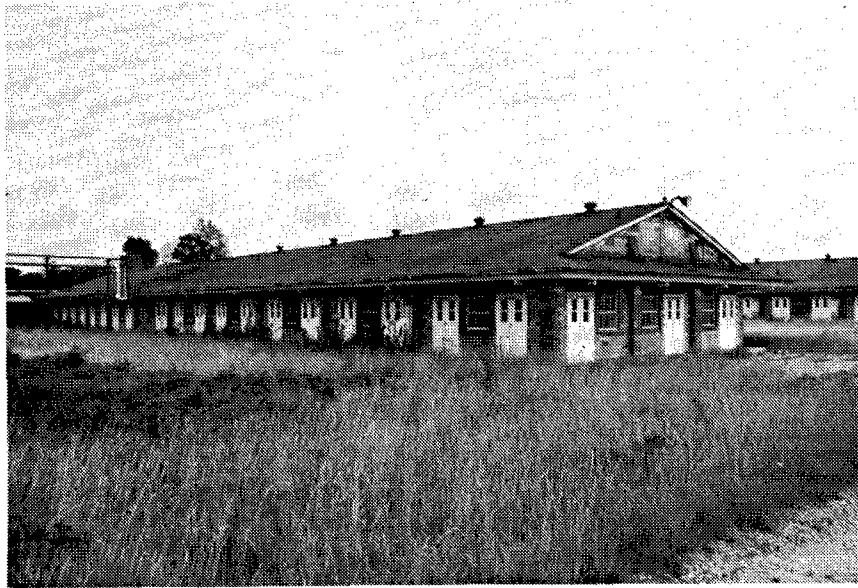
Figure 157. Building DT-26: Metal Parts Loading Building.
