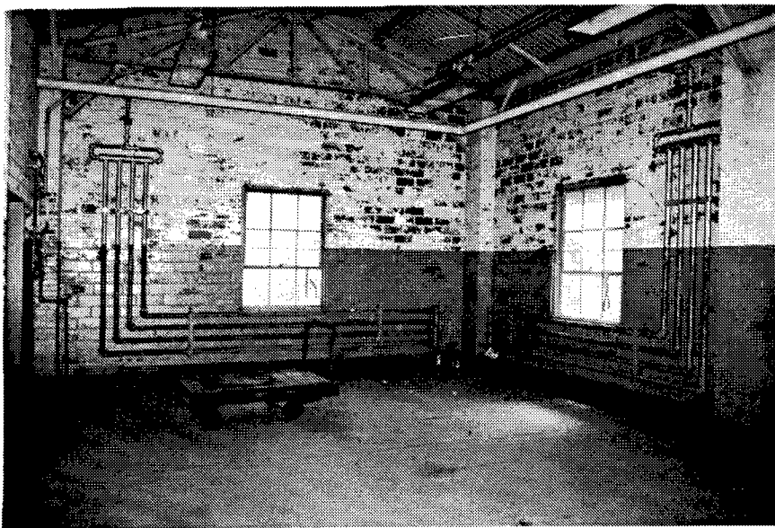
Figure 44. Building CA-21: Interior view of the TNT Box Building.
