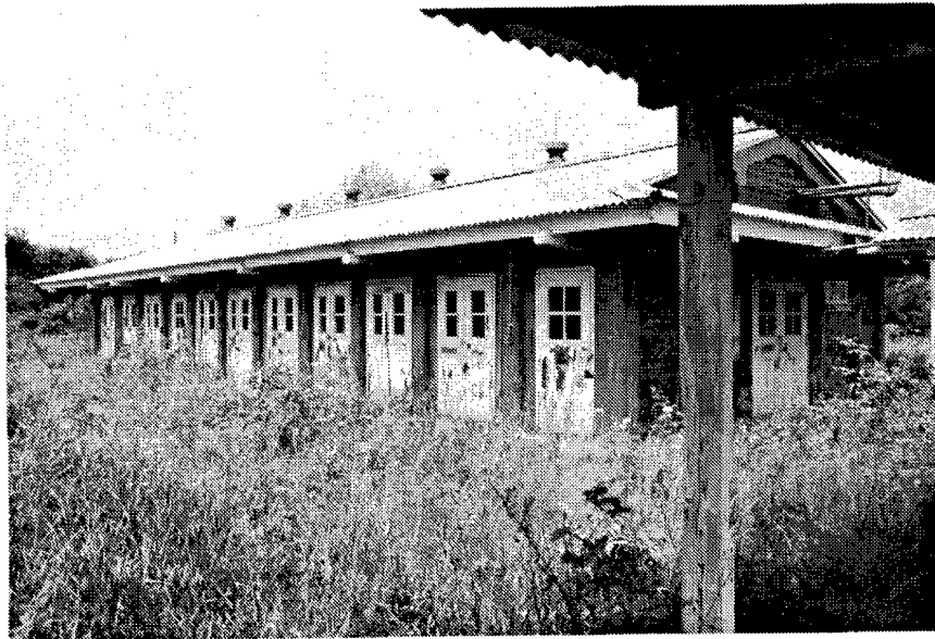
Figure 142. Building DT-14: Metal Parts Loading Building.
