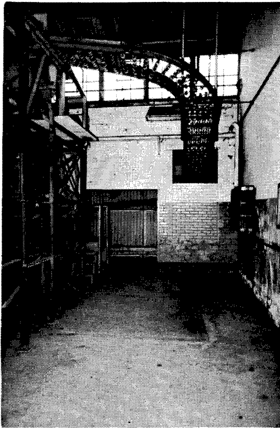
Figure 34. Building CA-6: Interior view of the H.E. Preparation Building.
