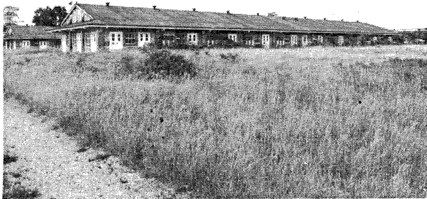
Figure 150. Building DT-21: Metal Parts Loading Building.
