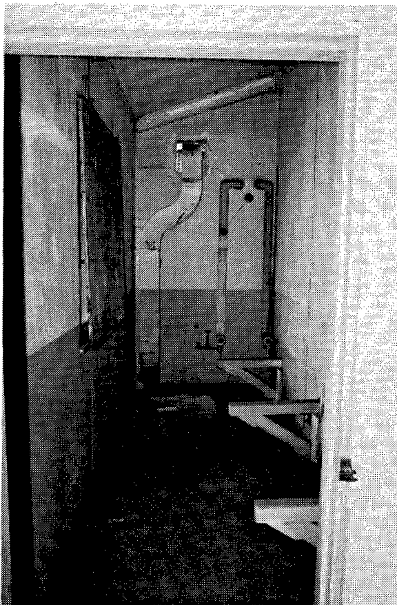
Figure 128. Building DT-3: Interior view of this building.
