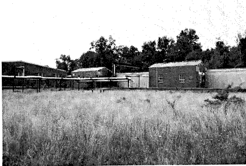
Figure 203. Building CB-19 (left) and Building CB-2 (right): Electric Locomotive Service Building (left) and a Paint and Oil Storage Building.
