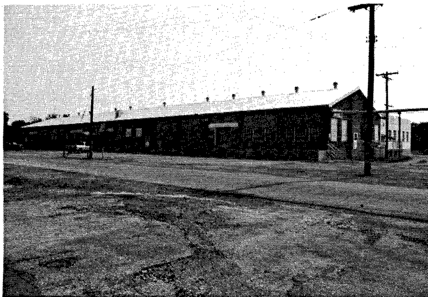
Figure 3. Building 1035: Administration General Purpose Building.
