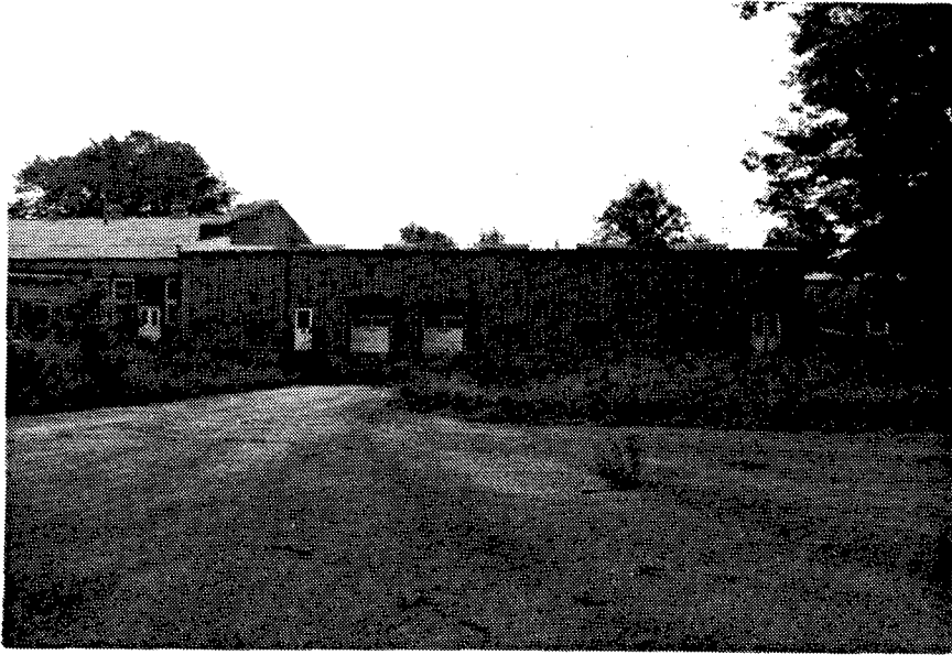
Figure 69. Building G-13: Top Pour Building located in Load Line #4, a part of the Major Caliber Loading Plant.
