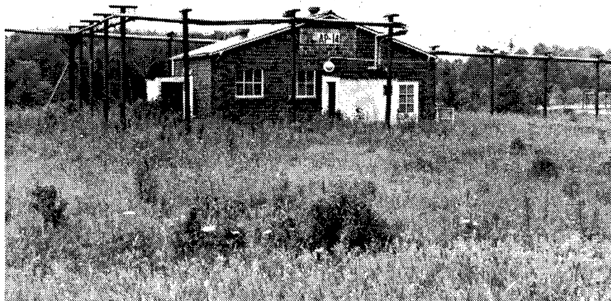
Figure 286. Building AP-14: Change House.
