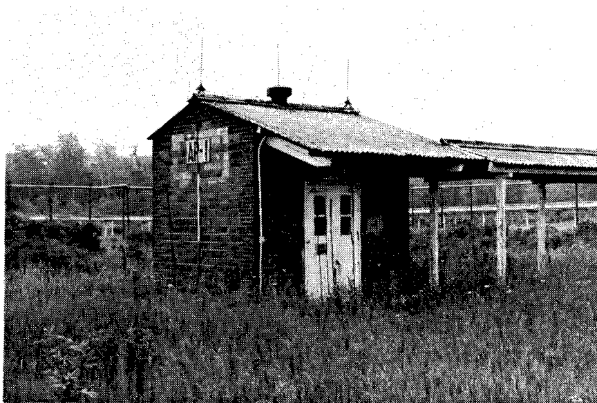
Figure 250. Building AP-1: Ready Magazine.
