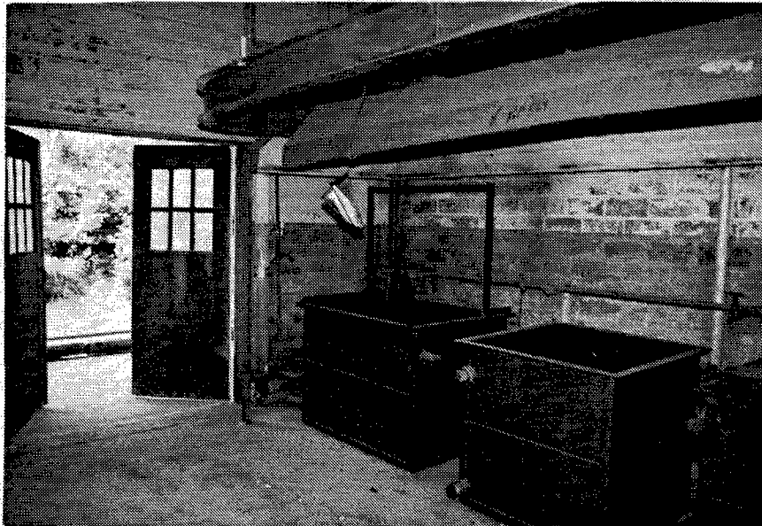
Figure 234. Building CB-2: Paint Spray Unit in the Paint and Oil Storage Building.
