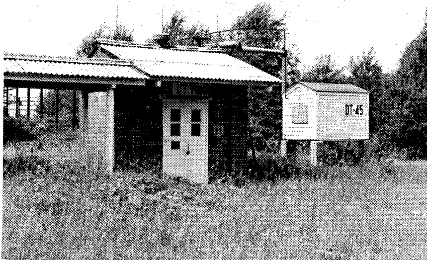
Figure 163. Building DT-45: Metal Parts Loading Building with a view of a Ready Magazine (Building DT-10).
