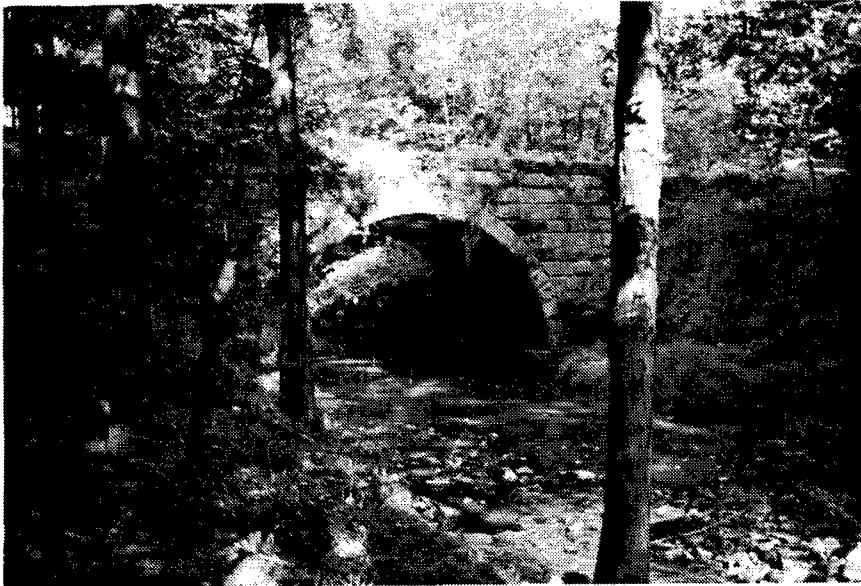
Figure 321. Wadsworth Road Bridge. This stone arch bridge spans the South Fork of Eagle Creek on Wadsworth Road and is located south of the northern boundary of Ravenna Army Ammunition Plant.
