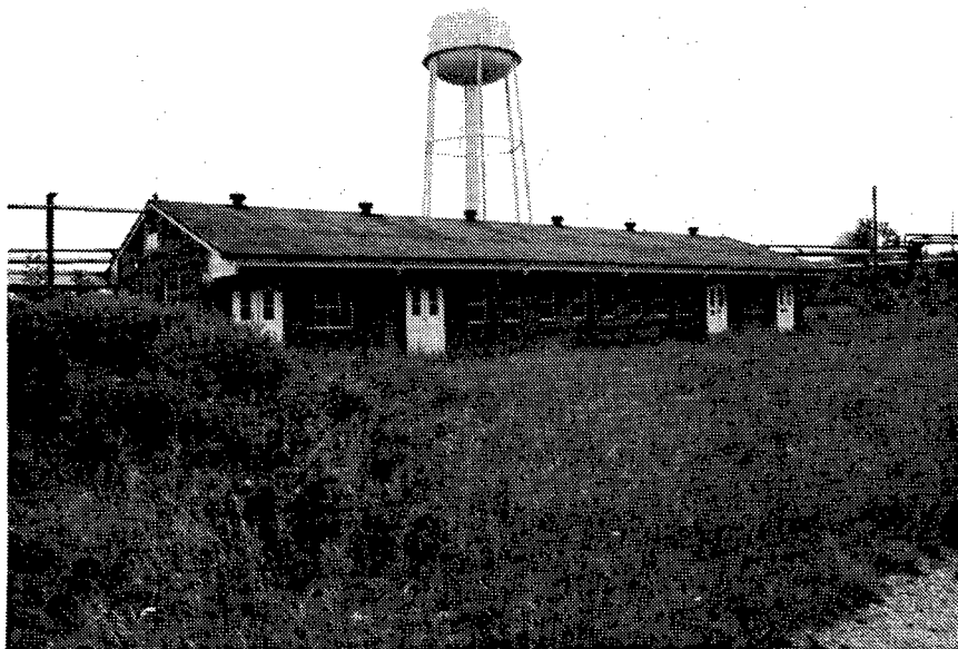
Figure 140. Building DT-13: Metal Parts Loading Building.
