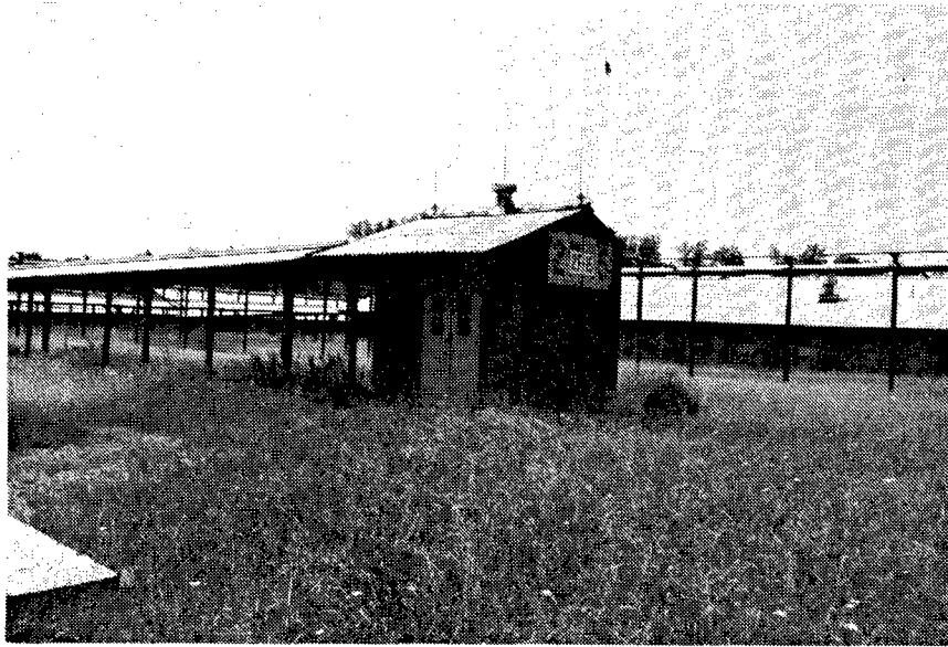
Figure 243. Building 2F-15: Paint Storage Building.
