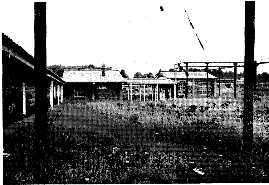
Figure 112. Building AP-5 and Building AP-6: Metal Parts Loading Buildings.
