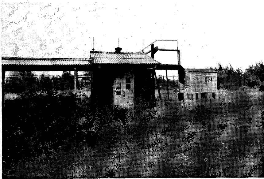
Figure 123. Building DT-1 and Building DT-41: Metal Parts Loading Buildings.
