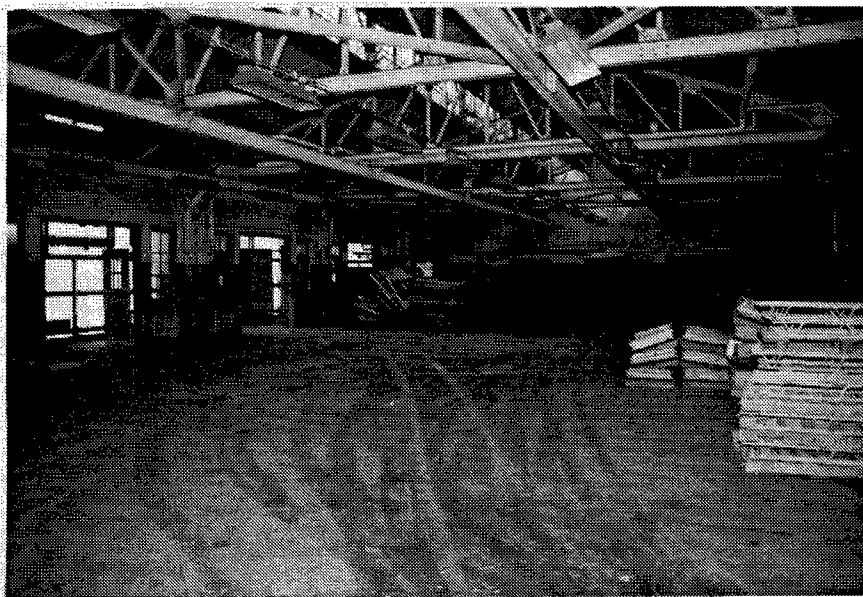
Figure 43. Building CA-17: Interior view of this Smokeless Powder Building.
