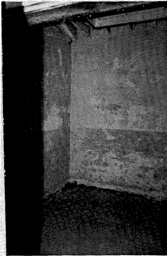
Figure 265. Building DT-23: Interior view of a Ready Magazine.
