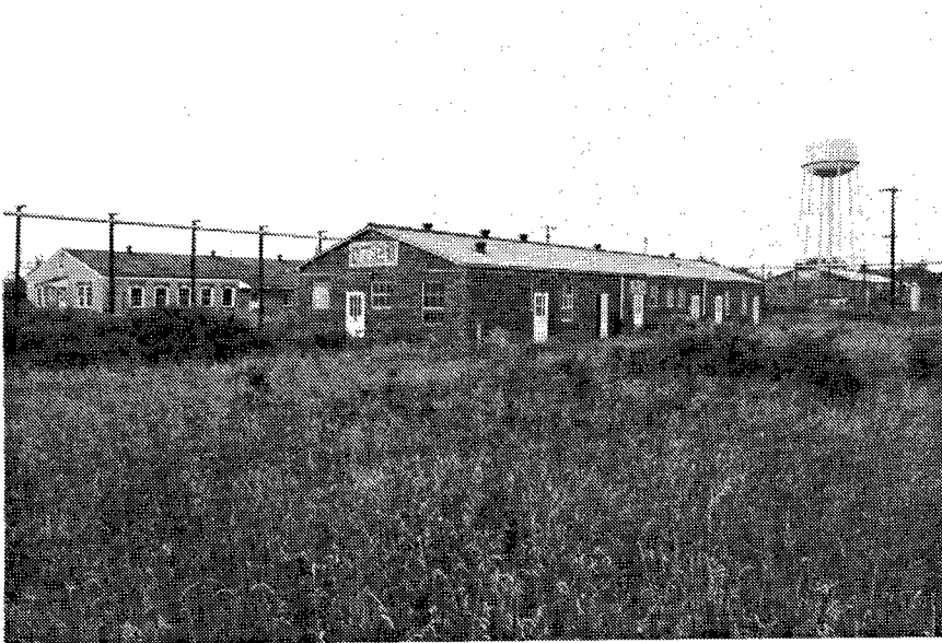
Figure 291. Building DT-28: Change House.
