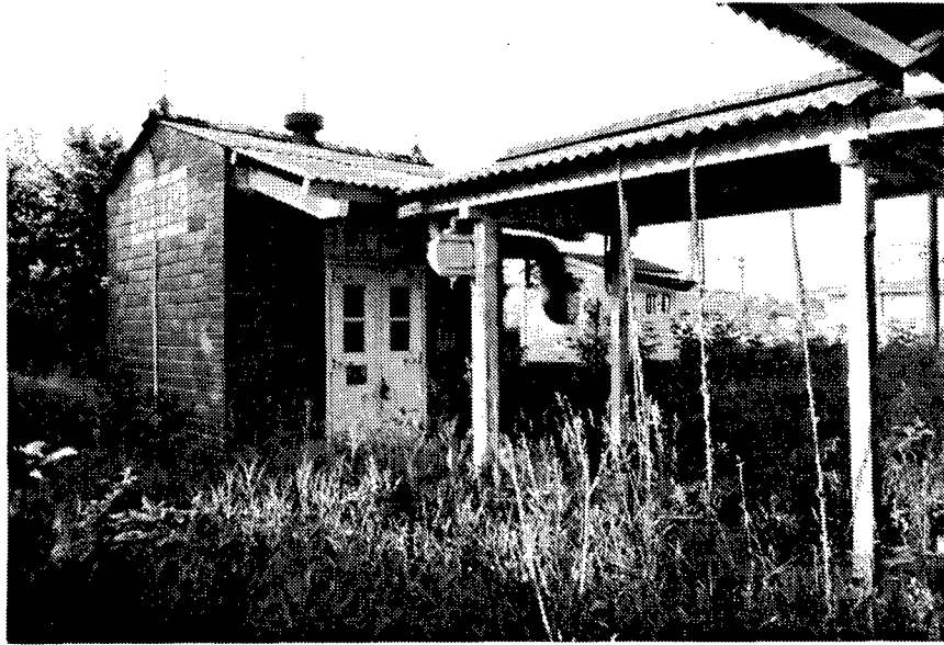
Figure 165. Building DT-47: Metal Parts Loading Building with a view of a Ready Magazine (Building DT-19).
