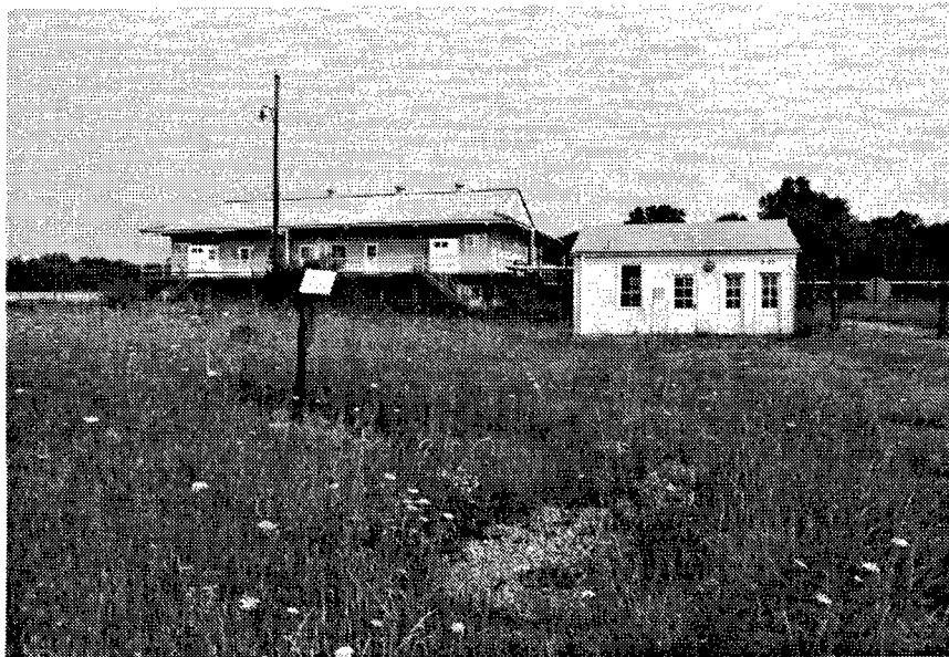
Figure 296. Building G-6 and Building G-20: Change House and Time Clock Alley, respectively.
