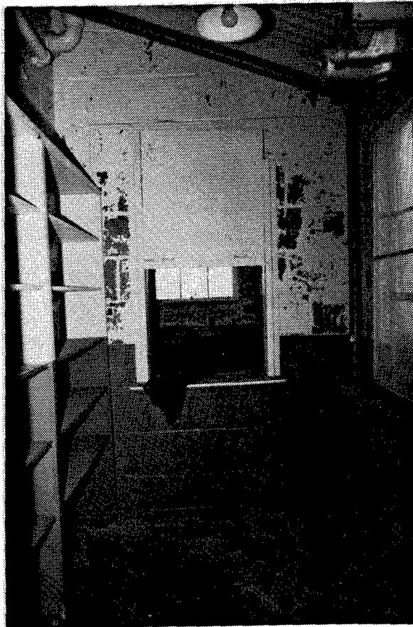
Figure 287. Building AP-14: Interior view of this Change House.
