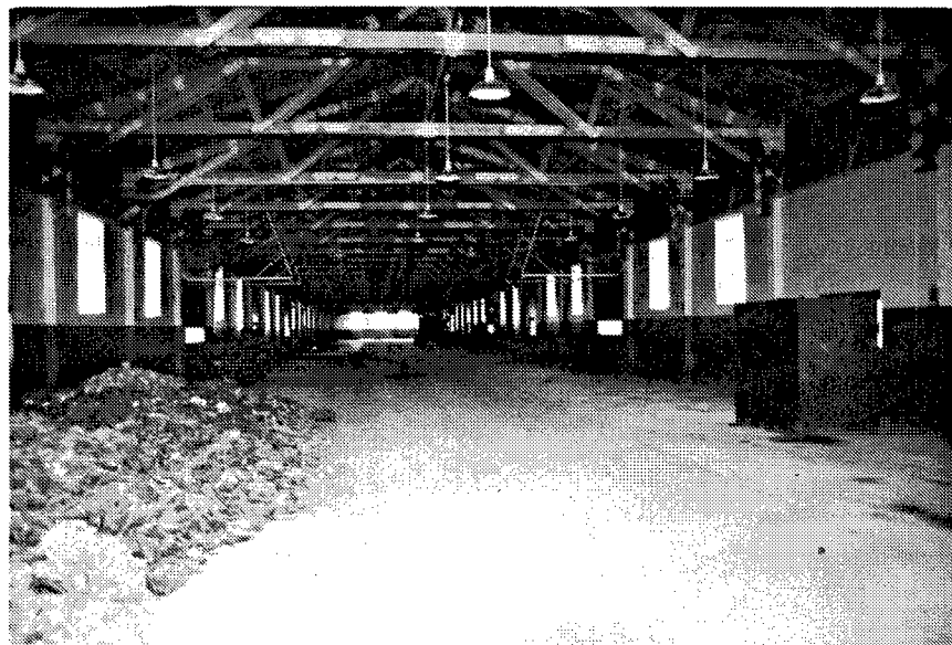
Figure 207. Building G-1A: Another interior view of the Truck Repair Shop.
