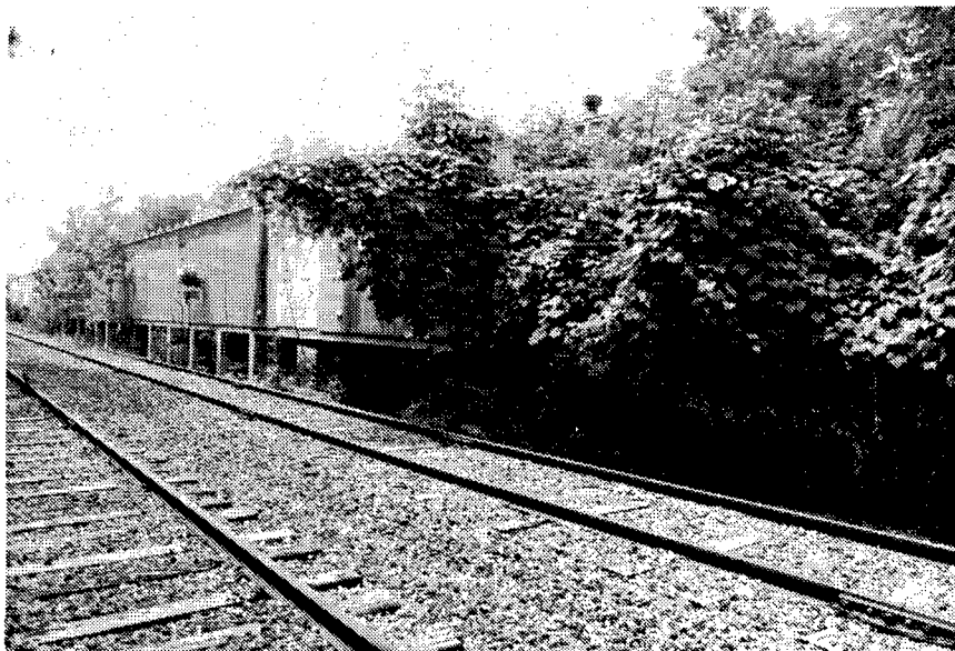
Figure 260. Building CA-7: Ready Magazine.
