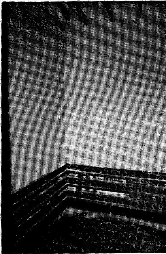
Figure 273. Building PE-11: Interior view of this Ready Magazine.
