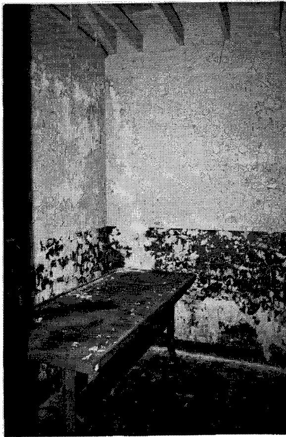
Figure 278. Building PE-19: Interior view of this Ready Magazine.
