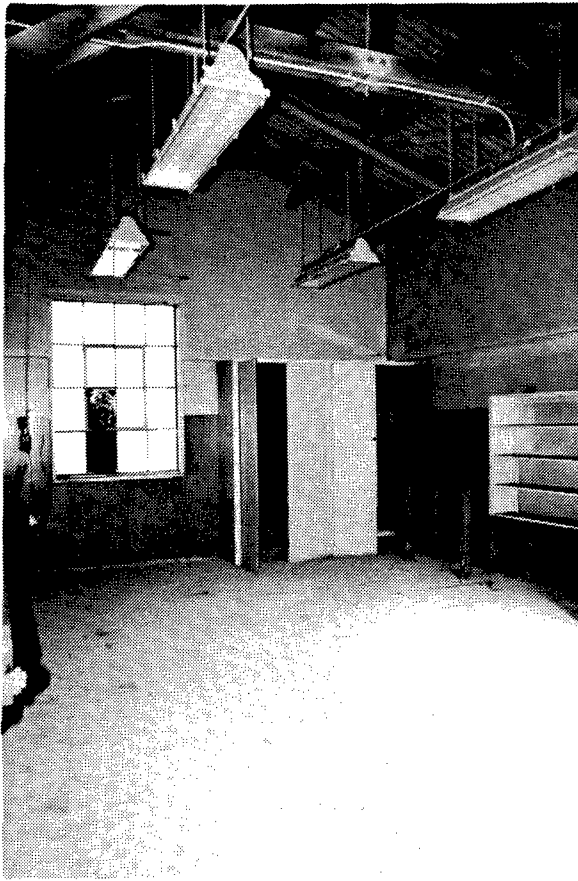
Figure 48. Building G-7: Interior view of this Booster Service Building.
