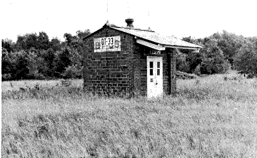
Figure 235. Building DT-33: Flammable Materials Storehouse.
