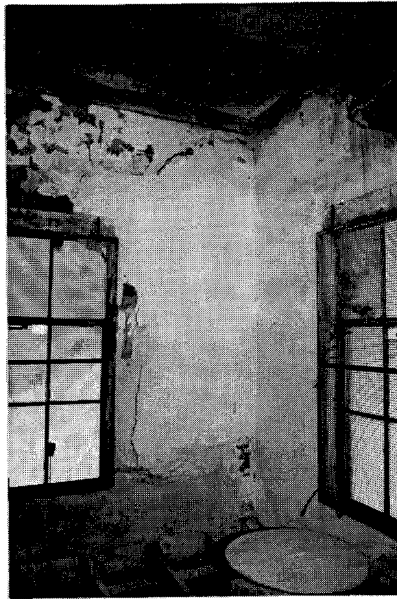
Figure 137. Building DT-11: Interior view of this Metal Parts Loading Building.
