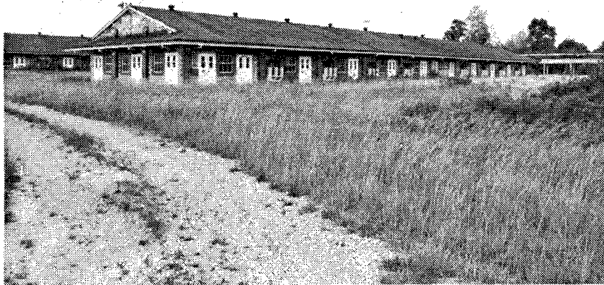
Figure 152. Building DT-22: Metal Parts Loading Building.
