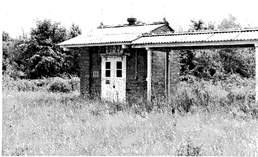
Figure 266. Building DT-27: Ready Magazine.
