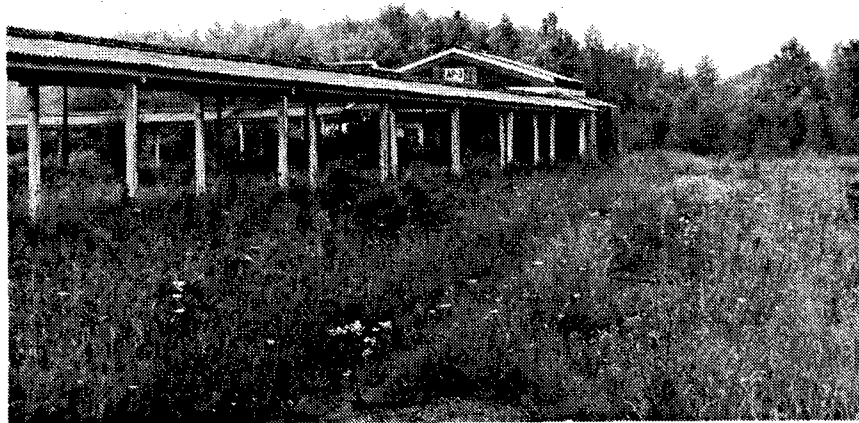
Figure 110. Building AP-3: Metal Parts Loading Building.
