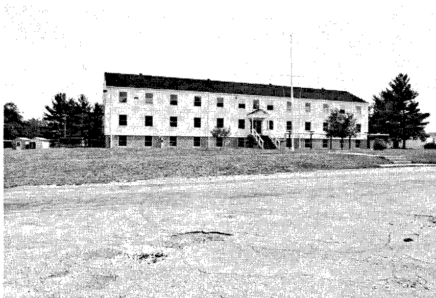
Figure 16. Building 1033: Dormitory and School Building.
