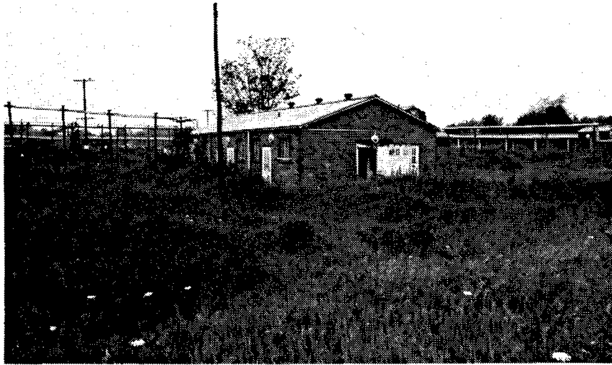
Figure 285. Building AP-13: Change House.
