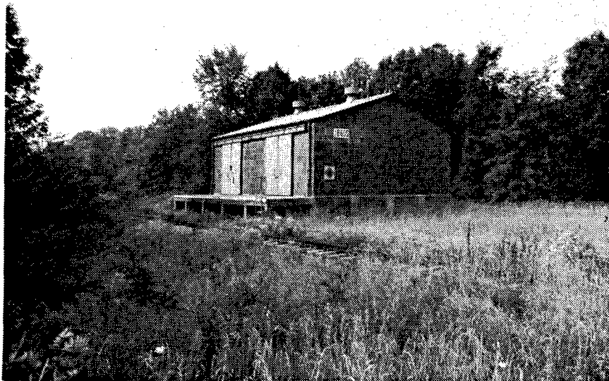
Figure 271. Building JB 605: General Purpose Magazine for fuze and booster storage.
