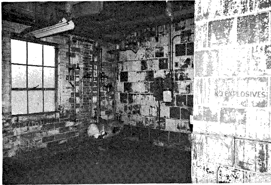
Figure 102. Building 2B-13: Interior view of this Tetryl Cupping Building.
