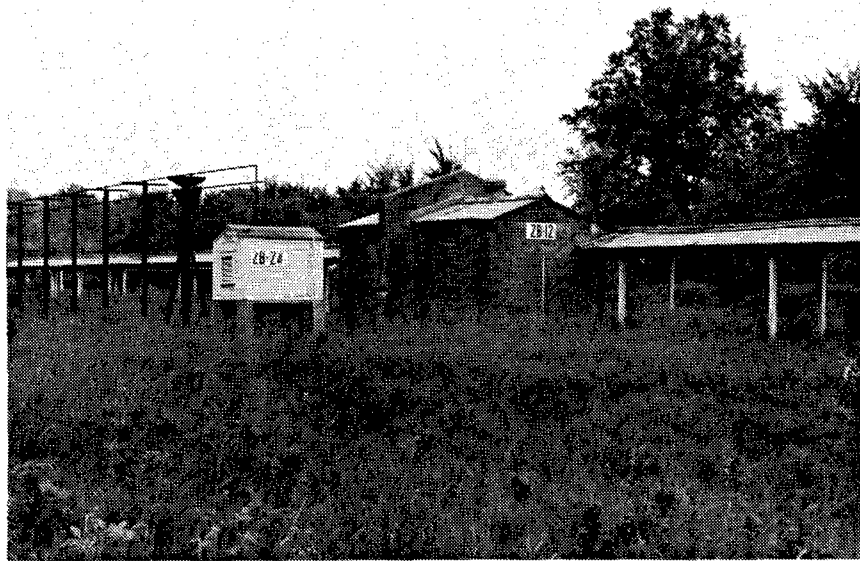
Figure 240. Building 2B-12 and Building 2B-24: Tetryl Pellet Storage Building and a Small Heater House, respectively.
