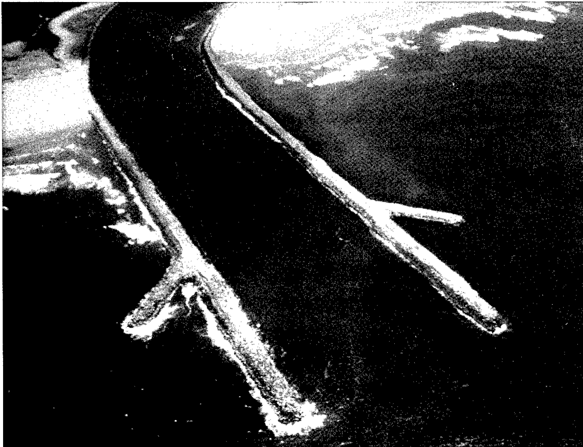
Figure 2. Jetties at Siuslaw River after 1985 extension
