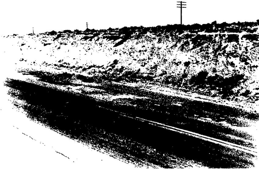
FIGURE 96.—*Highway Cut in a Portion of an Alluvial Fan (valley fill)*. Note the granular nature of the sediments. In this particular instance the cut exposed granular material on clay of a previous valley flow. The pavement rests on this clay (Nevada).
