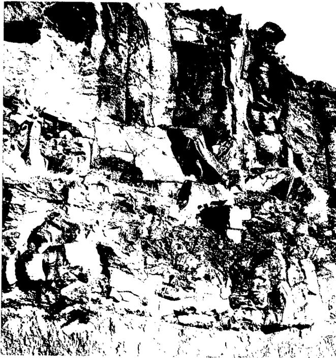
FIGURE 80. —*Highway Cut in a Layer of Basalt on an Inter-basalt Soil Layer (Washington).*
