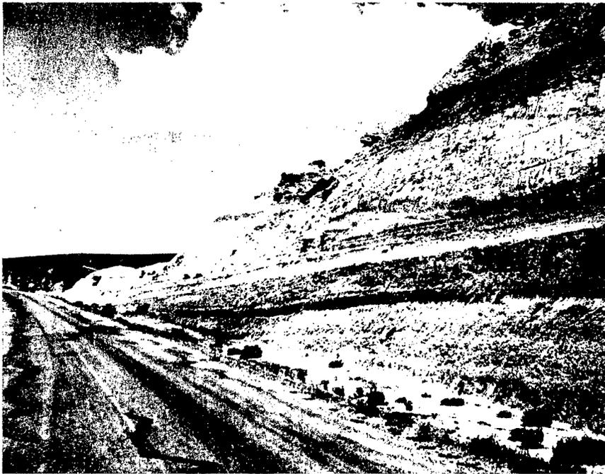
FIGURE 52.—*Highway Cut in Shale.* The numerous patches in the flexible pavement illustrate the engineering characteristics of this material. (See location 3 in fig. 49.)
