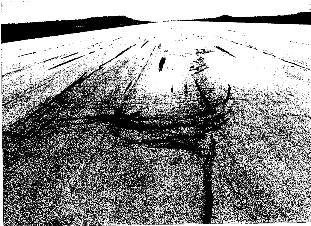
Photo C1. Close-up of slippage crack, Runway 15-33 (R1A)
