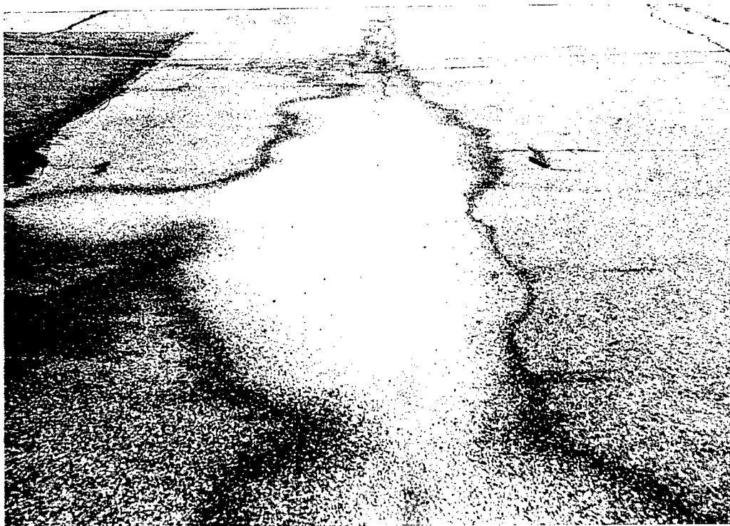
Photo C6. Medium-severity depression, South Ramp (A5B)
