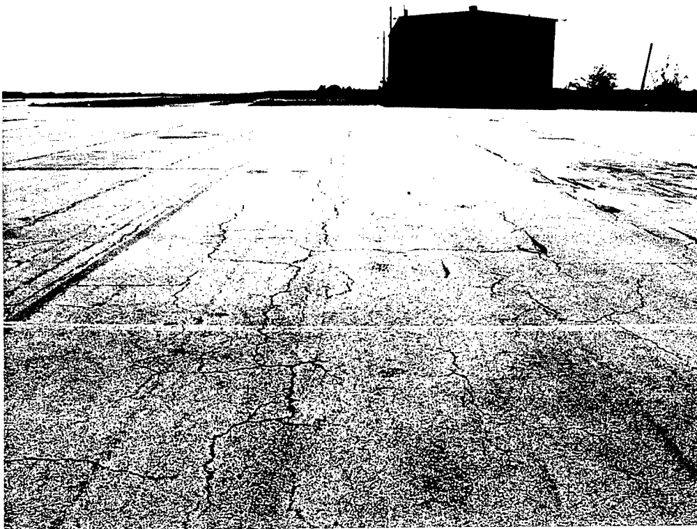
Photo C7. Block cracking, South Ramp (A6B)
