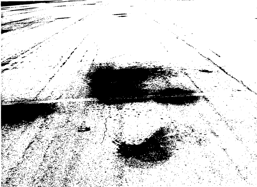
Photo C5. Typical oil spillage, South Ramp (A5B)
