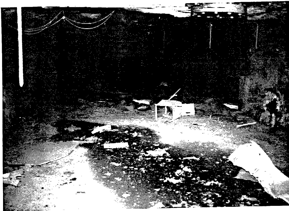
Figure 3-25. Another view of the damage 60 ft down E-drift from the 20-lb propylene oxide detonation.
