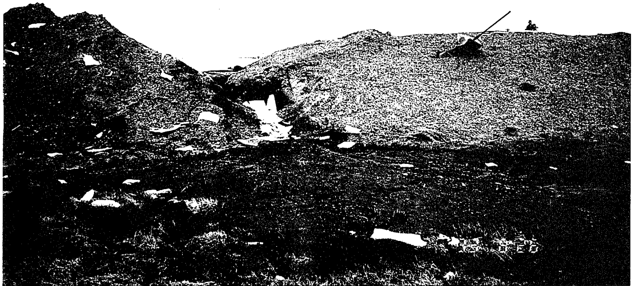
A view to the north of the inactive Beach Diesel Tanks (SS03) site. When the tanks were inactivated the lined berm was breached.
