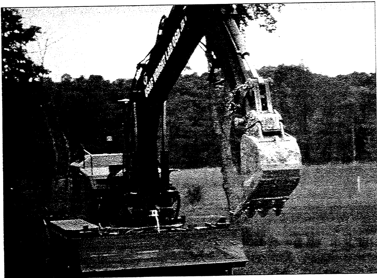
Figure 5.6.2-1 Wright Laboratory Remote Excavation Vehicle
