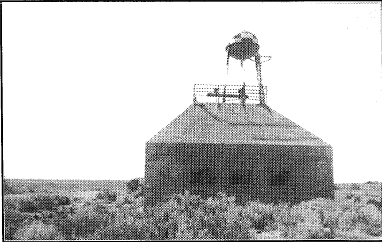
Figure 17. NATIV/JB-2 blockhouse, north elevation, with a later constructed water tower in background (Allred/Space Center 1994).
