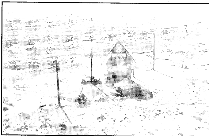
Figure 60. The Mart site Missile Theodolite tower, with covered cinetheodolite under open roof and evaporative coolers in front of the building, looking south, 26 November 1963 (Photo courtesy of WSMR Museum).
