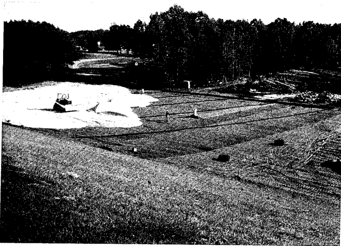
Photo 1 - Downstream Berm and Drainage System
