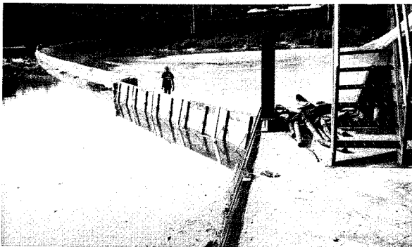
Photo #2 - Raising Water on 12 Meter (40 foot) test section, with temporary flashboards beyond
