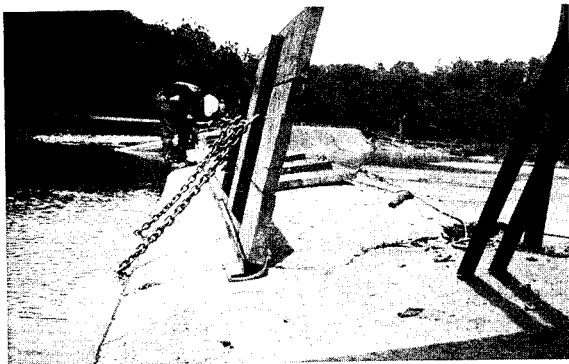
Photo #1 - Installation of Bottom Hinged Flashboard Panels
