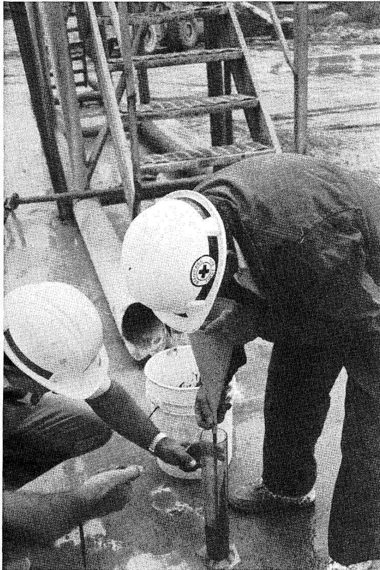
Figure 6. Measuring grout viscosity with Marsh flow cone
