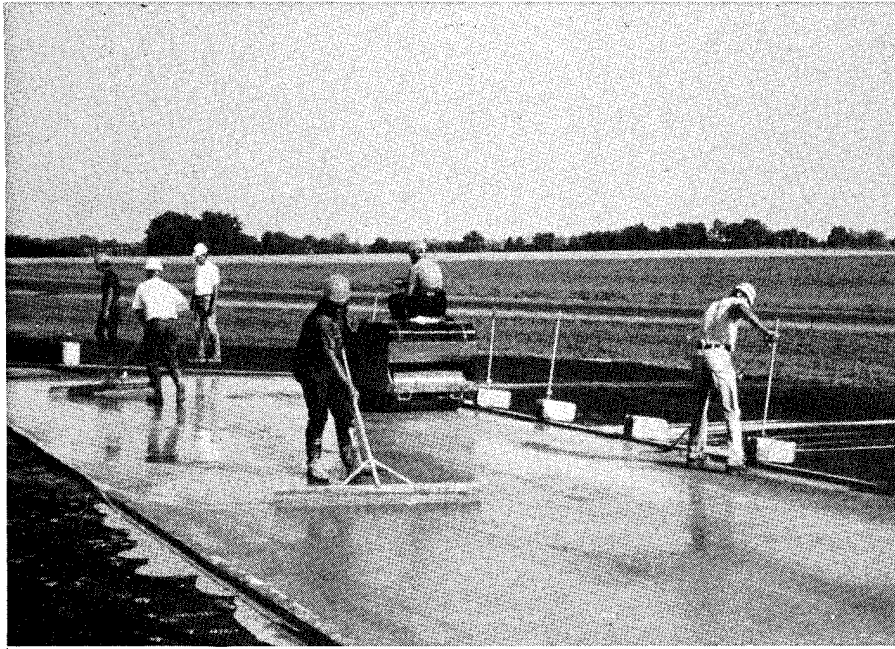
Figure 11. Removing excess grout from finished RMP surface
