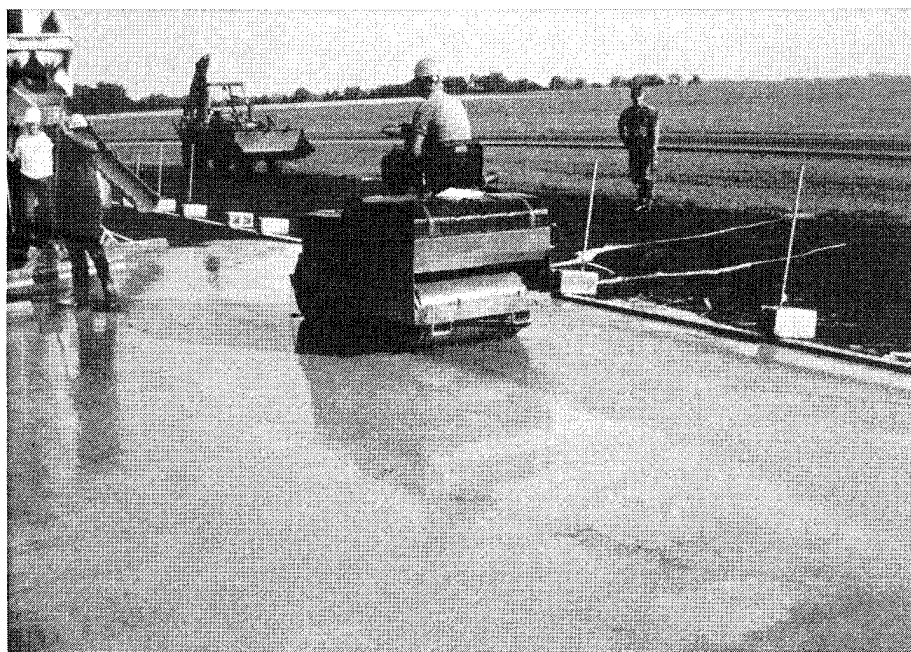
Figure 10. Small steel wheel roller vibrating grout into voids
