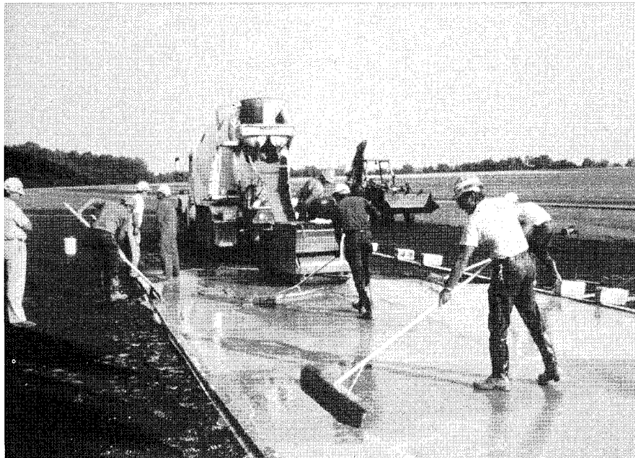
Figure 9. Squeegeeing excess grout over open-graded material
