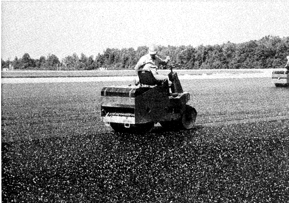
Figure 3. Rolling open-graded asphalt mixture with small roller
