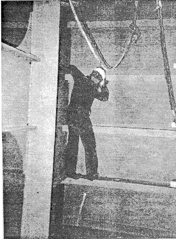
Inspector Climbing Side Longitudinals
