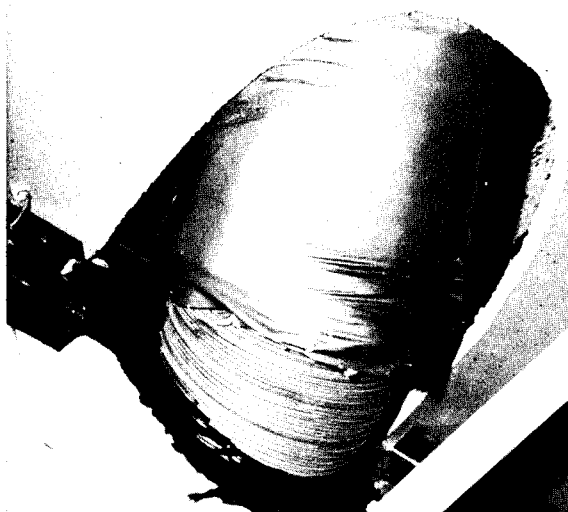
A fire-resistant ceiling is not effective if an architect or a workman allows wide holes for a pipe to pass through.
