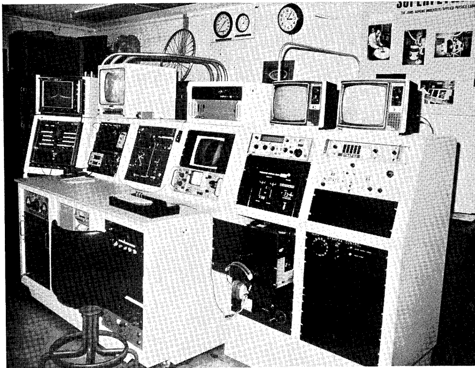
Fig. 5 New control console.
