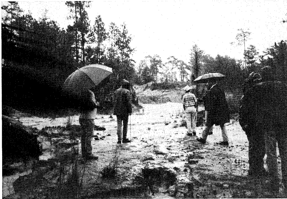
Figure 9. Shows the borrow pit, erosion channels draining the pit, and the failed berm which had been constructed across the pit outlet to the road to prevent runoff
