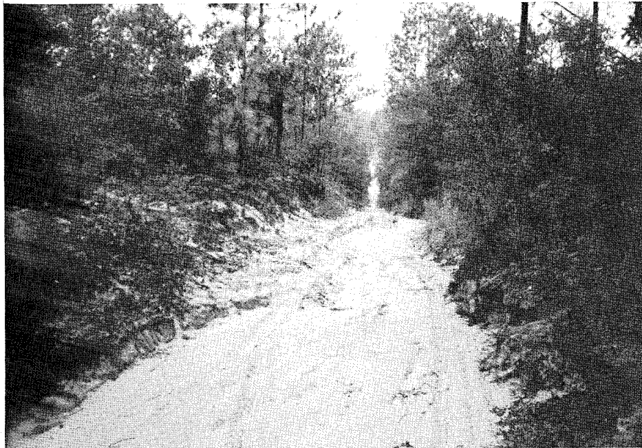
Figure 6. View looking west along Road 434 near Stop No. 1. This tertiary road is shown descending into the valley of a tributary of Juniper Creek. The road at this point serves as a channel funneling water from the relatively flat upland area into the valley and hence into the tributary
