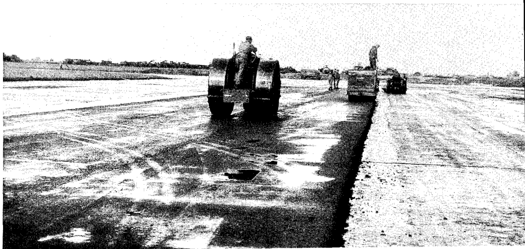
Workers roll the base course at RAF Fairford during runway rehabilitation authorized by the Ambassadors' Agreement. (below)
