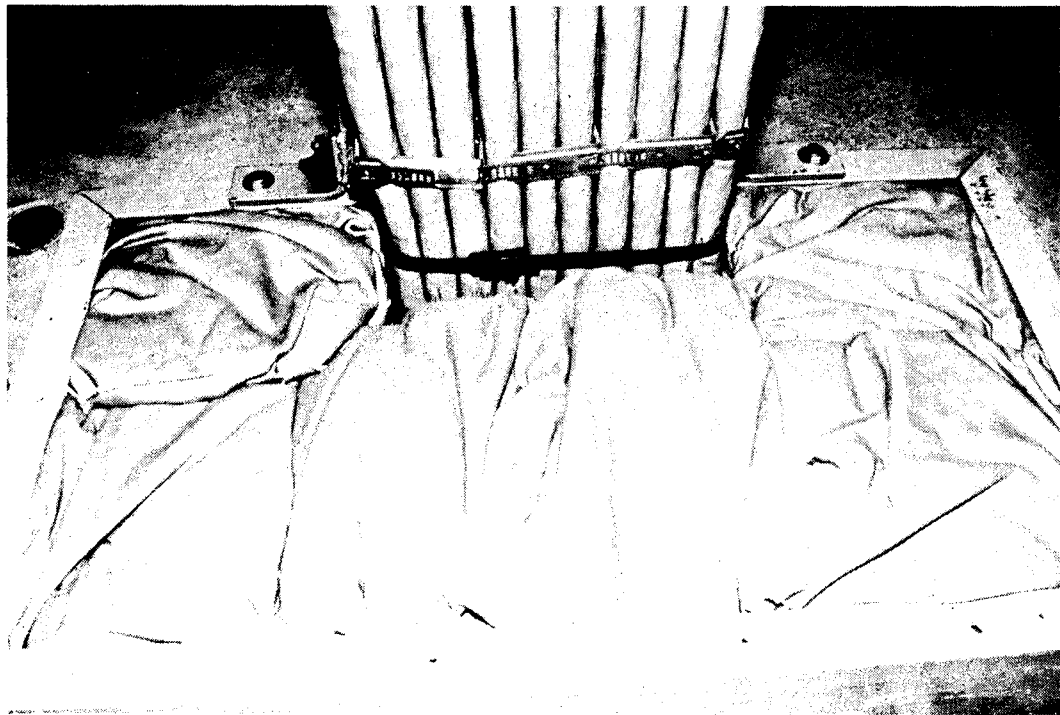
Figure 9. View of cable bundle in 1' x 2' vertis closure with mineral wool bags in place
