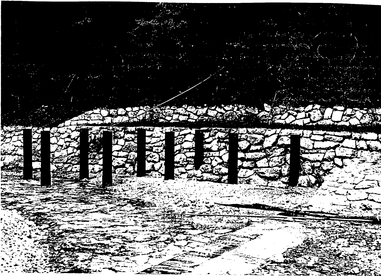
Plate 3 : Treibholzfang device on the river Lainbach. View downstream.
