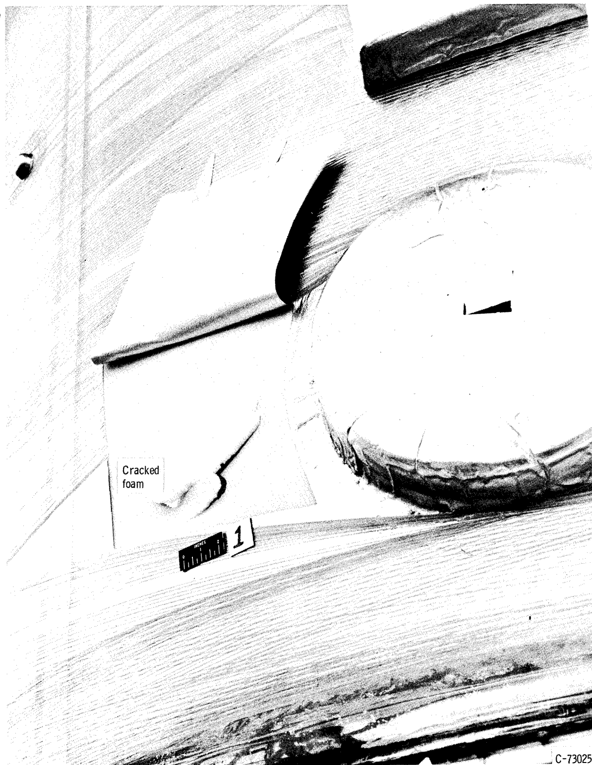
(b) MAM laminate folded back exposing cracked foam.
