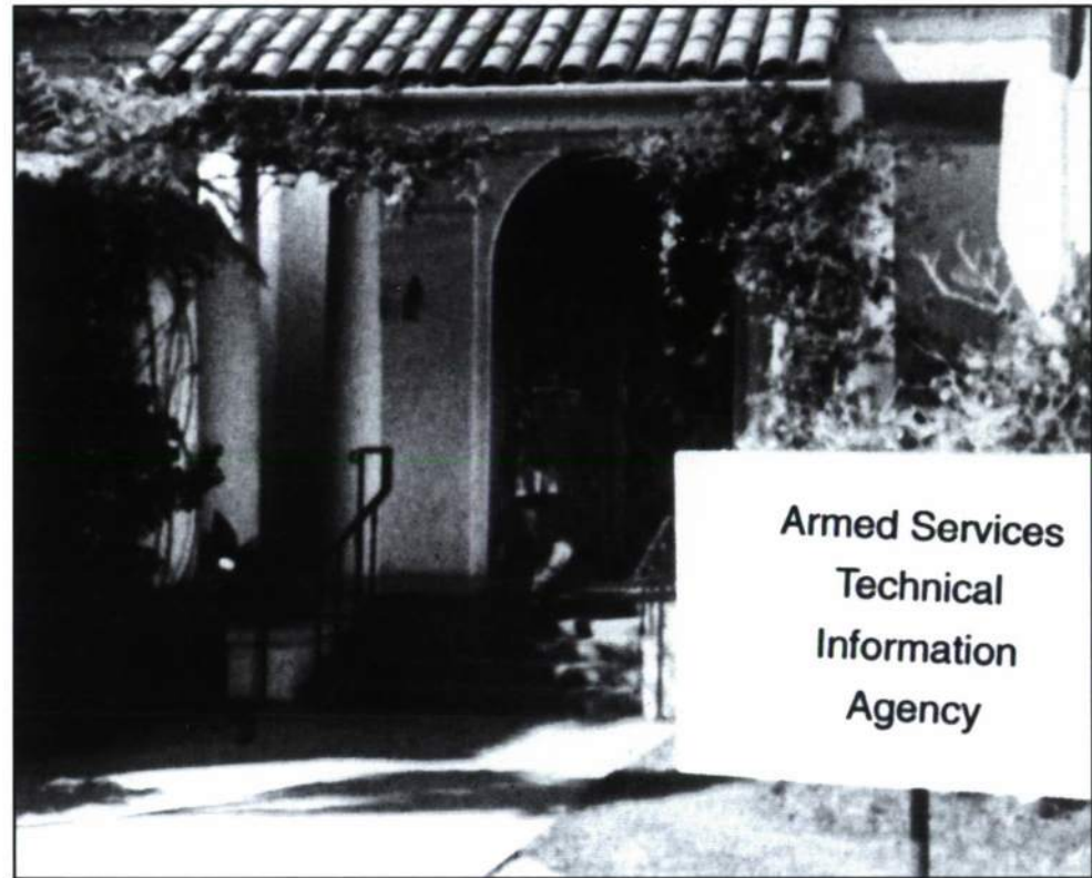
One of ASTIA's regional offices was located in this building in Pasadena, California.
