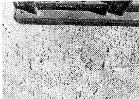
Fig. A.2.20.4b—Close-up scaling (very severe)
