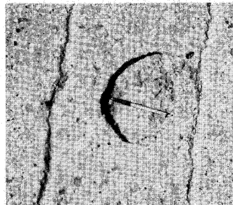
Fig. A.2.21.1—Small spall
