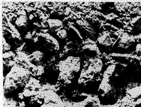
Fig. A.2.3—Cavitation damage
