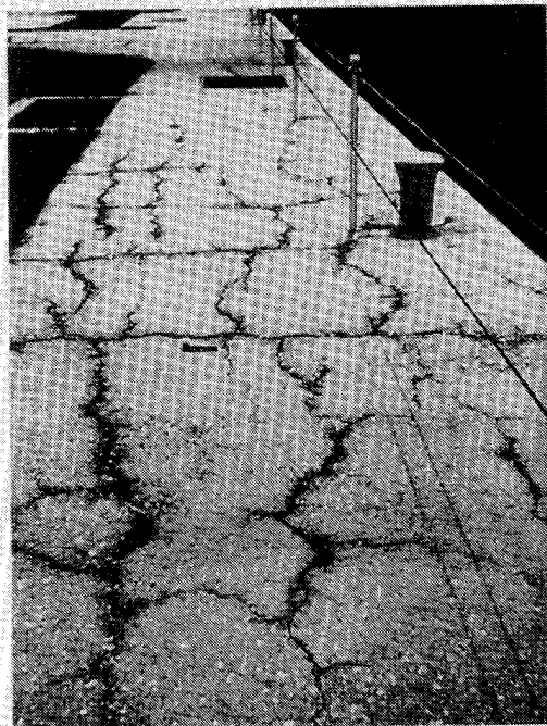
Fig. A.1.6d—Pattern cracking (alkali-silica reaction)
