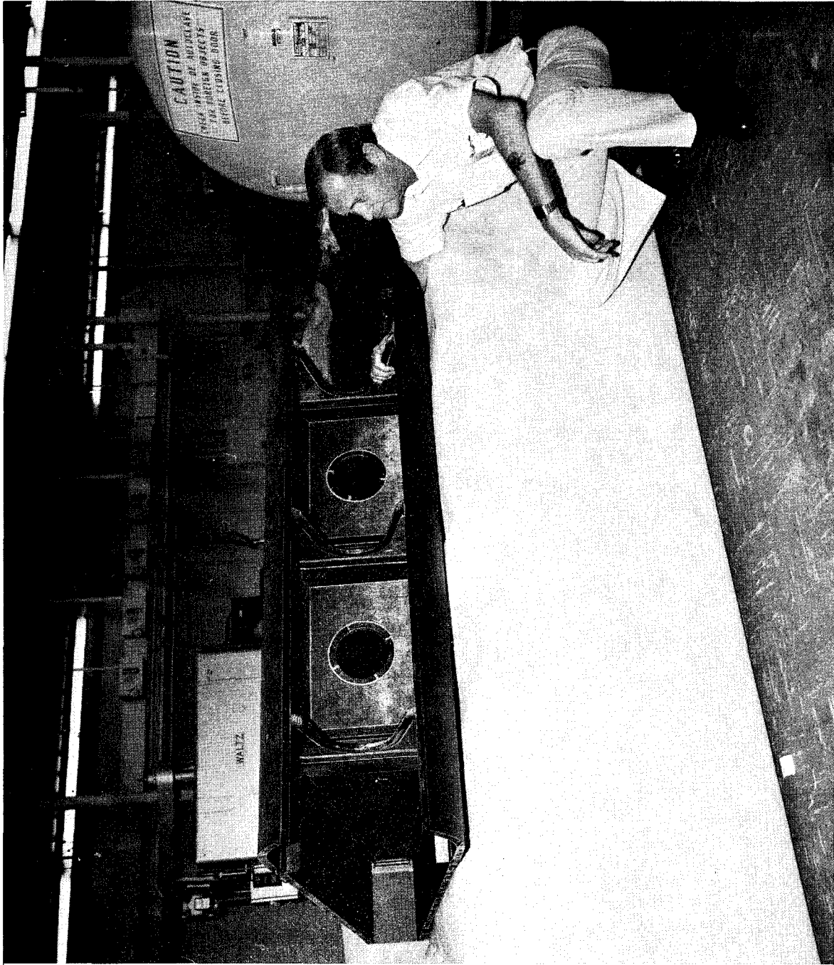
Figure 184. Completed Technology Demonstrator Segment Bonded Assembly
